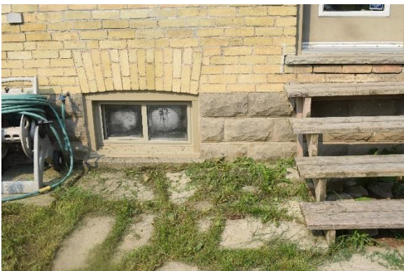
Plate 17: Looking west at foundation
