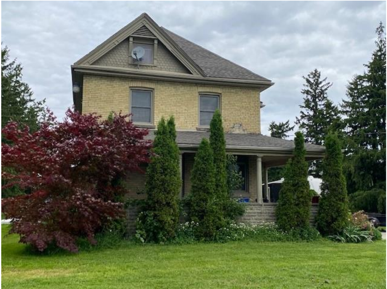
Image 3: Front, south elevation of house with hip roof and front facing gable with decorative bargeboard
