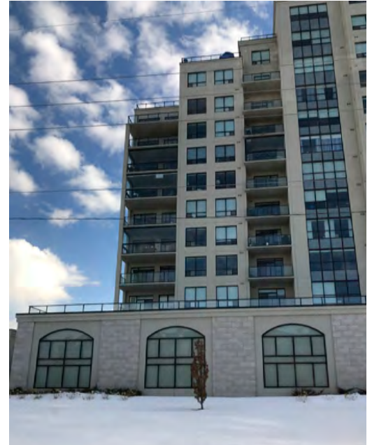
Above-Grade Parking Structure in Residential Development
