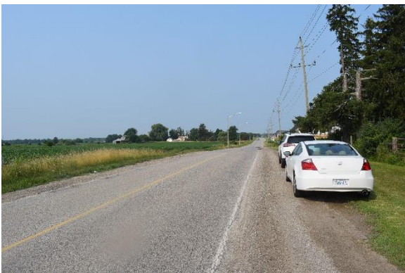
Plate 3: Looking west on Pack Road showing roadway, shoulders, and utility poles
