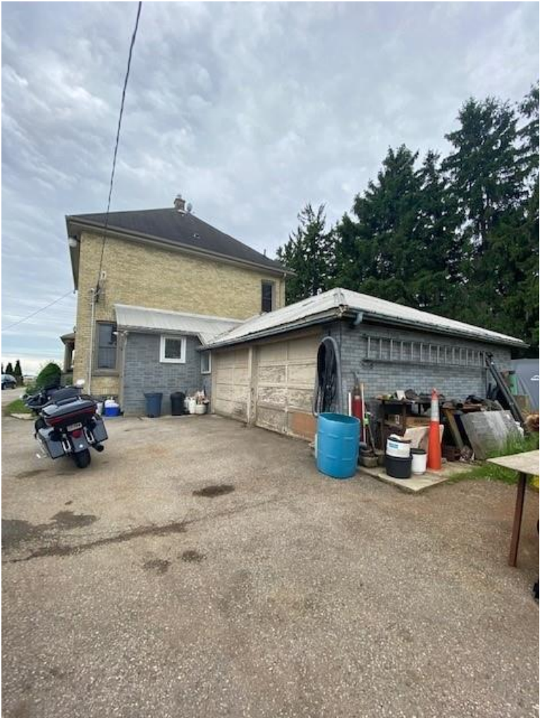
Image 6: Rear, north elevation of house on property showing contemporary garage additions and added rear entrance
