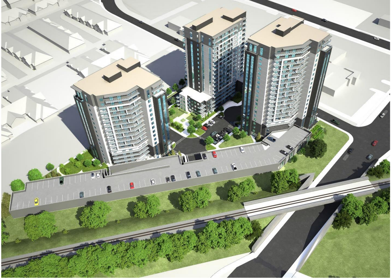
Figure 3: Bird's Eye view looking northeast (with CN Rail line in foreground and Building "A" on the left)
