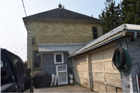
Plate 25: Additions, looking south
