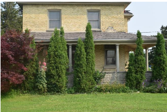
Plate 19: Looking north at first storey
