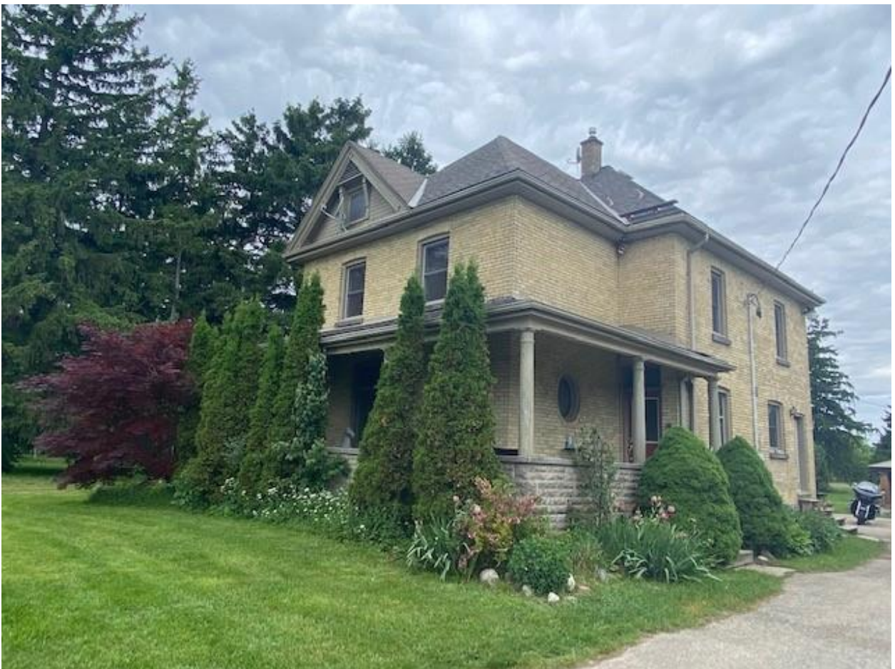
Image 2: South-east elevations of house on property showing wrap-around veranda and hip roof
