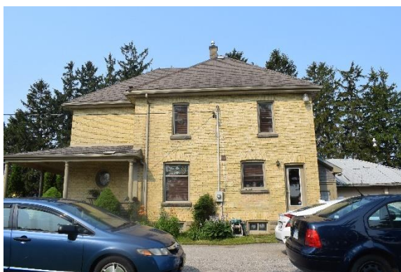
Plate 22: East elevation, looking west
