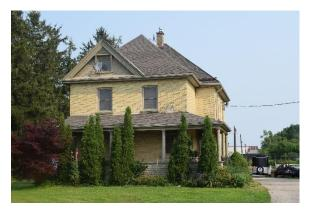
Plate 15: Looking north showing two and one half storey structure, hip roof, brick chimney, gable dormer, and projecting east bay
