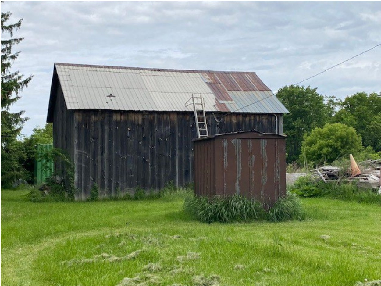
Image 16: Outbuildings at rear of property – metal shed, barn, and storage container
