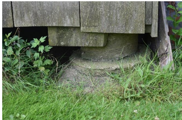
Plate 28: Concrete footing, looking south
