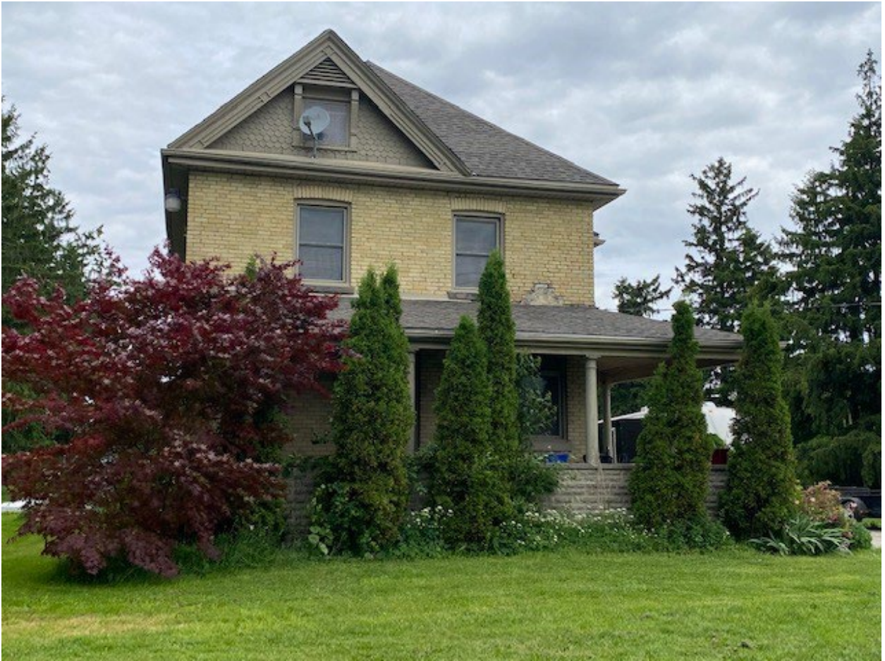
Image 3: Front, south elevation of house with hip roof and front facing gable with decorative bargeboard
