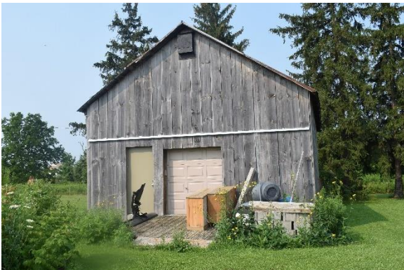
Plate 27: Gable roof outbuilding, east elevation looking west
