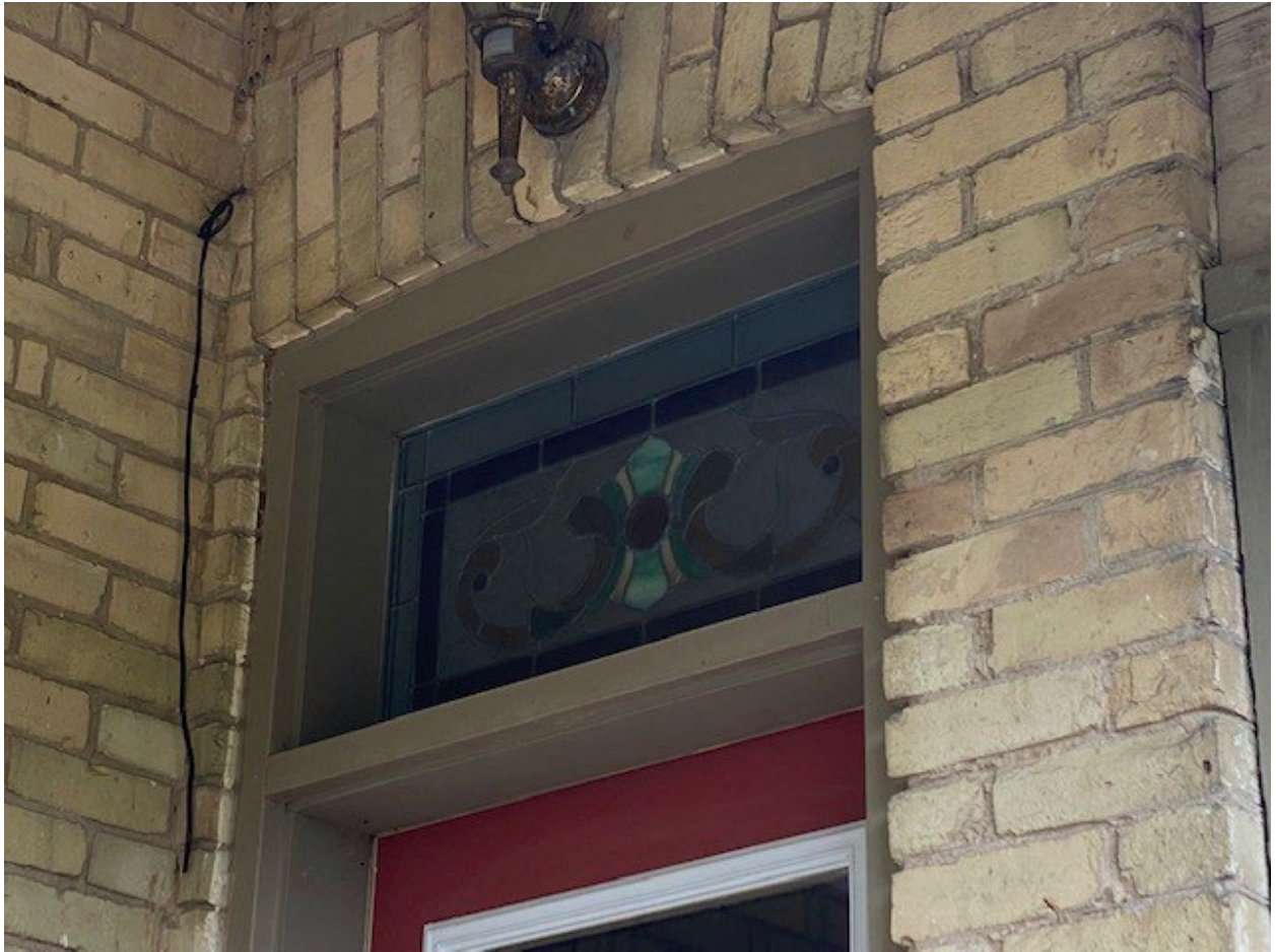
Image 11: Stained glass transom located above entrance door off veranda
