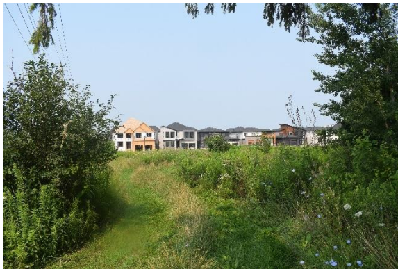
Plate 6: Looking west at new residential construction
