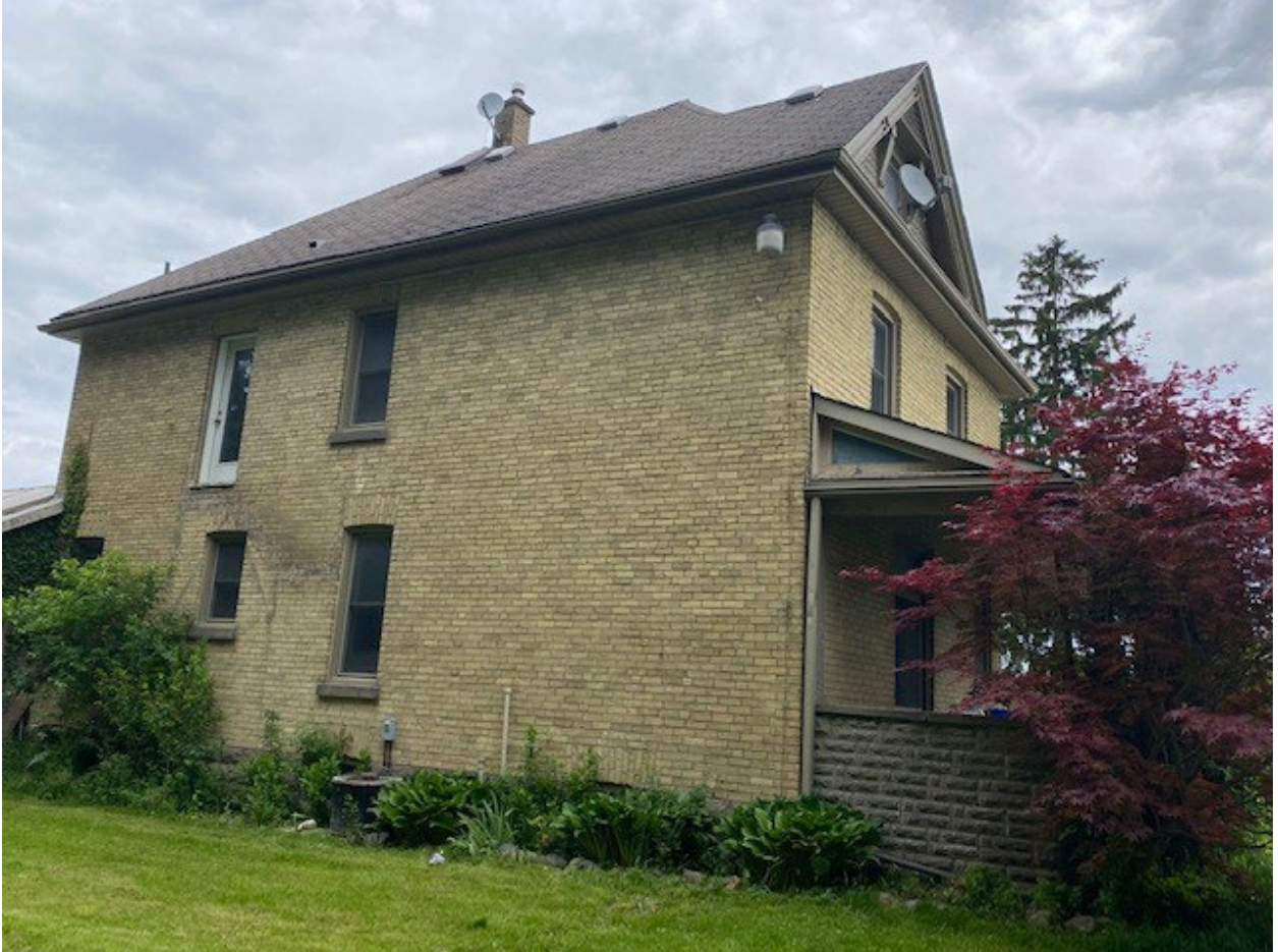
Image 4: West, side elevation of house on property
