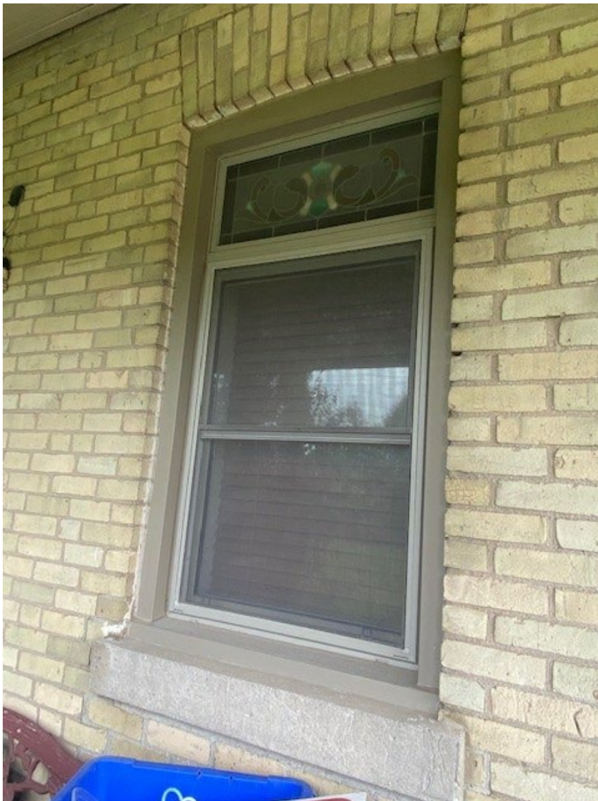
Image 12: Stained glass transom located above first storey window on south elevation
