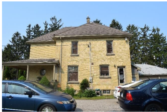
Plate 22: East elevation, looking west
