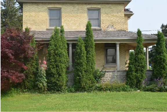
Plate 19: Looking north at first storey
