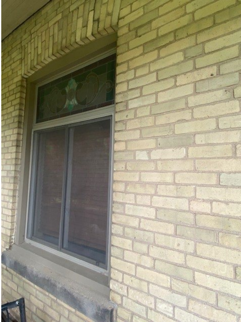
Image 13: Stained glass transom located above first storey window on south elevation
