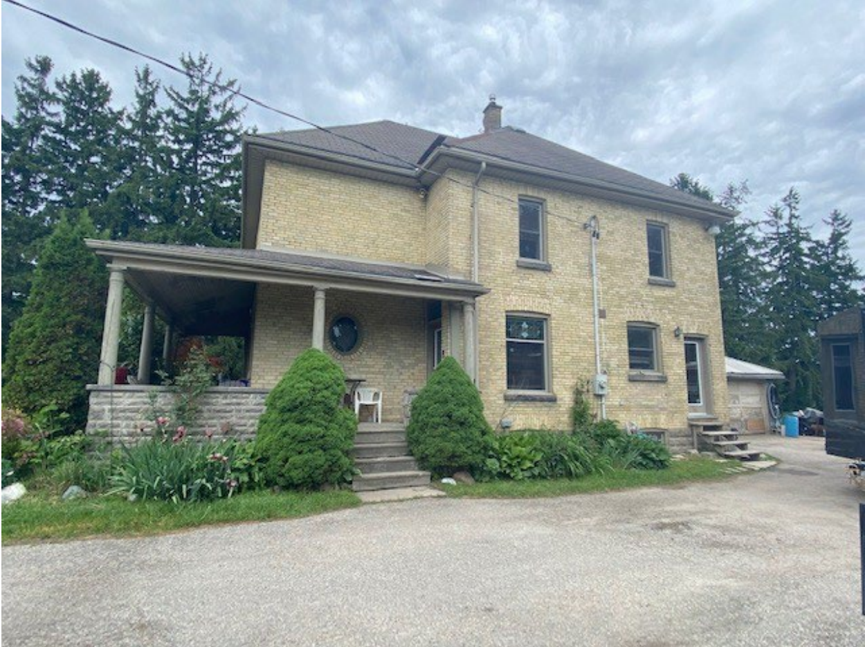
Image 8: East, side elevation of house on property showing wrap-around veranda
