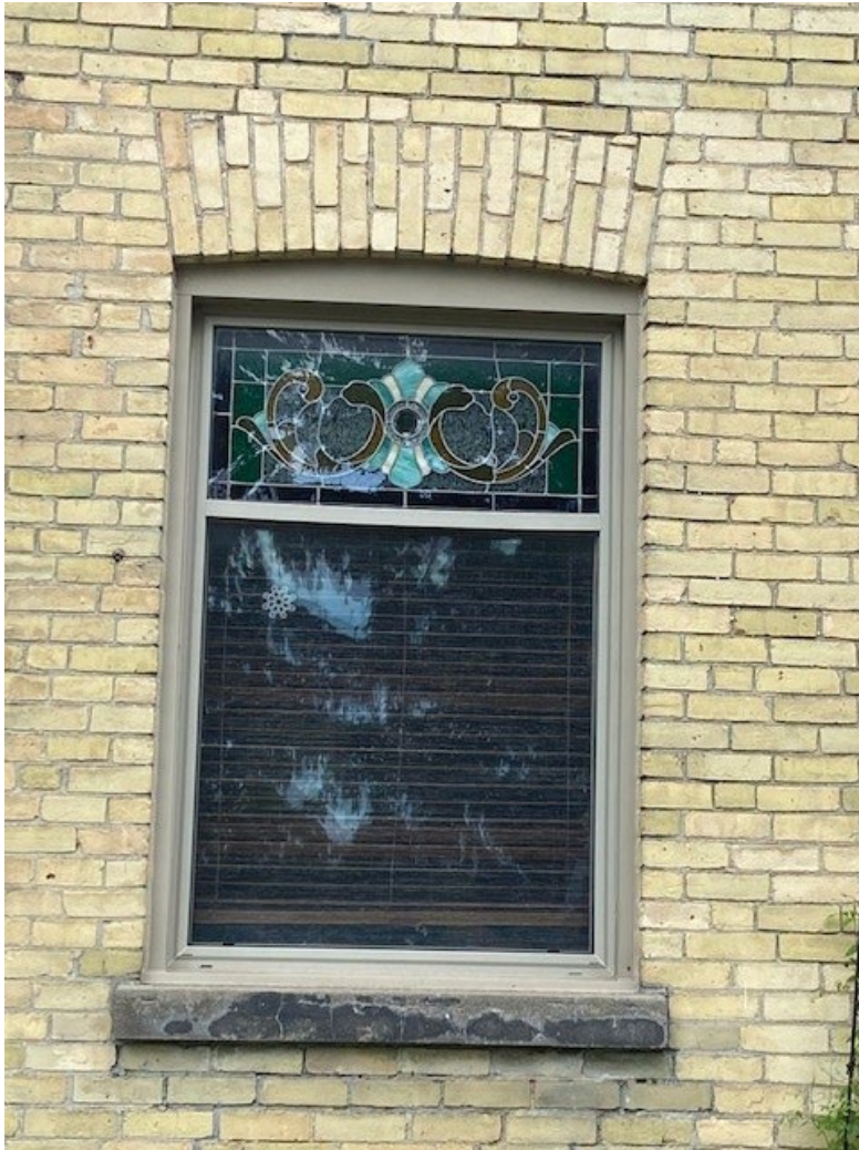
Image 9: Stained glass transom located above first storey window on east elevation
