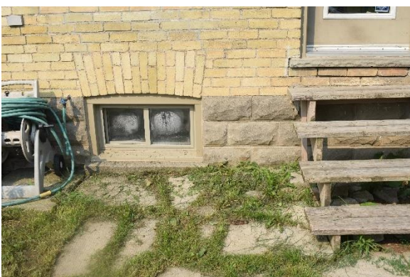
Plate 17: Looking west at foundation
