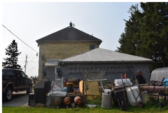
Plate 24: North elevation, looking south
