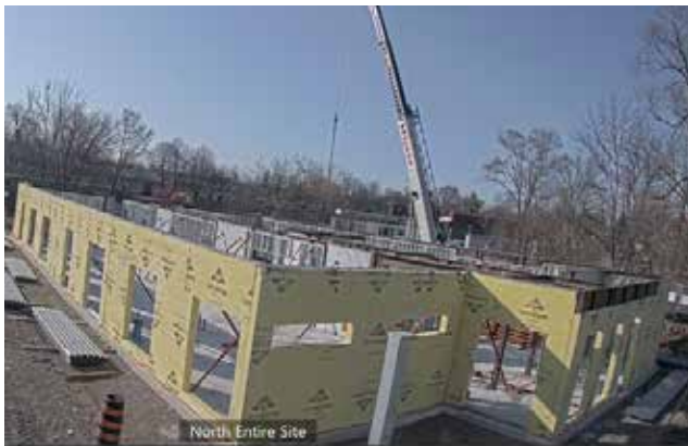
Thompson Road – Rapid Housing Initiative Project
