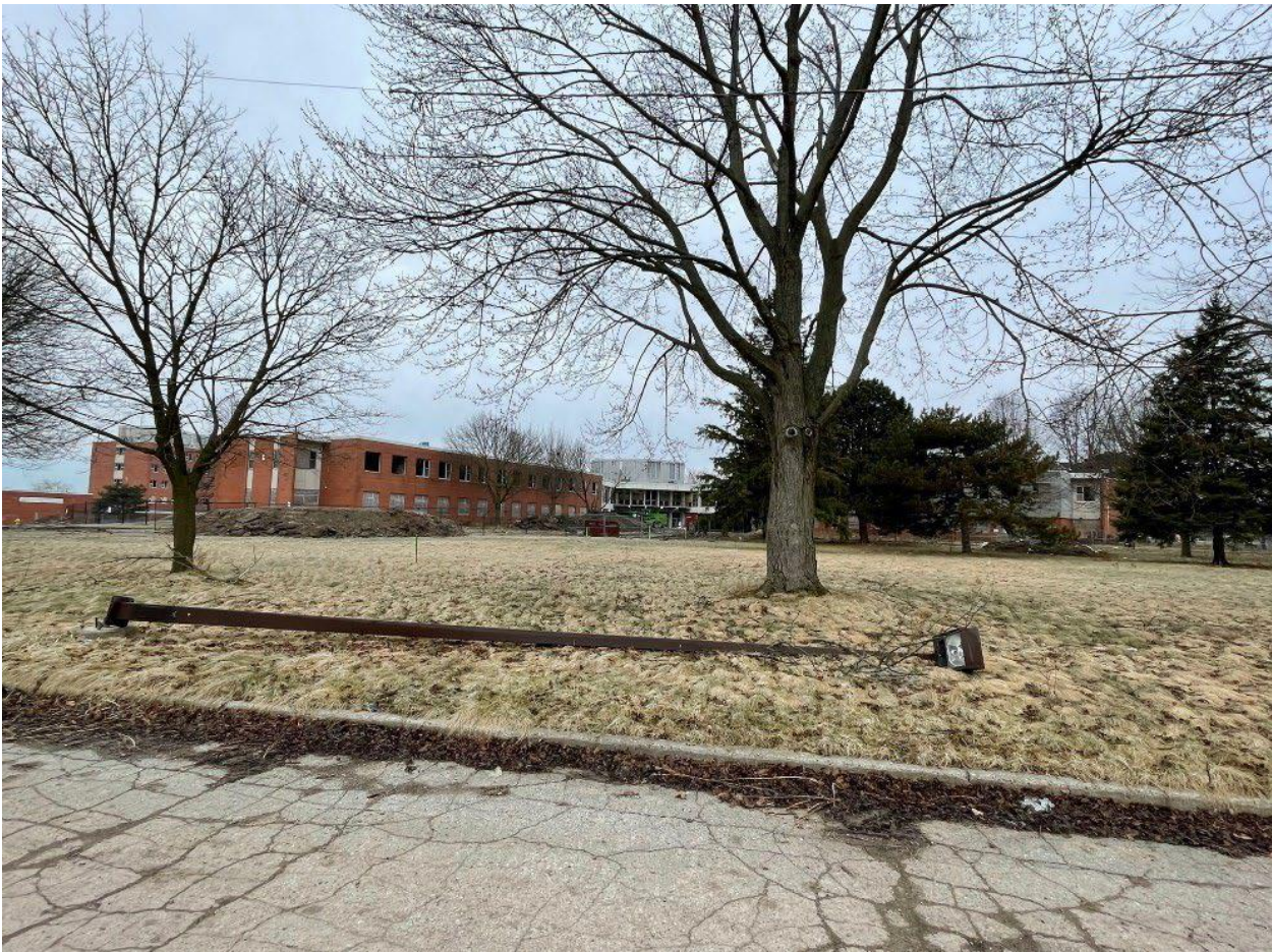
Figure 4. Building #1 (B12013) North Pavilion Building, facing east – L Dent, May 2022
