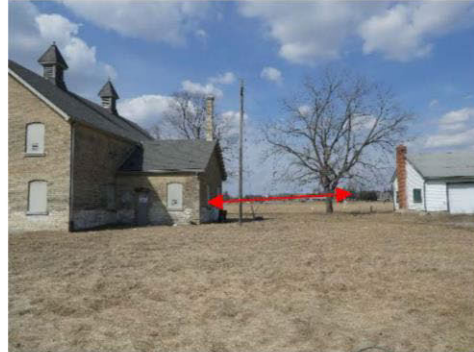
18m (60ft) to north structure demolition activity.
