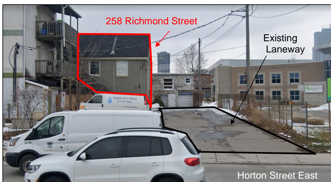
Figure 2: Photo of Subject Site and rear laneway (facing North on Horton Street East)
