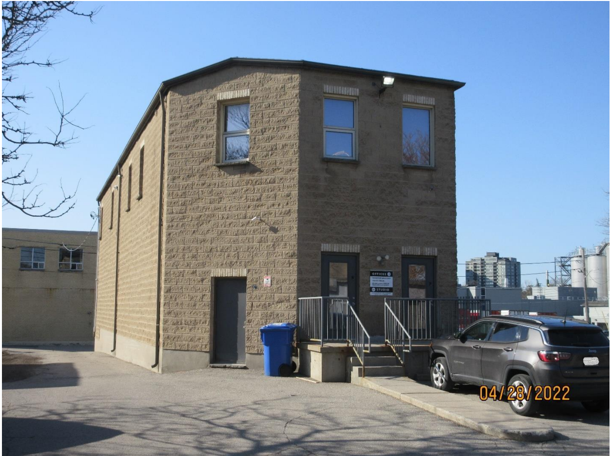
Image 3: View of the east and north (rear) façades of the property at 180 Simcoe Street.
