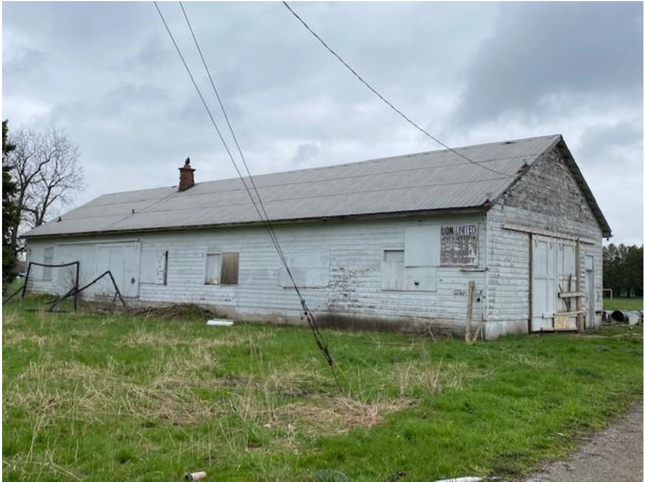
Figure 19. Building #5 (B16183) Soccer Shed, facing north-east – L Dent, May 2022
