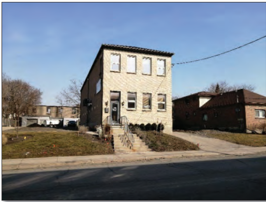
Figure 28: South elevation looking north-east from southside of Simcoe Street (MHBC, 2022).
