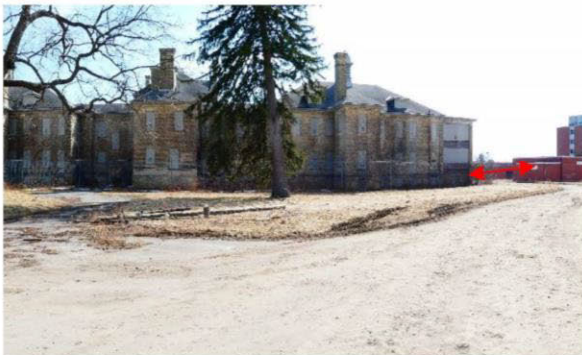
No structures on north, south or east elevations
