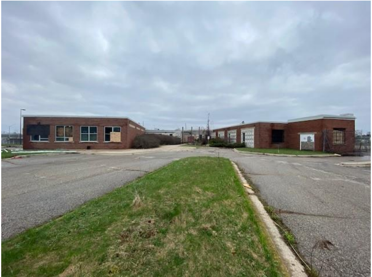
Figure 7. Building #2 (B12150) Ontario Government Building, facing west – L Dent, May 2022
