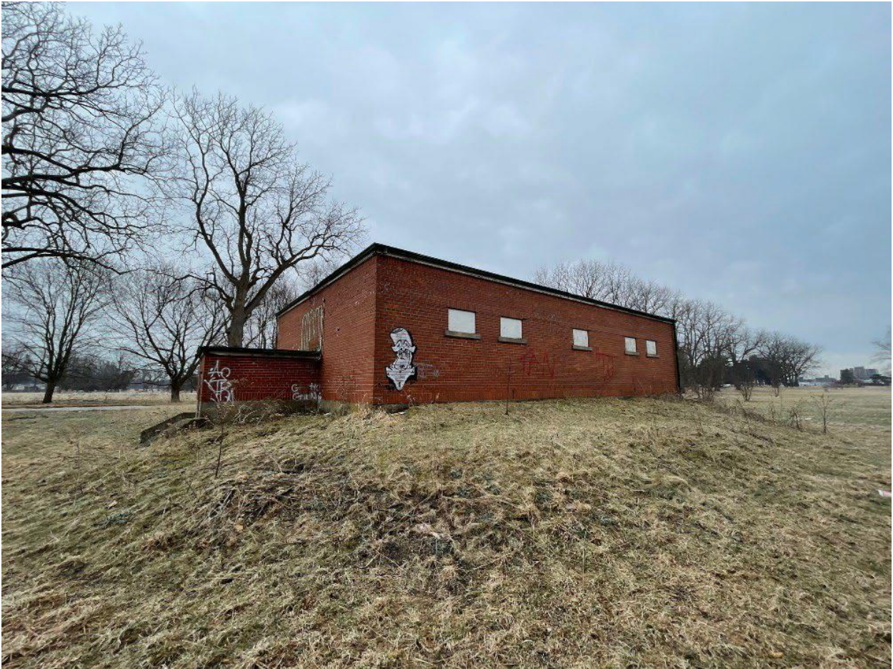
Figure 18. Building #4 (B12016) Granary, facing south-west – Zelinka, Mar 2022
