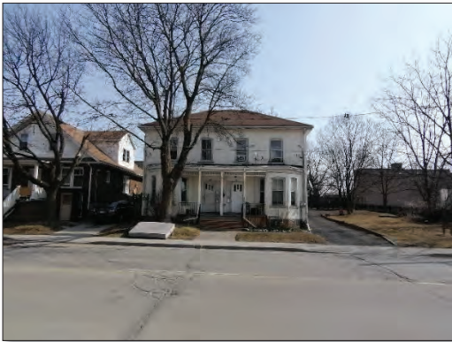
Figure 36: View of front façade (MHBC, 2022)
