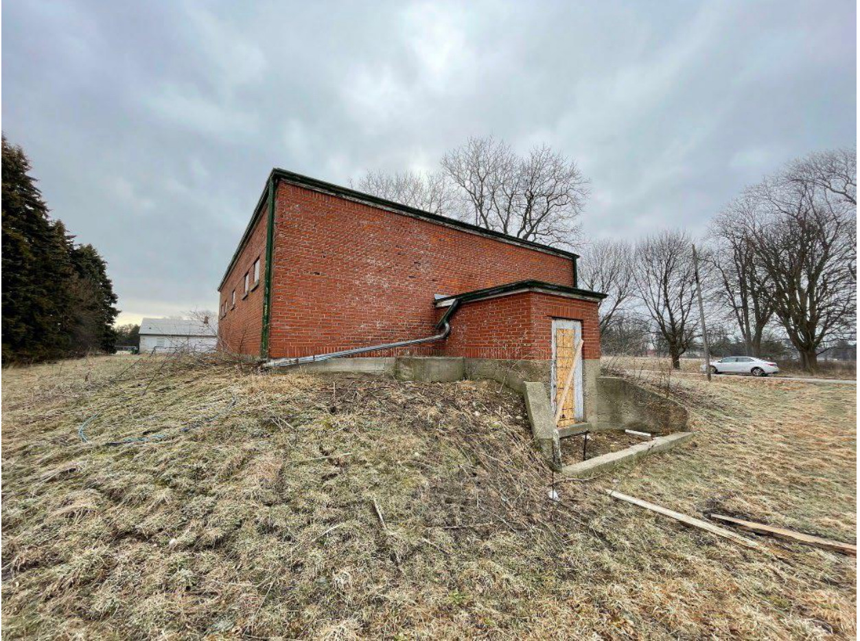
Figure 16. Building #4 (B12016) Granary, facing east – Zelinka, Mar 2022
