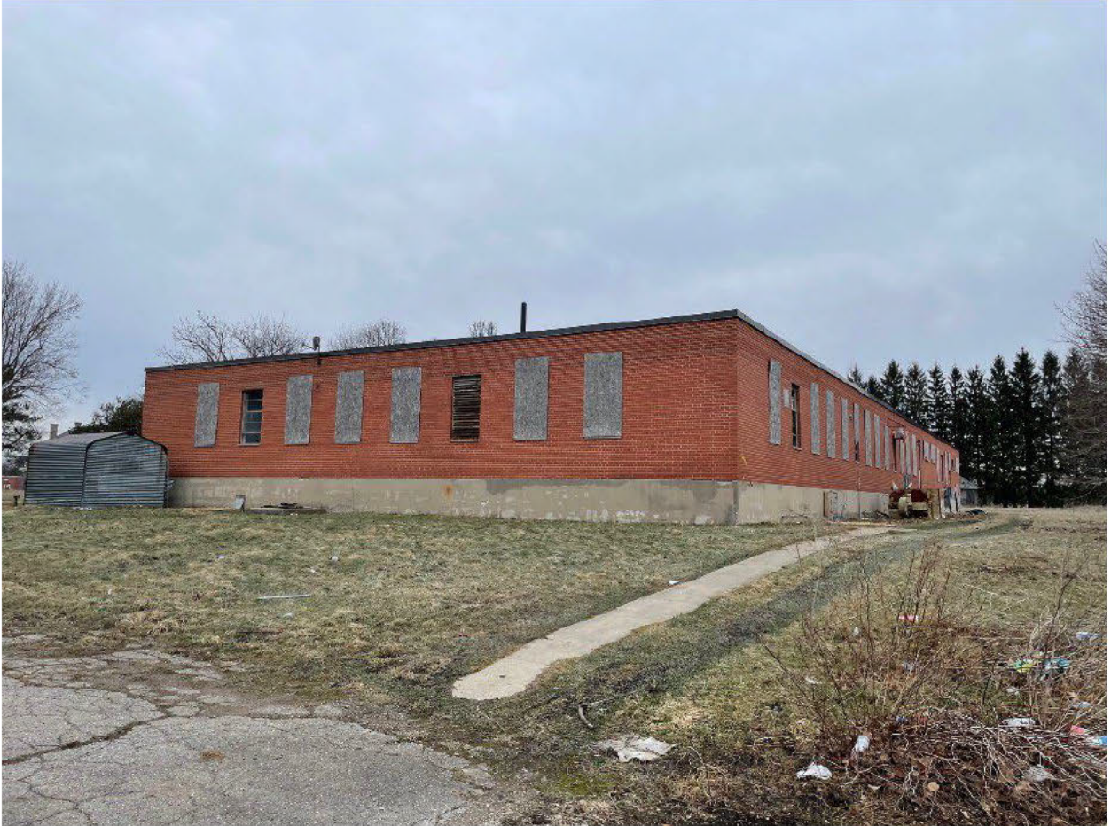
Figure 26. Building #7 (B12033) Laundry Building, facing north – Zelinka, Mar 2022
