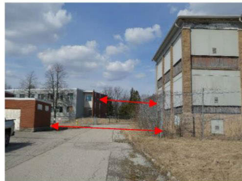
18m (60ft) to west structure demolition activity. And 37m(120ft) to north/west structure demolition activity.
