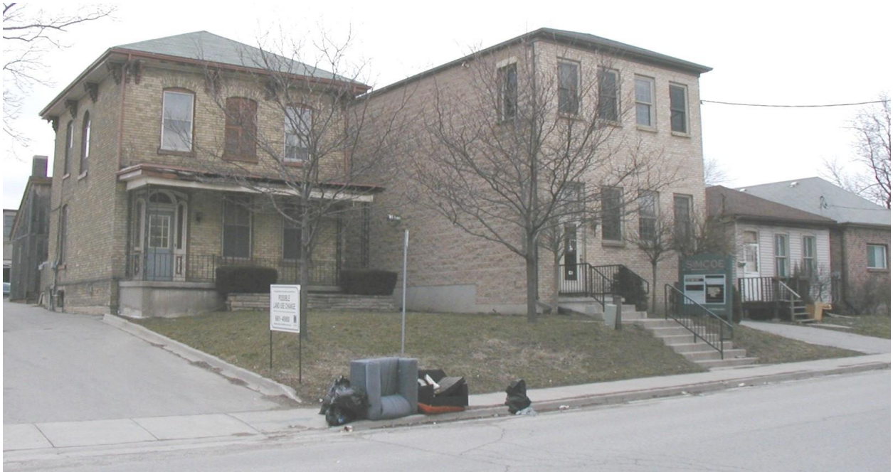
Image 5: View of the properties at 178 Simcoe Street (left), 180 Simcoe Street, and 182 Simcoe Street in 2002. The buildings on 178 Simcoe Street and 182 Simcoe Street were demolished in 2002.
