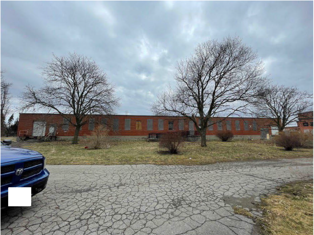
Figure 25. Building #7 (B12033) Laundry Building, facing east – Zelinka, Mar 2022
