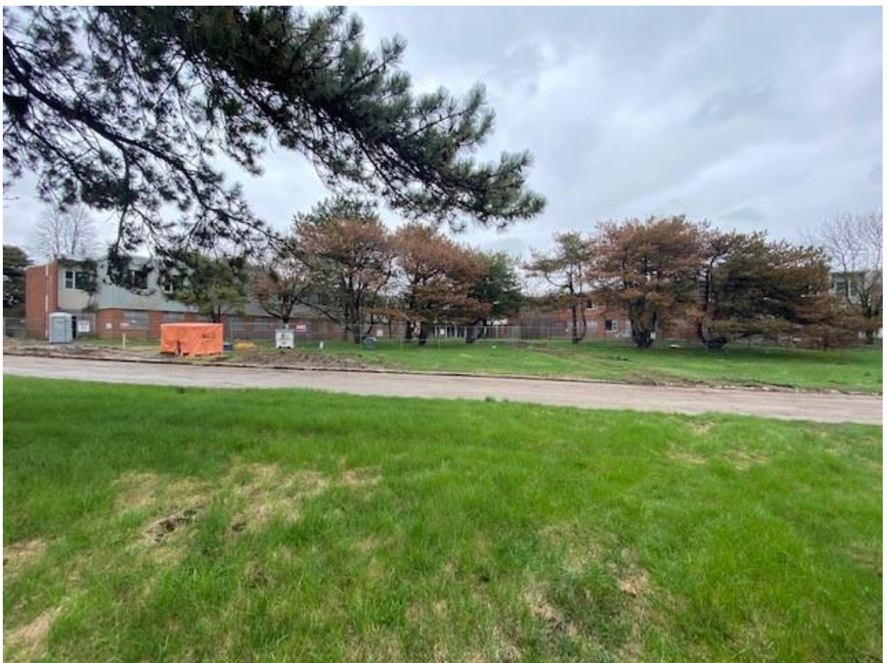
Figure 2. Building #1 (B12013) North Pavilion Building, facing east – L Dent, May 2022
