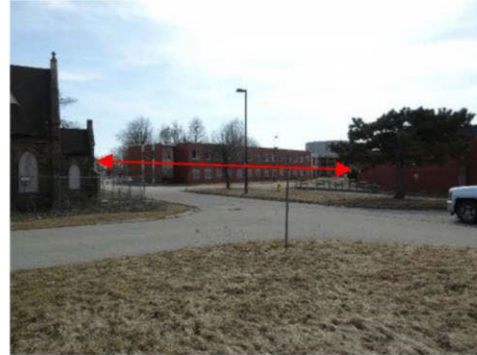
30m (98ft) to west structure demolition activity.
