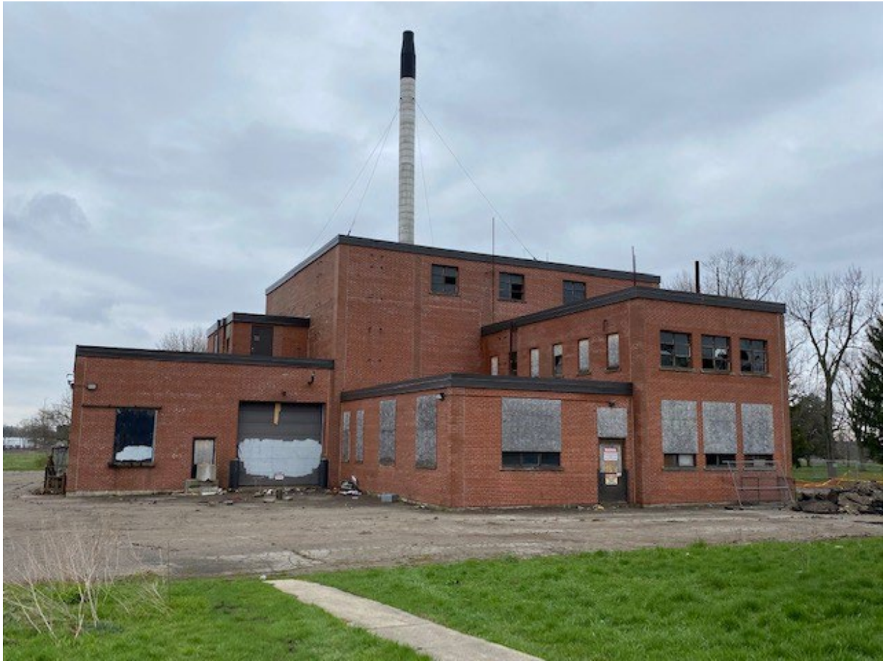
Figure 27. Building #8 (B12034) Powerhouse, facing south – L Dent, May 2022
