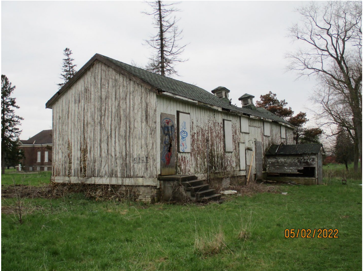
Figure 21. Building #6 (B17057) Potting Shed, facing south-west – M. Greguol, May 2022
