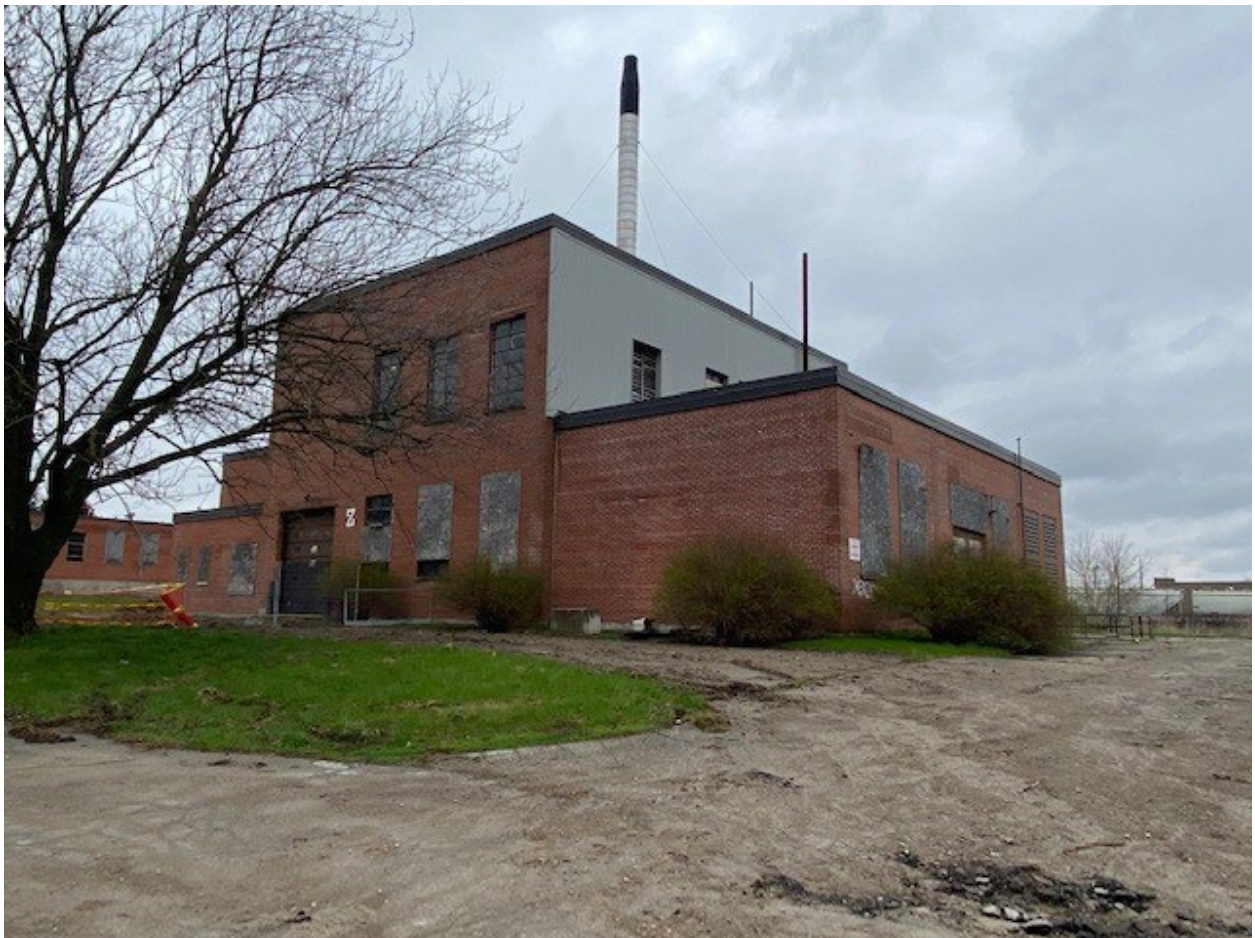
Figure 28. Building #8 (B12034) Powerhouse, facing north-east – L Dent, May 2022
