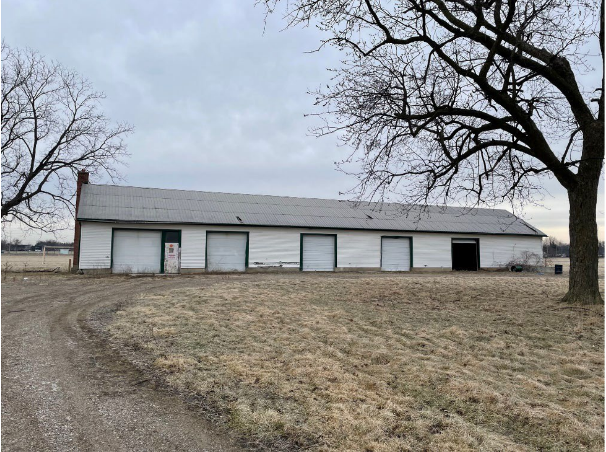
Figure 11. Building #3 (B16182) Tractor Barn, facing north – Zelinka, Mar 2022
