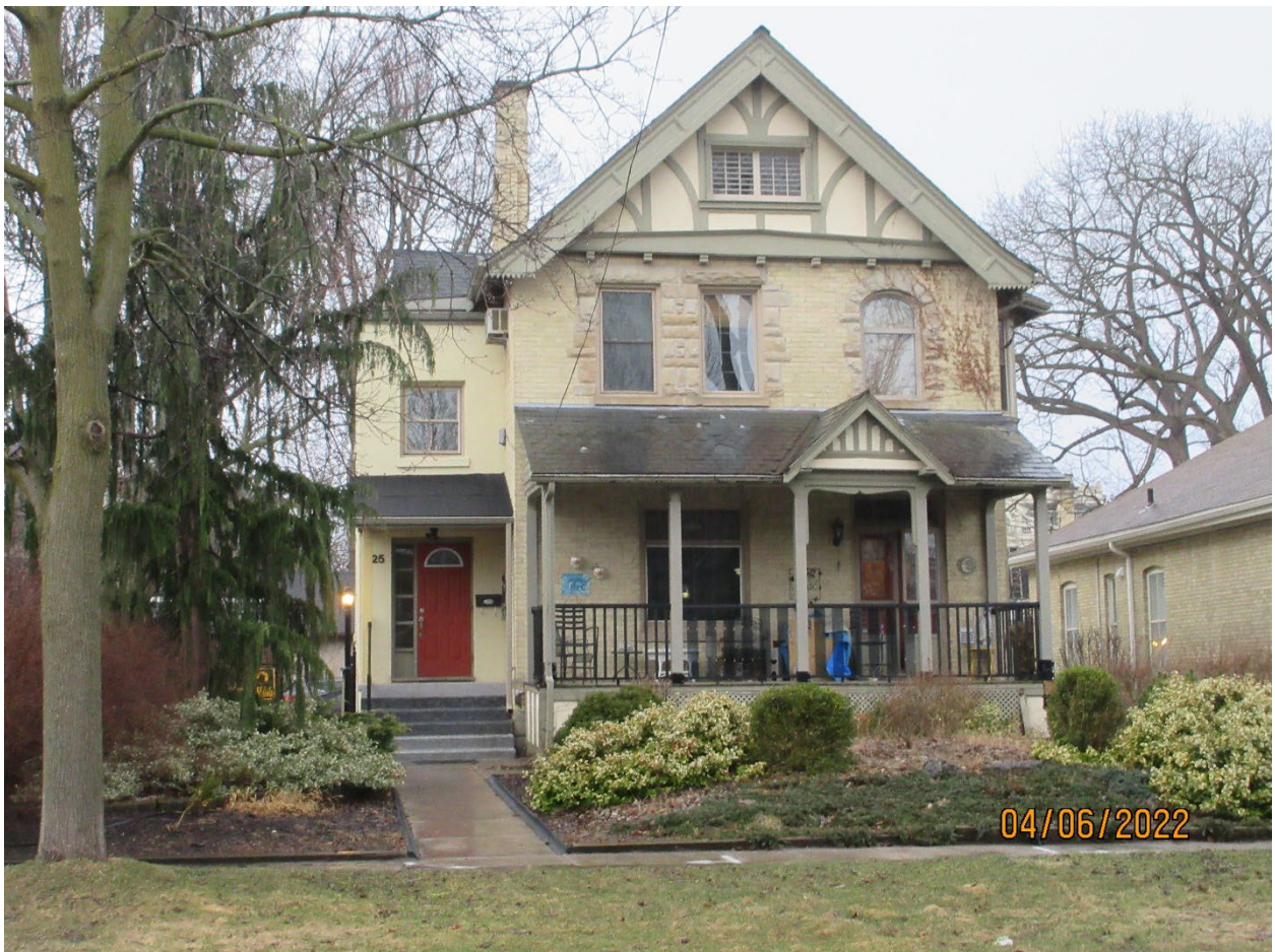
Image 3: Photograph of the property at 525 Dufferin Avenue, on April 6, 2022, showing the changes completed to the railing/guard of the porch.
