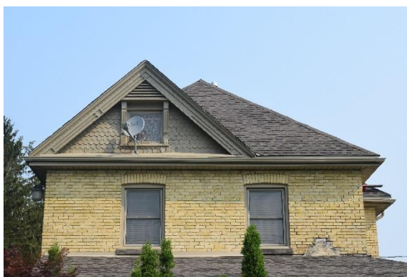
Plate 18: Looking north at gable dormer and second storey windows
