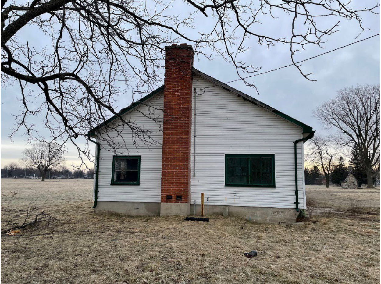
Figure 12. Building #3 (B16182) Tractor Barn, facing east – Zelinka, Mar 2022
