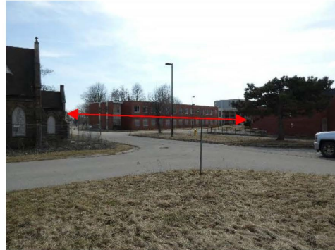
30m (98ft) to west structure demolition activity.
