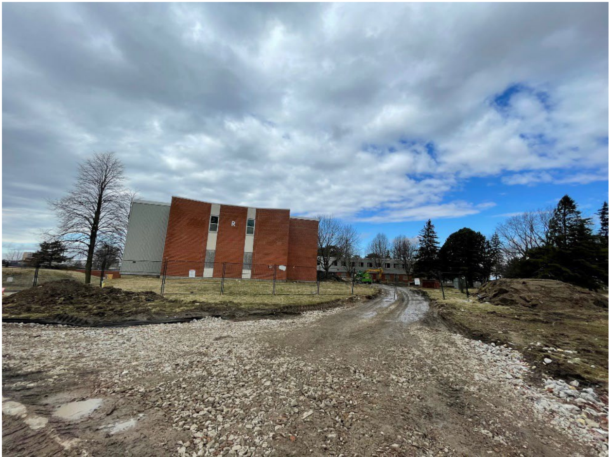
Figure 1. Building #1 (B12013) North Pavilion Building, facing east – Zelinka, Mar 2022
