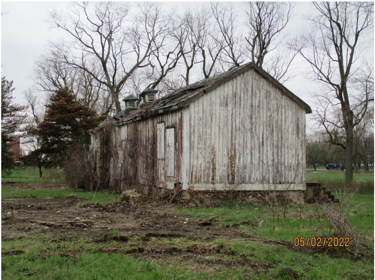
Figure 24. Building #6 (B17057) Potting Shed, facing north-east – M. Greguol, May 2022
