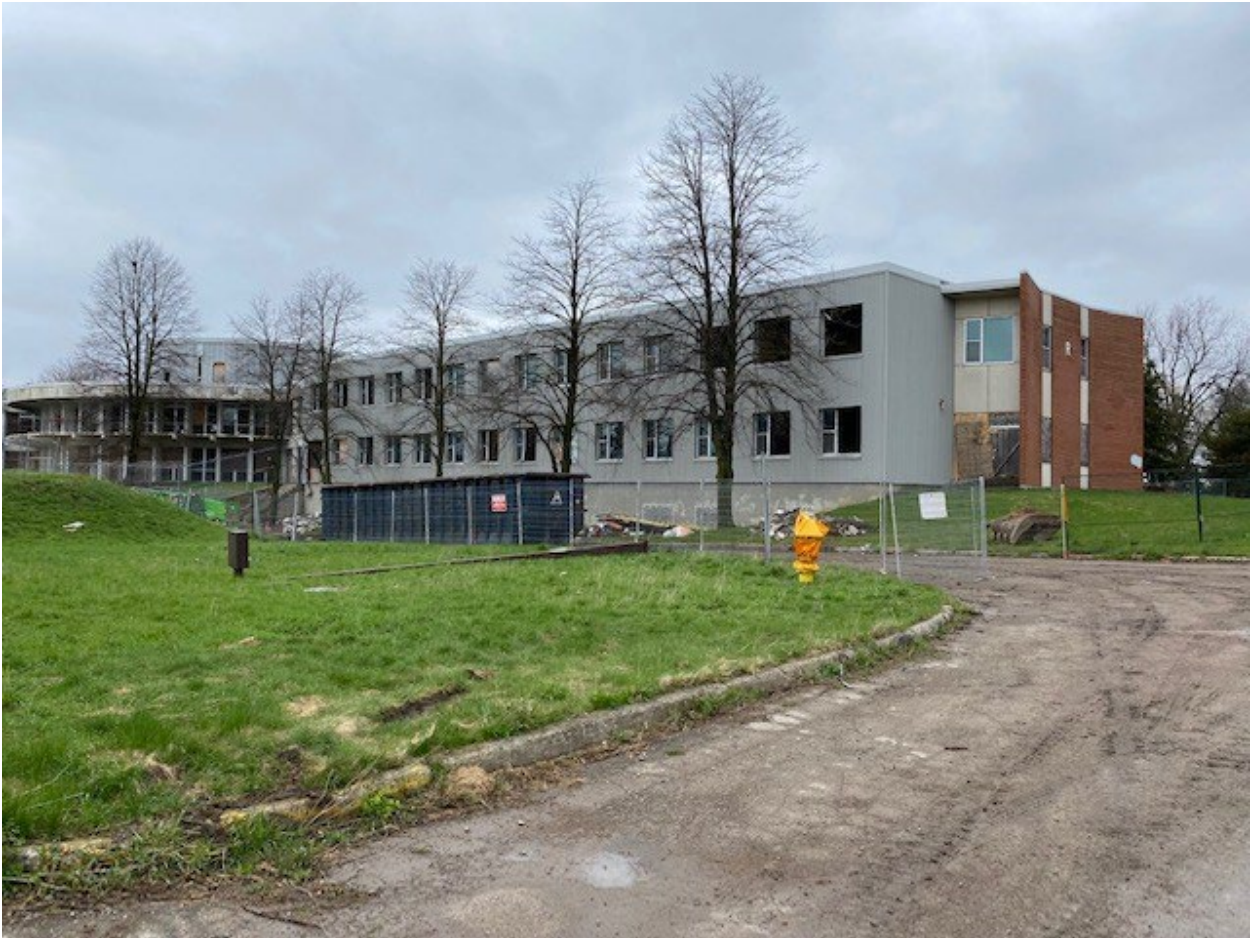
Figure 6. Building #1 (B12013) North Pavilion Building, facing north-west – L Dent, May 2022
