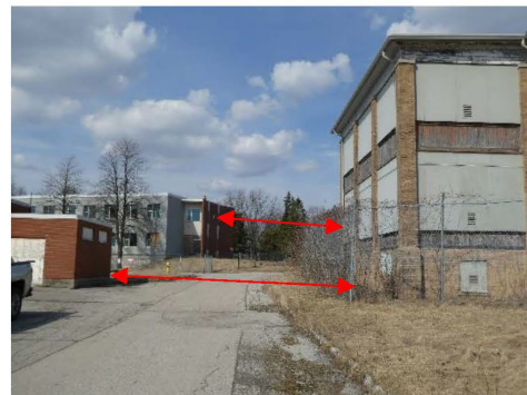
18m (60ft) to west structure demolition activity. And 37m(120ft) to north/west structure demolition activity.
