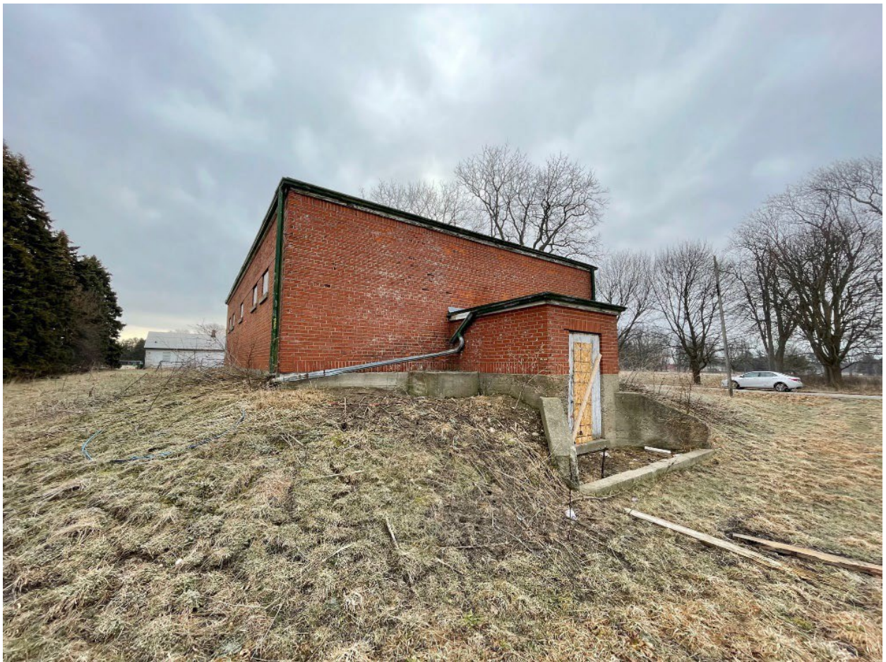
Figure 16. Building #4 (B12016) Granary, facing east – Zelinka, Mar 2022
