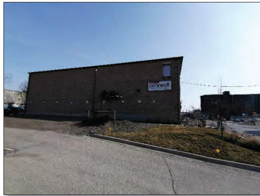
Figure 29: West elevation looking eastward (MHBC, 2022).
