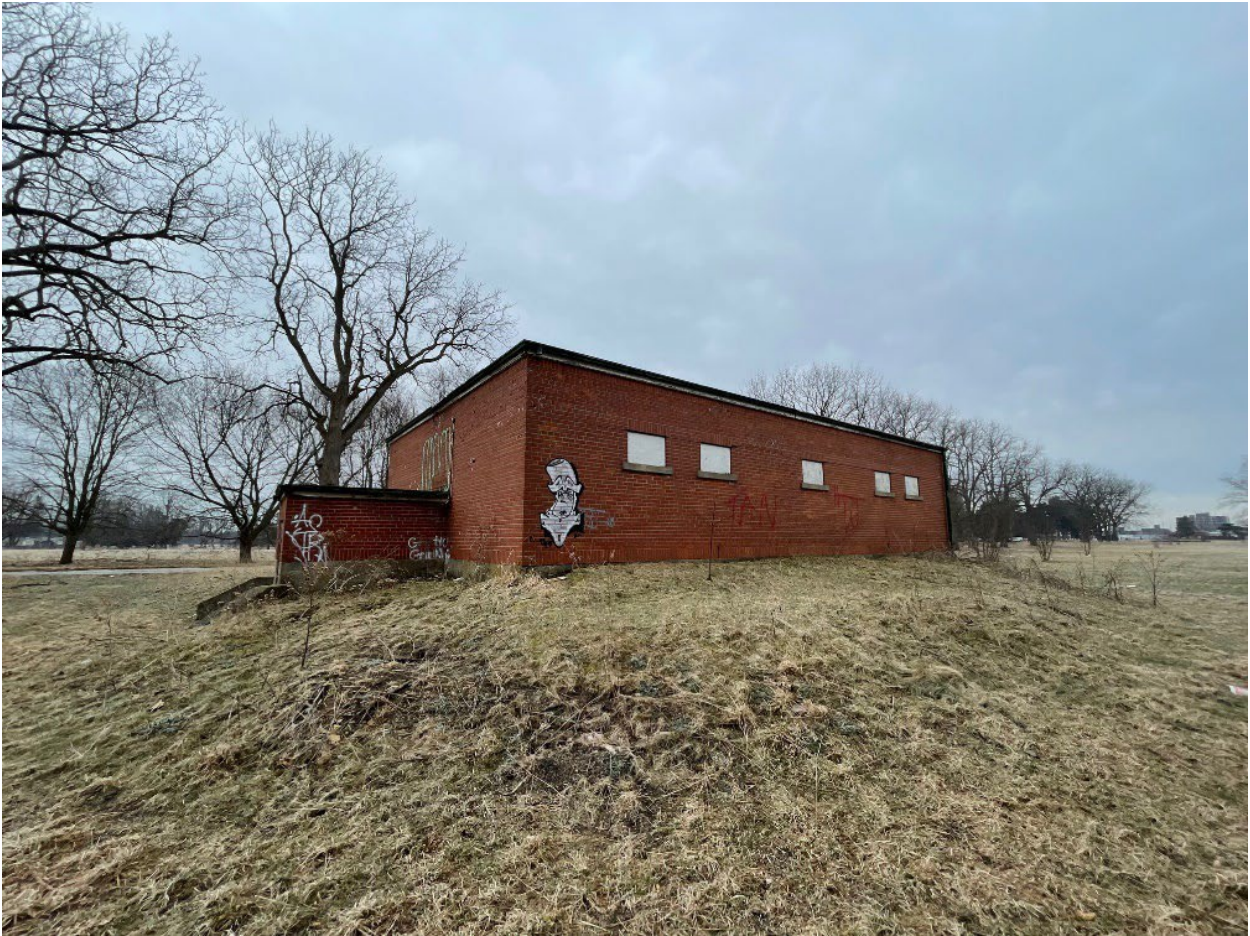
Figure 18. Building #4 (B12016) Granary, facing south-west – Zelinka, Mar 2022
