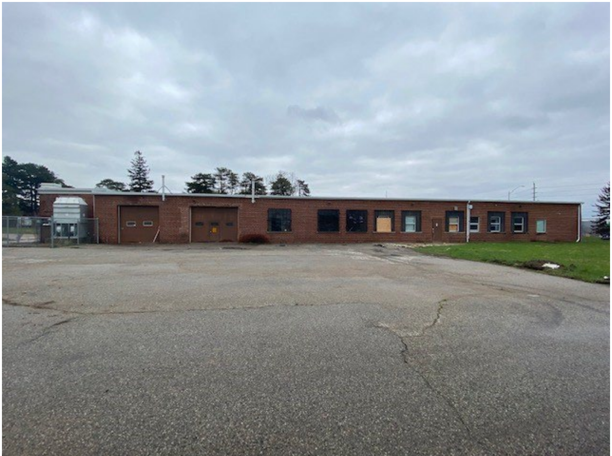
Figure 8. Building #2 (B12150) Ontario Government Building, facing south – L Dent, May 2022
