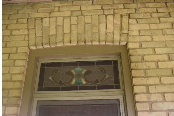
Plate 20: Stained glass transom, looking north
