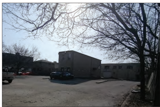
Figure 31: North (rear) elevation looking south-east (MHBC, 2022).
