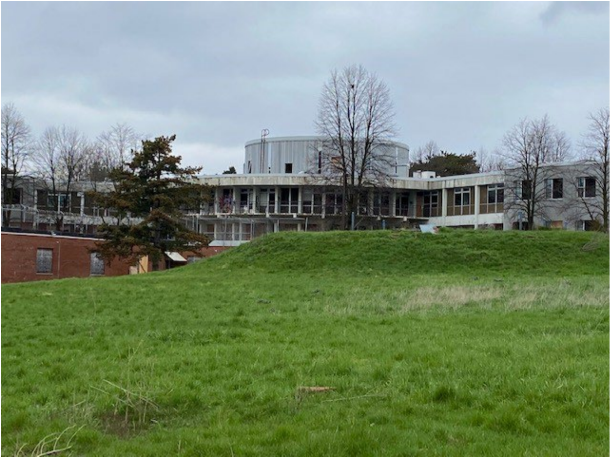
Figure 5. Building #1 (B12013) North Pavilion Building, facing north-west – L Dent, May 2022
