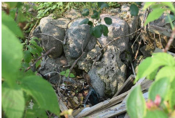
Plate 30: Remaining stone foundation, looking southwest
