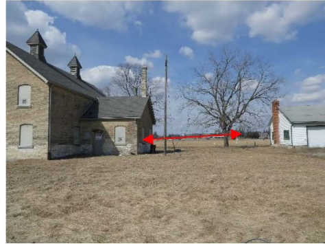
18m (60ft) to north structure demolition activity.
