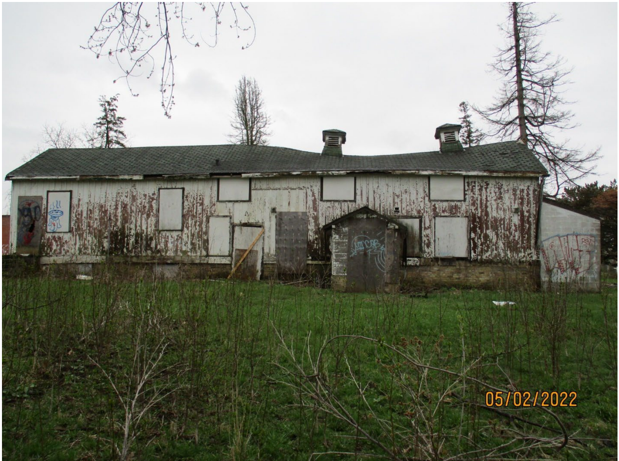
Figure 22. Building #6 (B17057) Potting Shed, facing south – M. Greguol, May 2022
