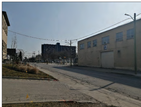
Figures 3 & 4: (above) View of surrounding area looking westward from subject property along the north side of Simcoe Street; (below) View of surrounding area looking eastward from subject property (MHBC, 2022).
