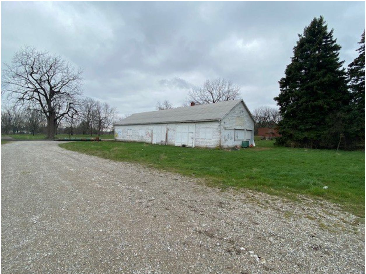
Figure 20. Building #5 (B16183) Soccer Shed, facing south-west – L Dent, May 2022
