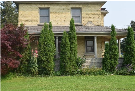
Plate 13: Lawn, shrubs, and perennials, looking north
