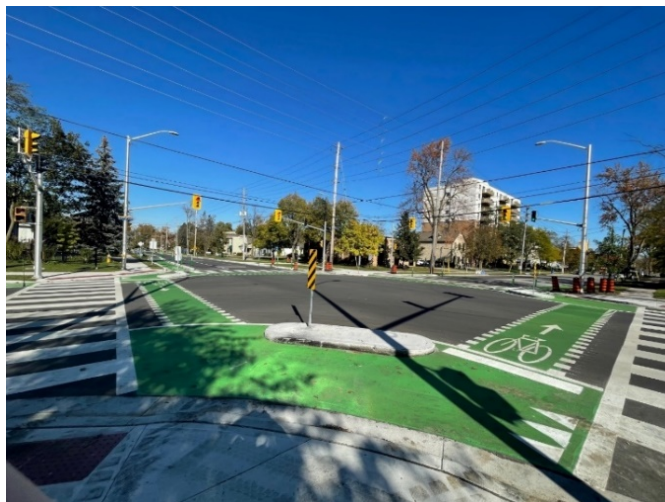
New bike lanes at Colborne and Central intersection
