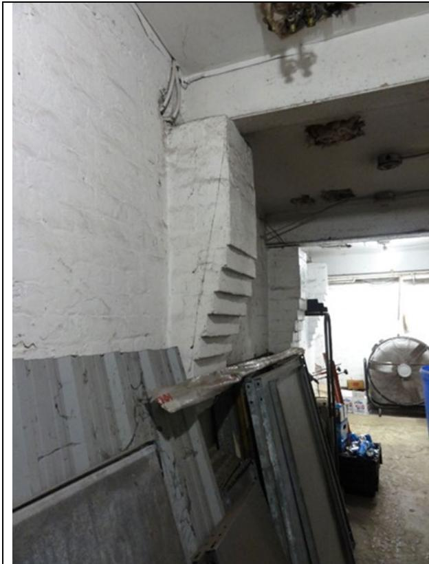
Image 5: Stacked corbelled brick support – primary building basement
