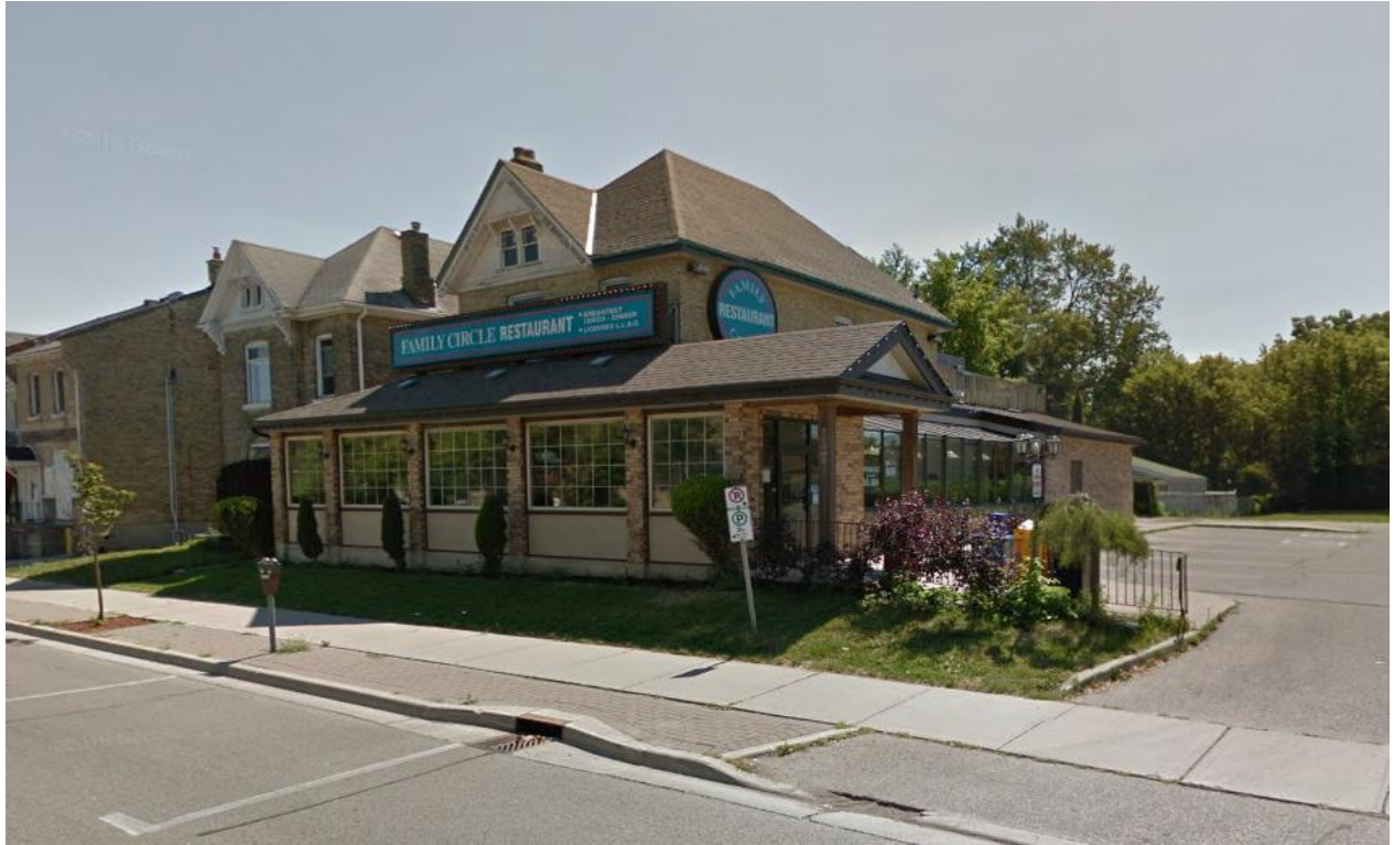
3. Family Circle restaurant in the south portion of the subject lands. To be demolished.
