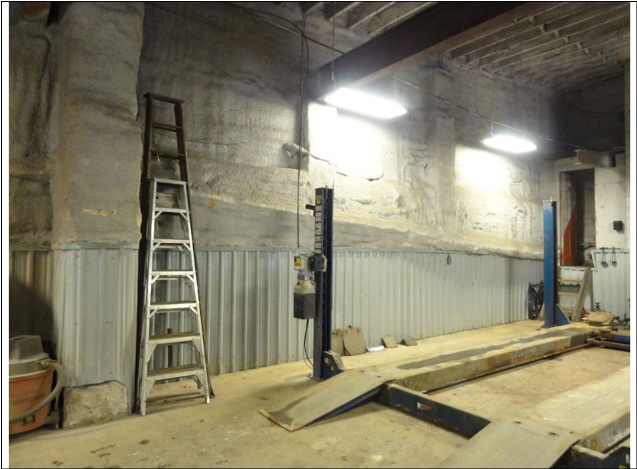
Image 11: Interior view of old wash house
