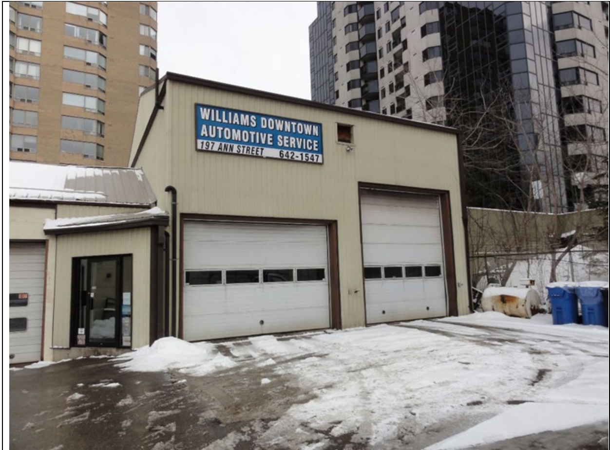
Image 13: Exterior view of contemporary garage – facing east
