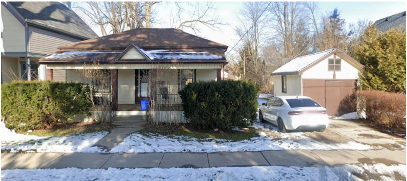
Image 3: 18 Byron Avenue East, Front/South Elevation (present day). Note one storey massing, form, and covered porch with triangular pediment above the entrance steps to the porch as well as original location of double-hung sash windows, and wooden deck. While some original features appear to remain, many have been replaced, such as openings, roofing and cladding. Source: Google Streetview, 2021.
