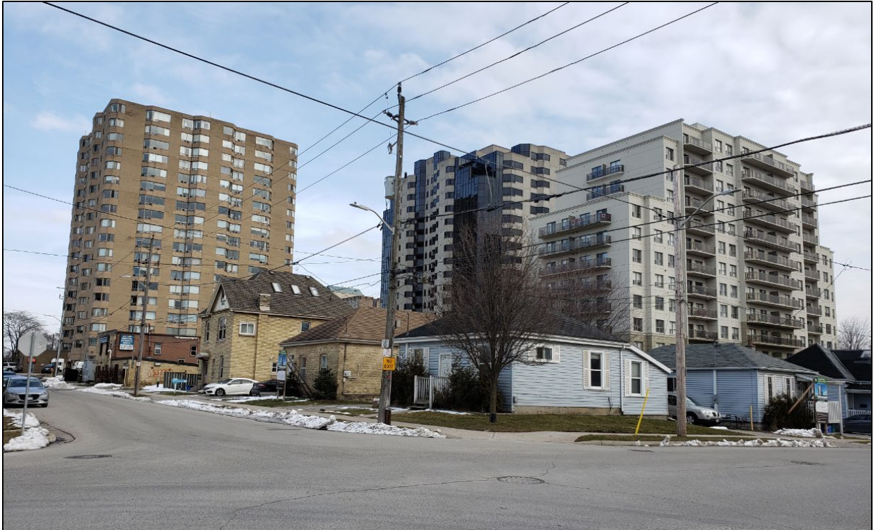
Figure 1: Northwest view of property – intersection of Ann Street and St. George St
