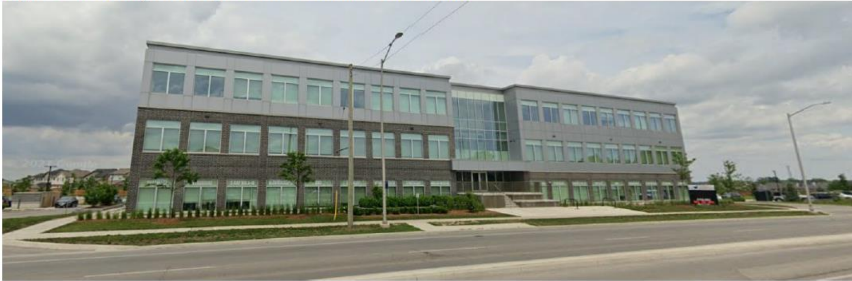
Figure 2 – Existing Building and Interface with Public Realm
