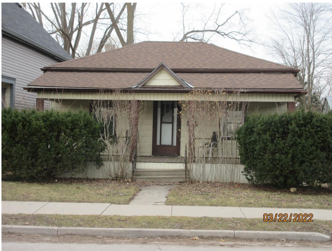
Image 3: Photograph of the subject dwelling located at 18 Byron Avenue East (2022).
