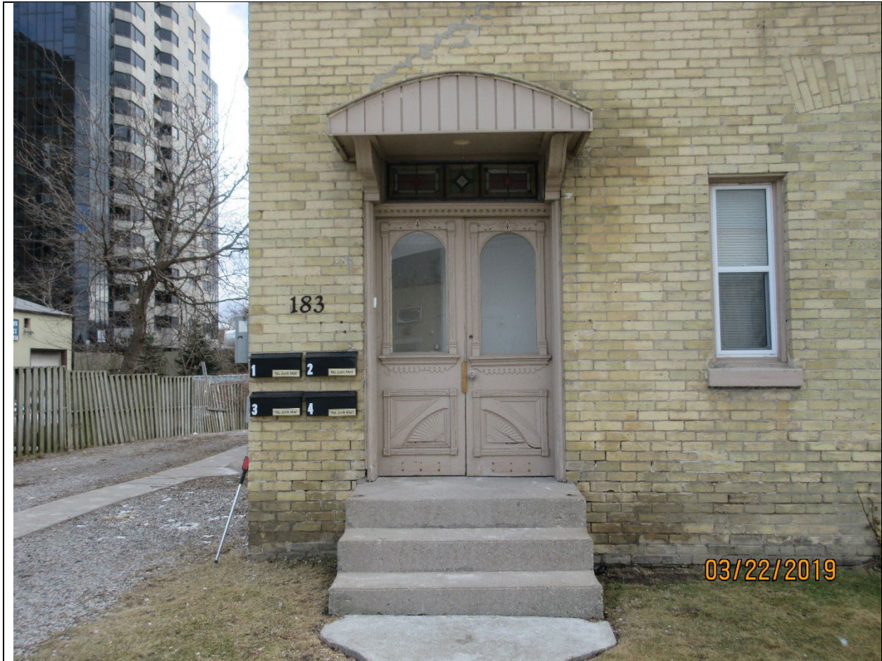
Image 20: 183 Ann Street – front entrance door detail (K. Gonyou, Mar 22, 2019)
