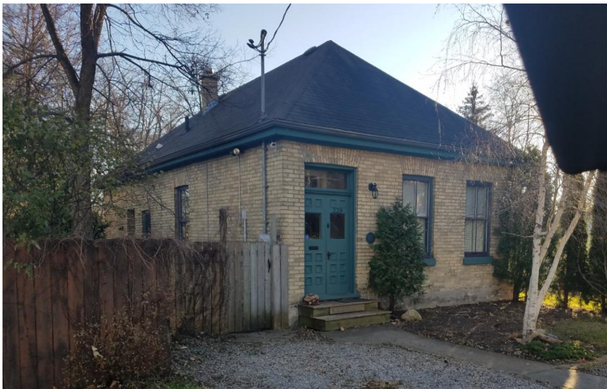
8. 239 Hill Street looking south
