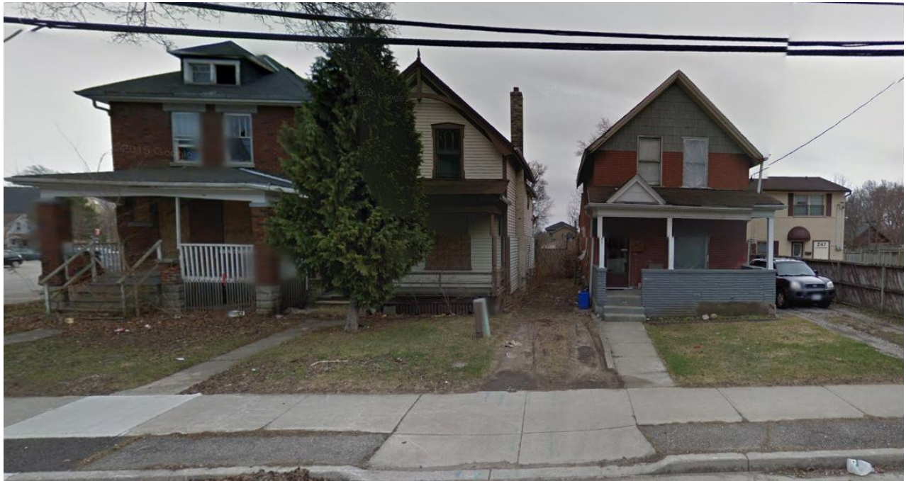
4. Single detached homes on Grey Street in the east portion of the subject lands. To be demolished.
