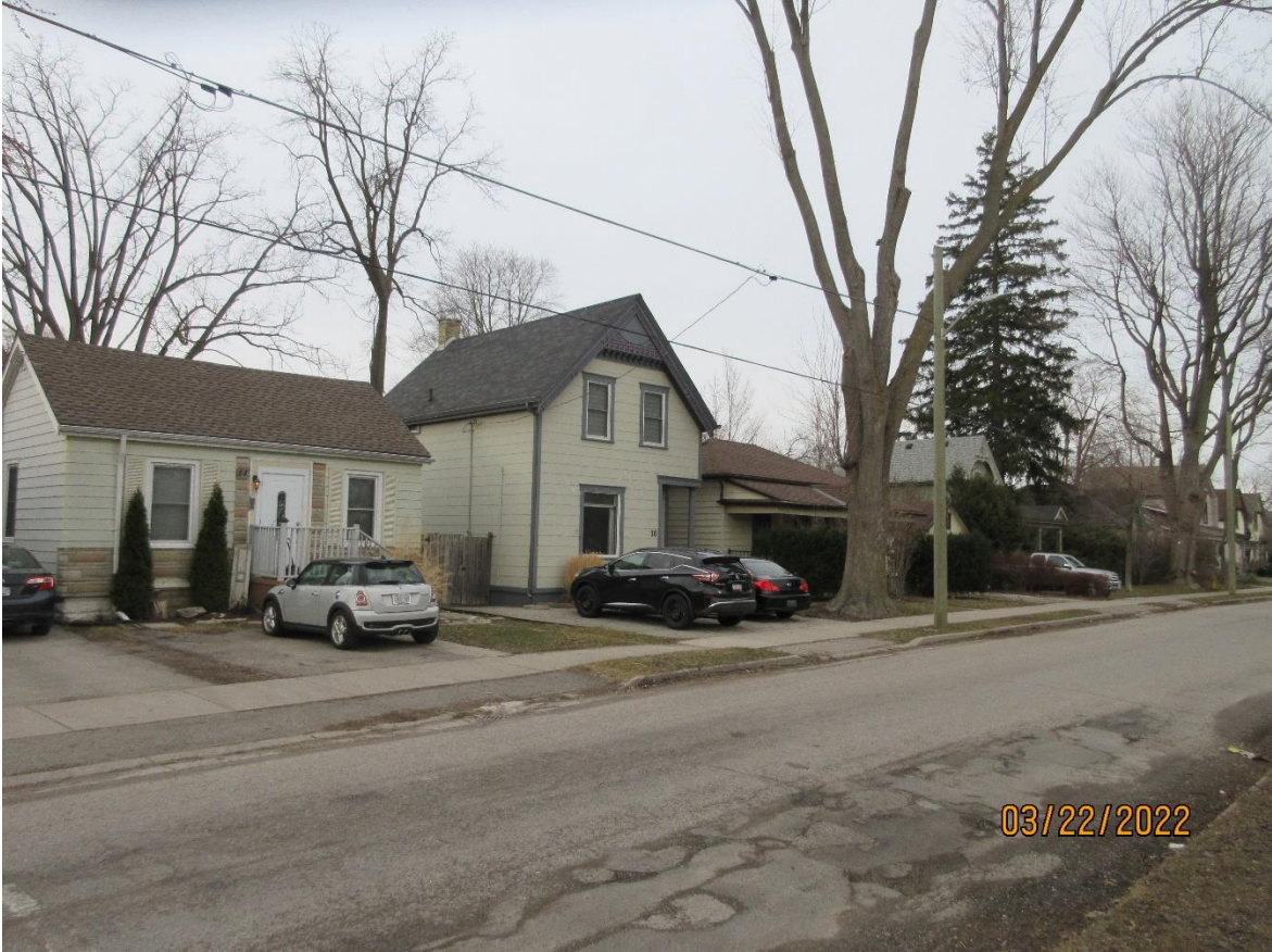
Image 8: View looking northeast along Byron Avenue East showing the context of the subject property including the small scale and massing of the dwelling within the surrounding area (2022).
