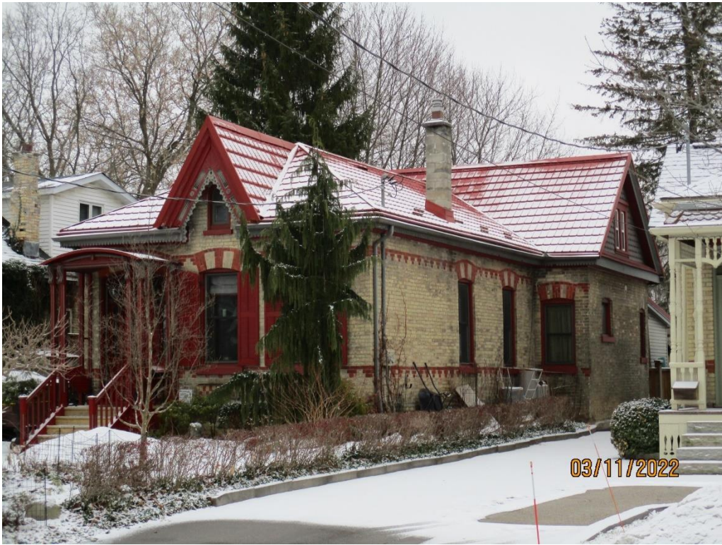
Image 13: Photograph of the dwelling located at 43 Bruce Street showing a rear addition to the existing single storey cottage. In this compatible addition, the use of a cross-gable has been used to minimize the visibility of the increase in building height at the rear of the dwelling (2022).
