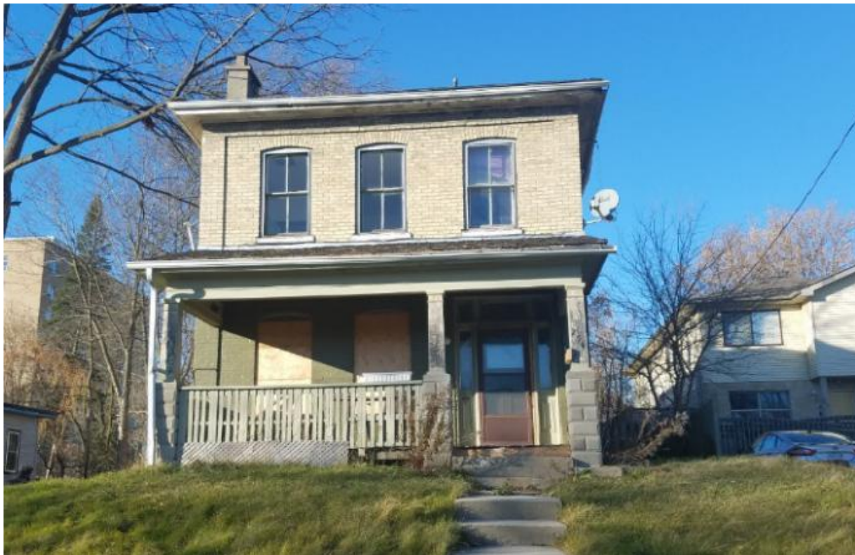
7. 254 Hill Street looking north
