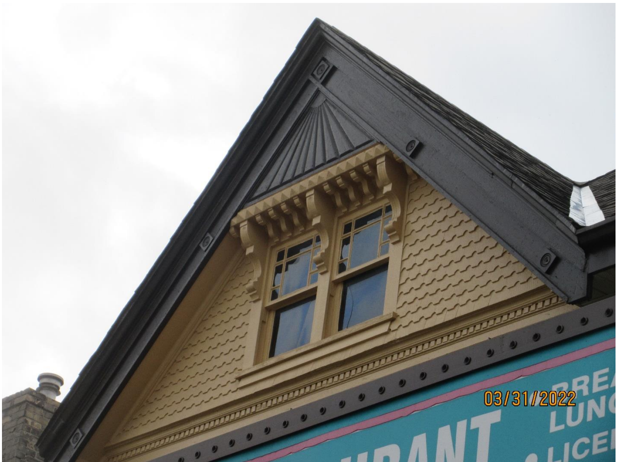
Image 4: Detail of the Queen Anne Revival detailing of the front gable, including the wood shingle imbrication, brackets, bargeboard, dentil moulding, and sunburst motif in the apex. The fenestration of the upper sash of the window is also in the Queen Anne Revival style.
