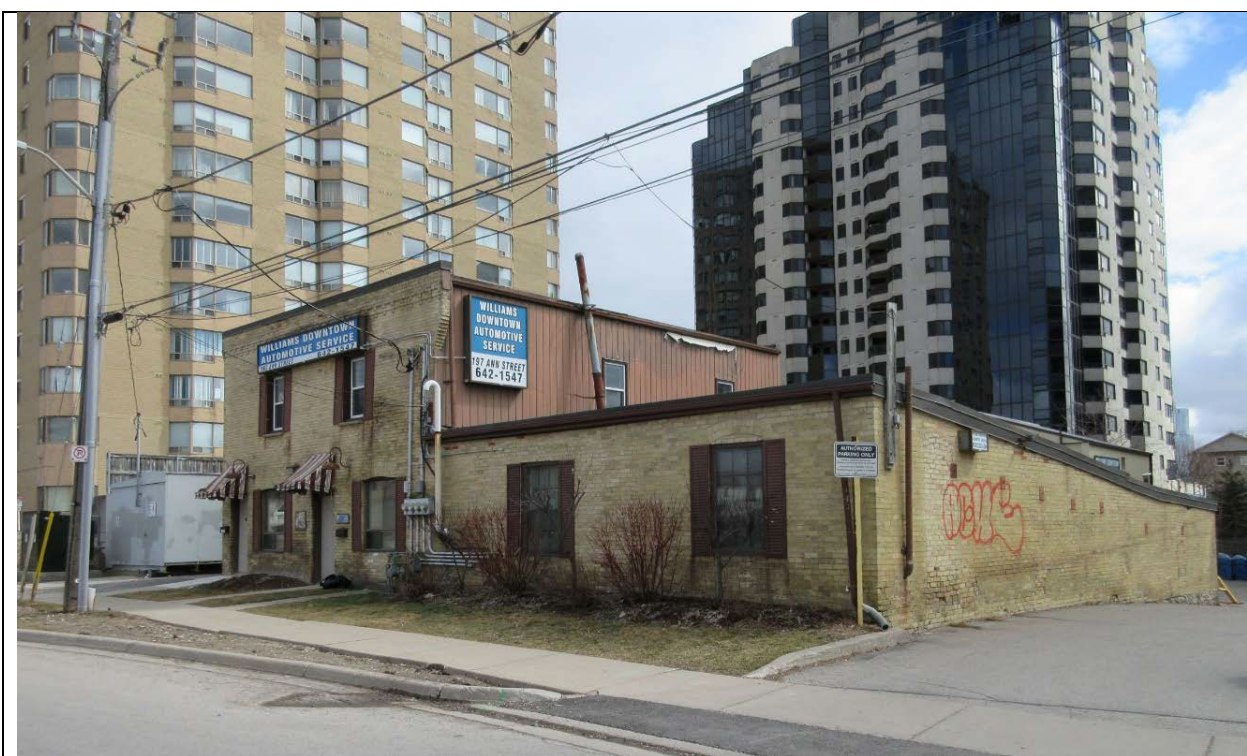
Image 2: View of façade – primary building and adjacent 'old wash house'
