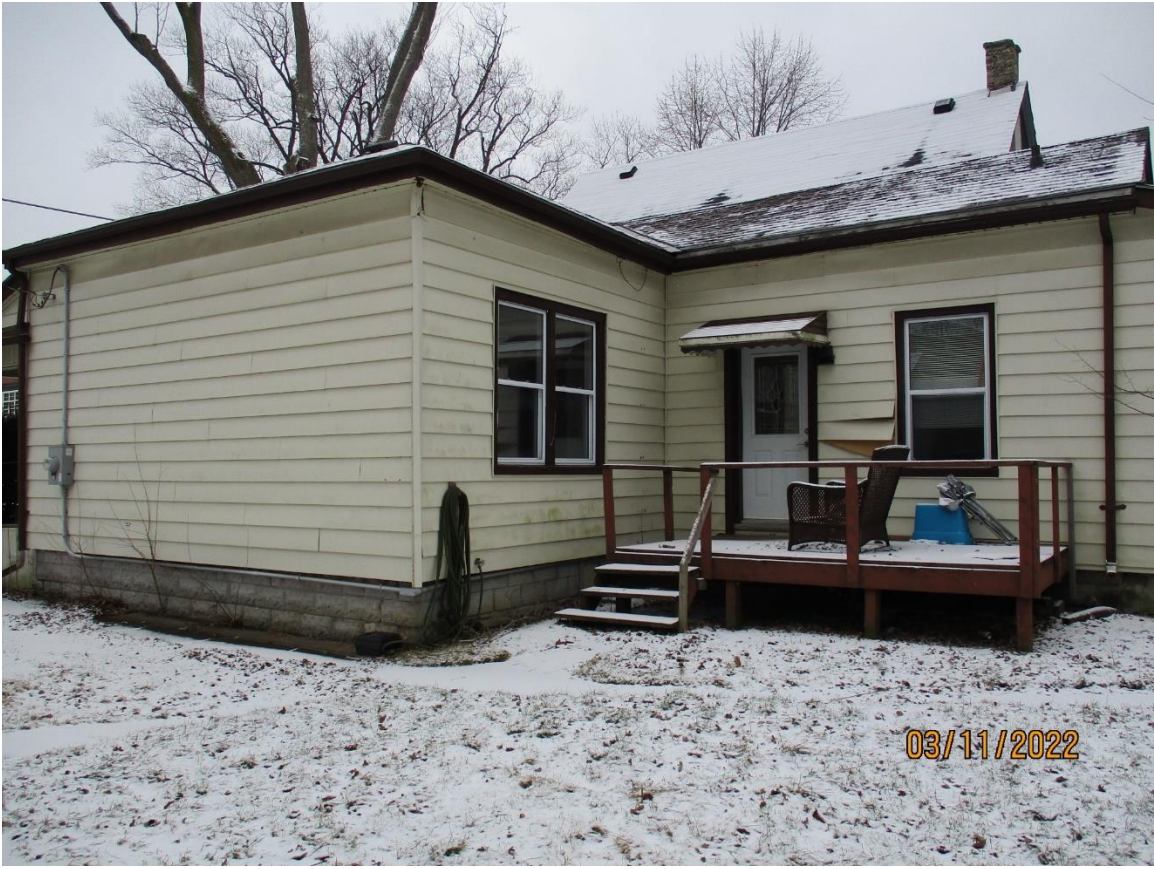
Image 5: Photograph of the rear of the dwelling at 18 Byron Avenue East showing the first rear addition on the existing dwelling (2022).
