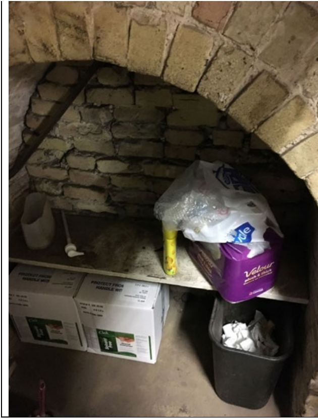
Image 7: Rounded arch opening – view, old washroom to primary building basement
