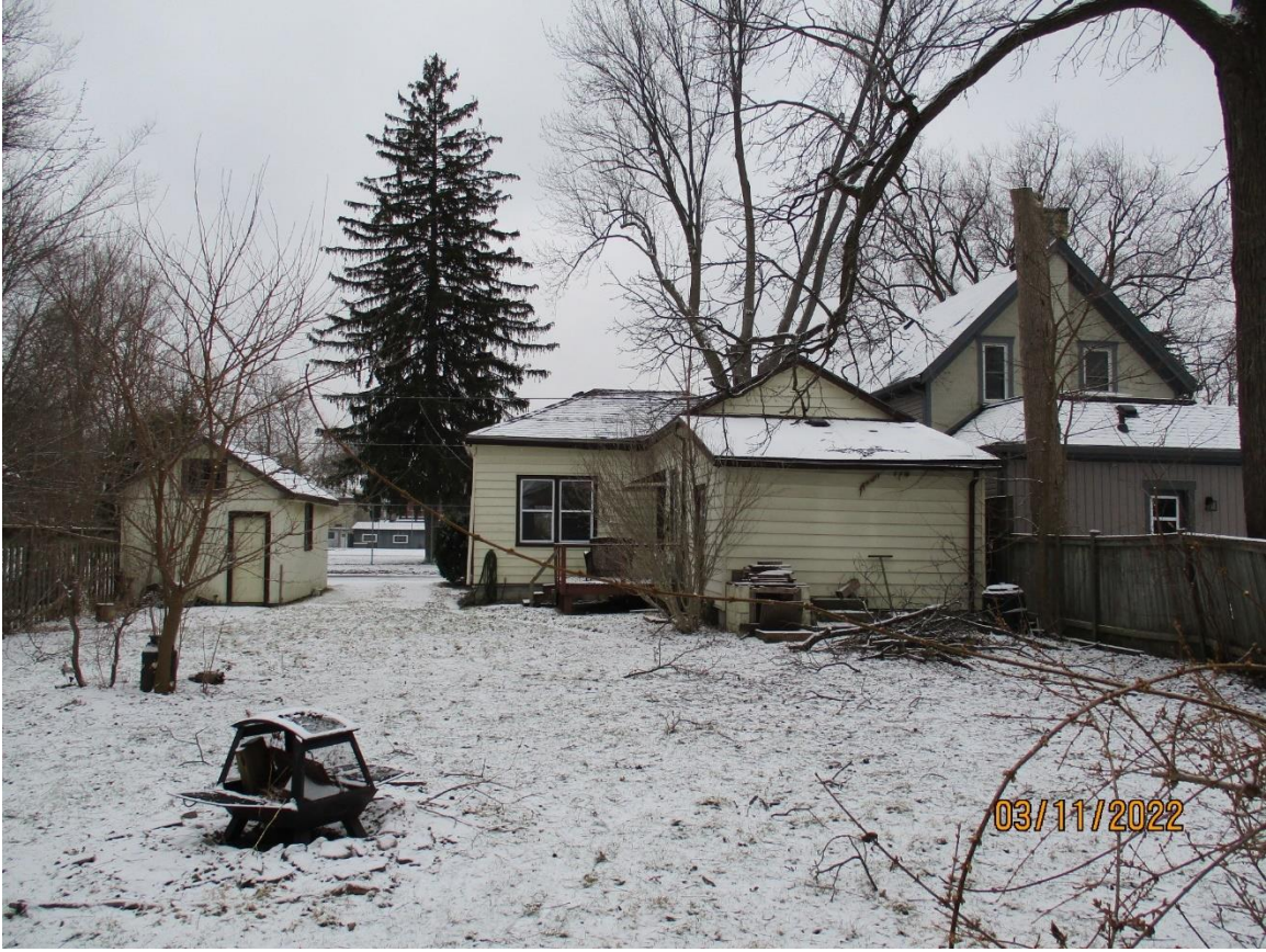
Image 6: Photograph of the rear of the dwelling at 18 Byron Avenue East showing the two rear additions, the detached garage, and the adjacent property at 16 Byron Avenue East (2022).
