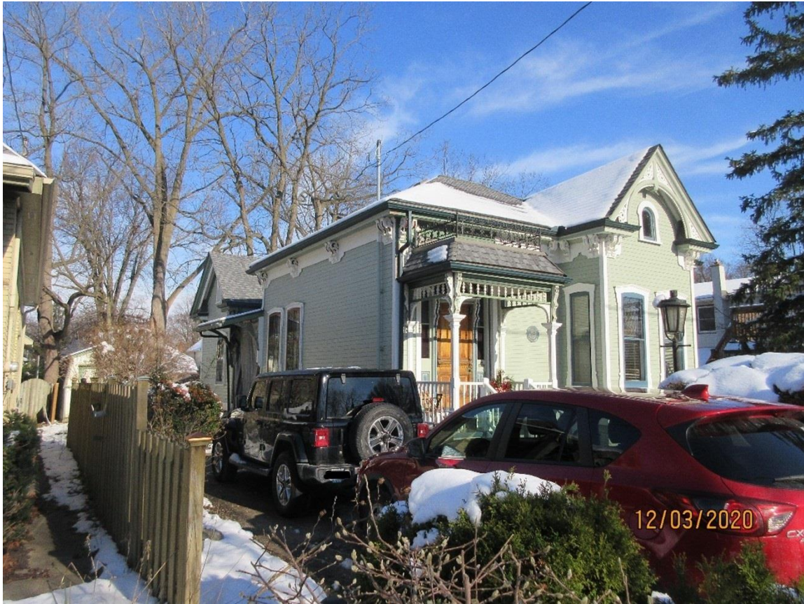
Image 17: Photograph of the dwelling located at 50 Bruce Street showing a rear addition added to the rear of the dwelling in a manner that conserves the heritage attributes of the property. Though likely a historic addition, the cottage retains its form and the addition is situated at the rear of the dwelling (2022).
