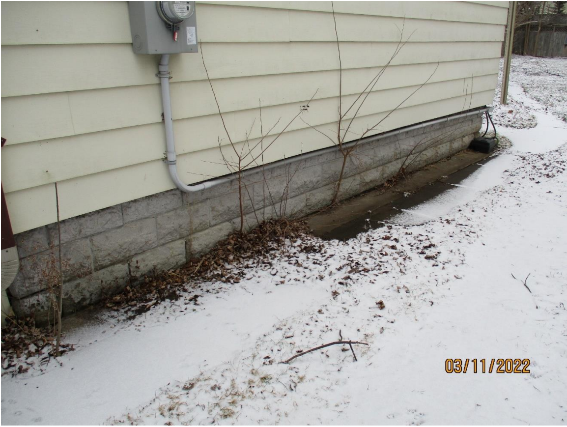
Image 7: Photograph of the foundation of the dwelling at 18 Byron Avenue East, showing the rusticated concrete blocks (2022).
