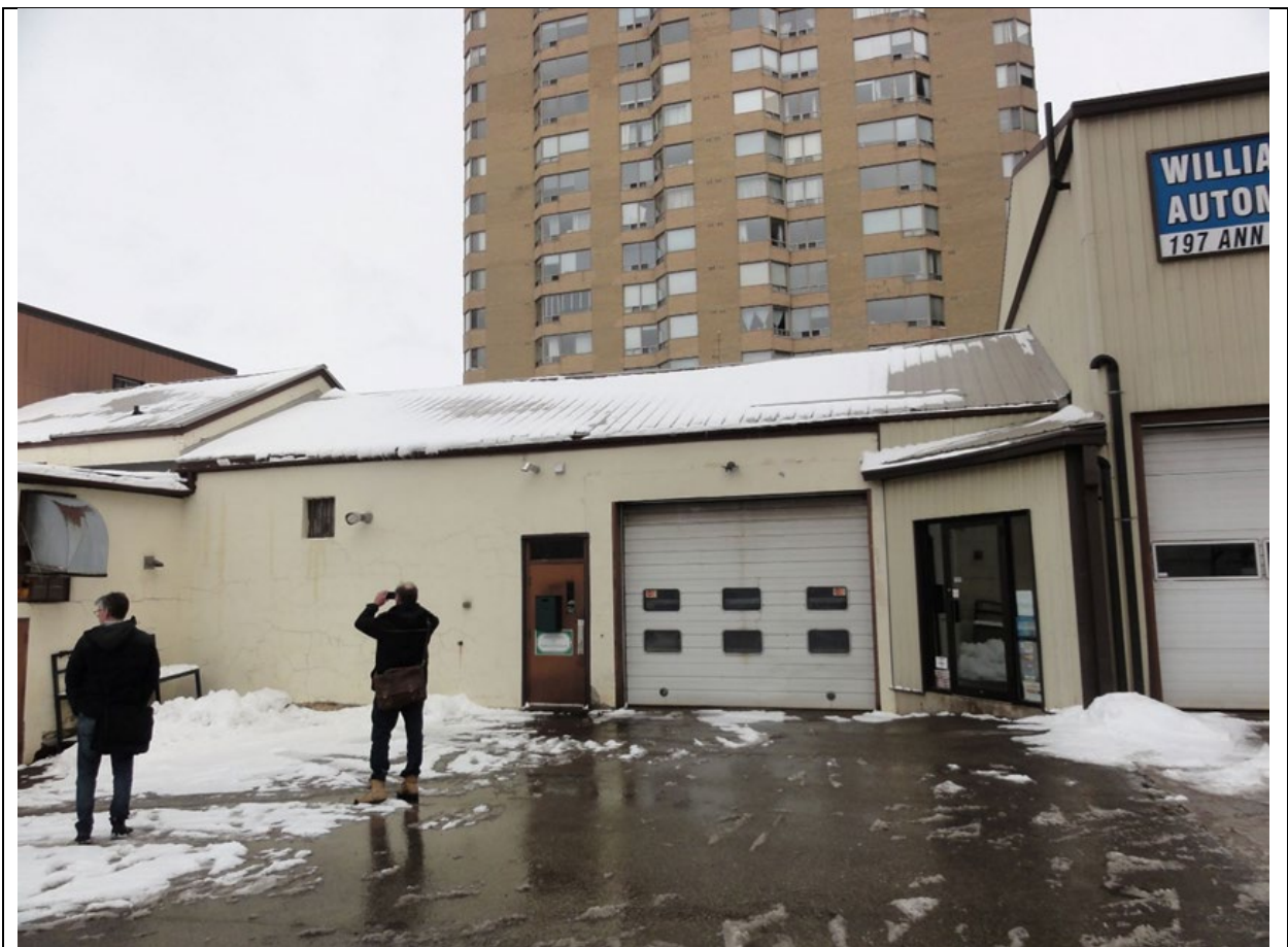
Image 12: Exterior view of south extension – facing east
