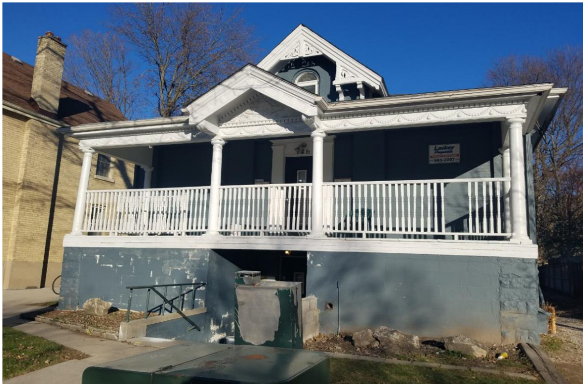
11. 146 Wellington Street looking east
