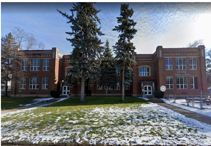
Image 14: 130 Wharncliffe Road S. (Victoria Public School), West Elevation. Google Streetview 2021.
