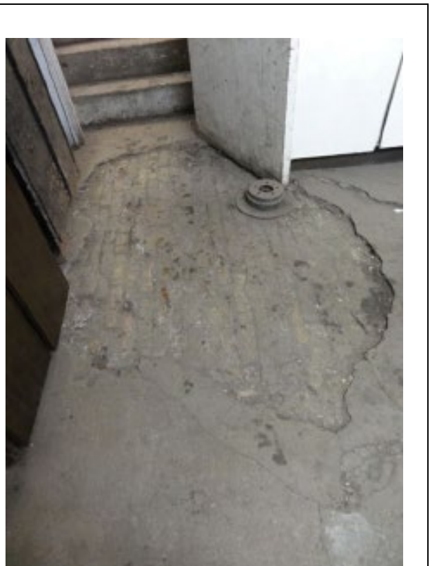
Image 6: Detail of partially exposed original brick floor – primary building
