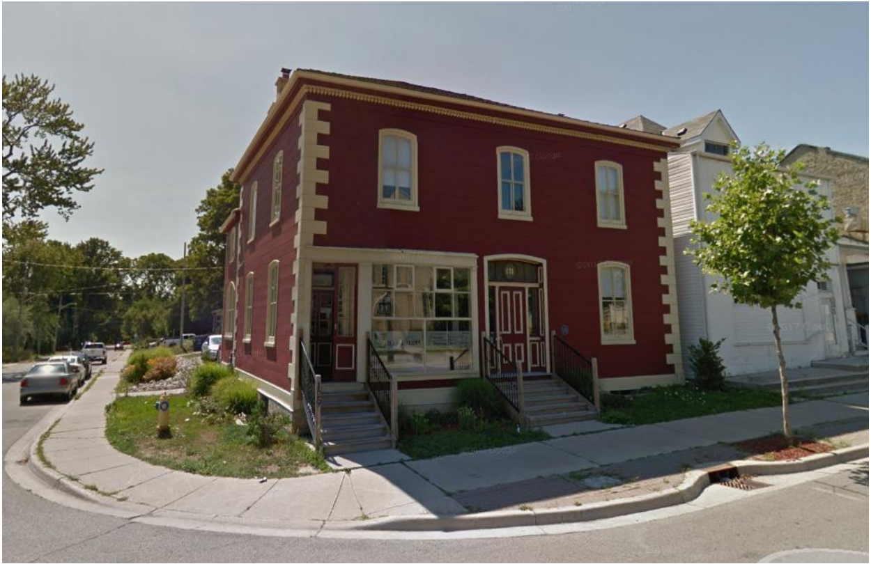
5. 129, 131 Wellington Street looking west
