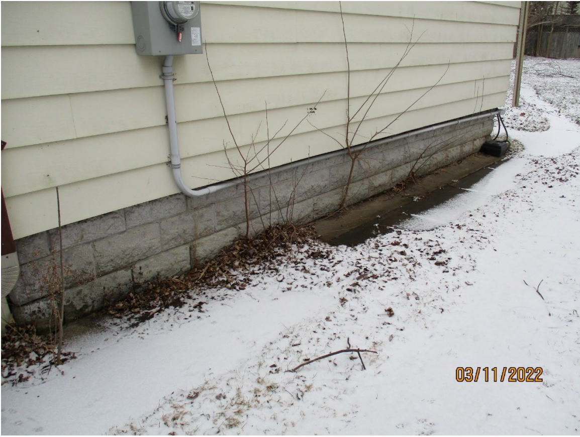
Image 7: Photograph of the foundation of the dwelling at 18 Byron Avenue East, showing the rusticated concrete blocks (2022).
