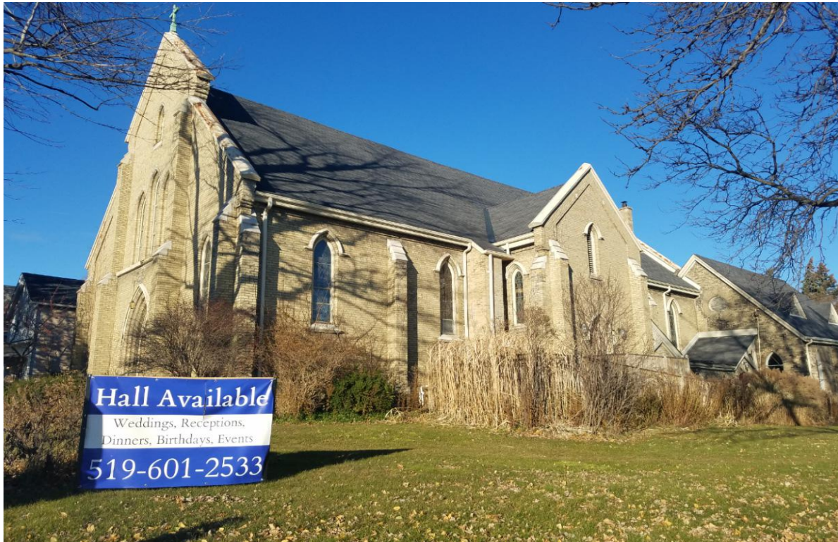
10. 138 Wellington Street looking east
