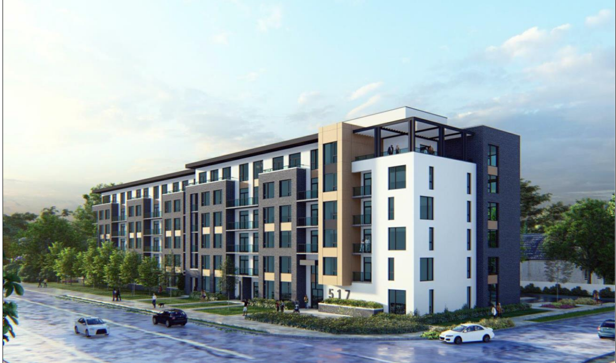
Figure 6: View from Intersection of Fanshawe Park Road East and Geary Avenue
