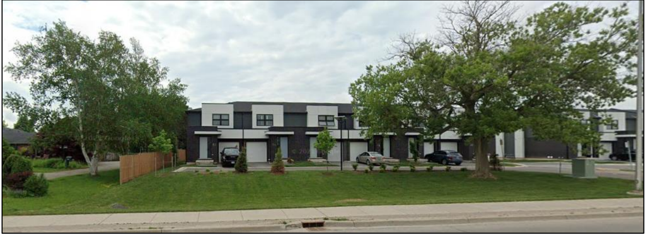
Figure 12. View of the Townhouse Development to the Immediate West of the Subject Lands (499 Sophia Crescent), Facing South on Gainsborough Road (June 2021)
