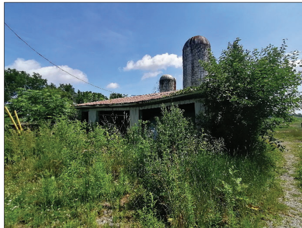
Figure 25: View of outbuilding 2 looking east (MHBC, 2021)
