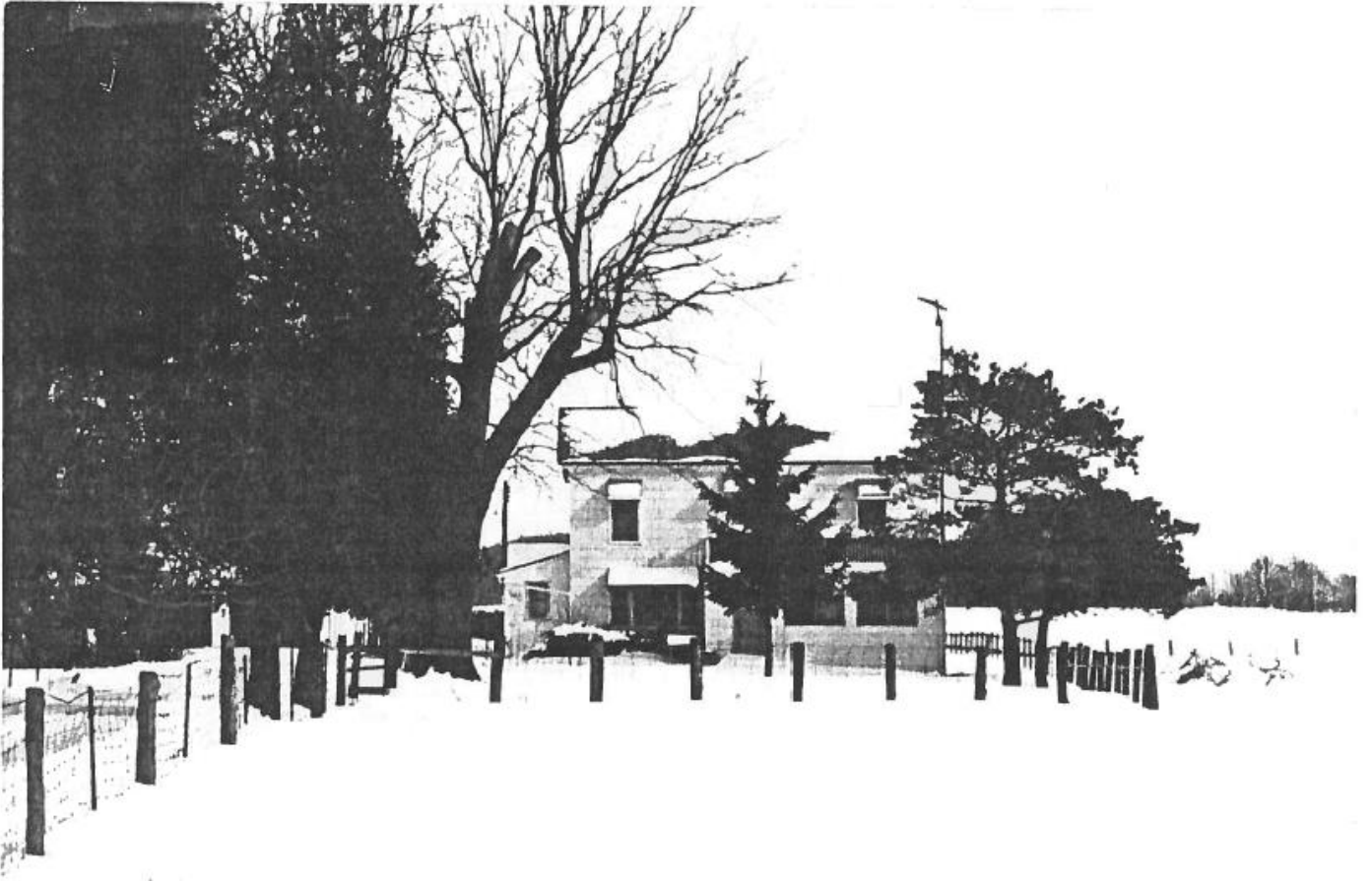
Image 1: Photograph of the property at 3700 Colonel Talbot Road from the Annexed Area Inventory (1993).
