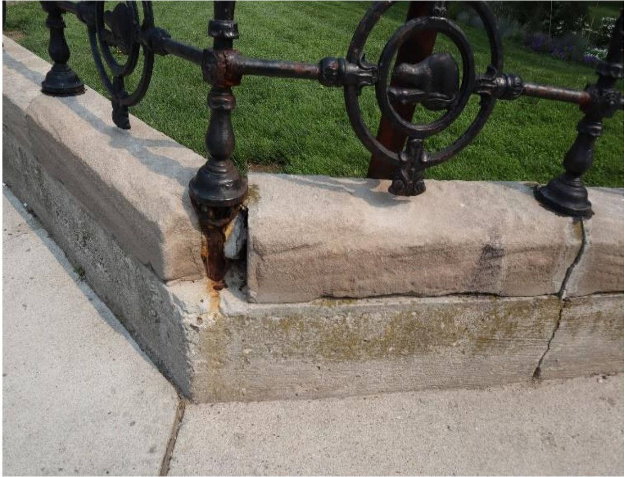
Photograph 29: Pin tie of a vertical rail post (AECOM, May 2021)
