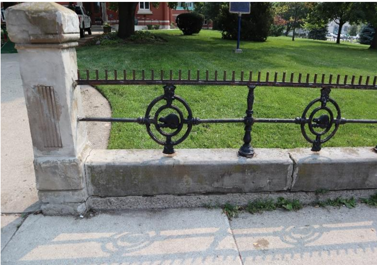
Photograph 39: Section of fence on Richmond Street with a modified top horizontal bar (AECOM, May 2021)
