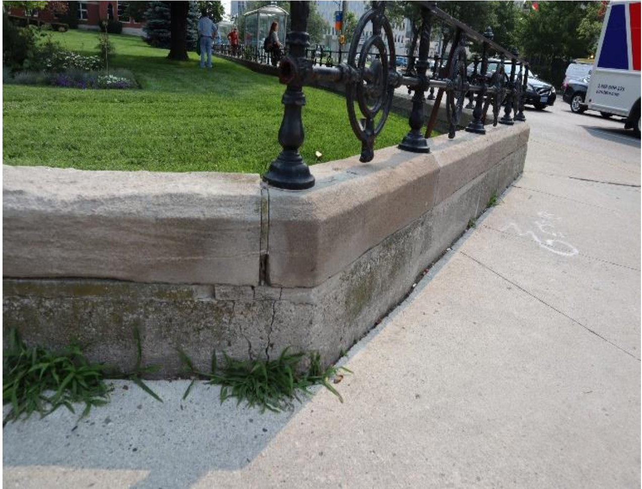
Photograph 28: Details of a corner of the beaver fence (AECOM, May 2021)
