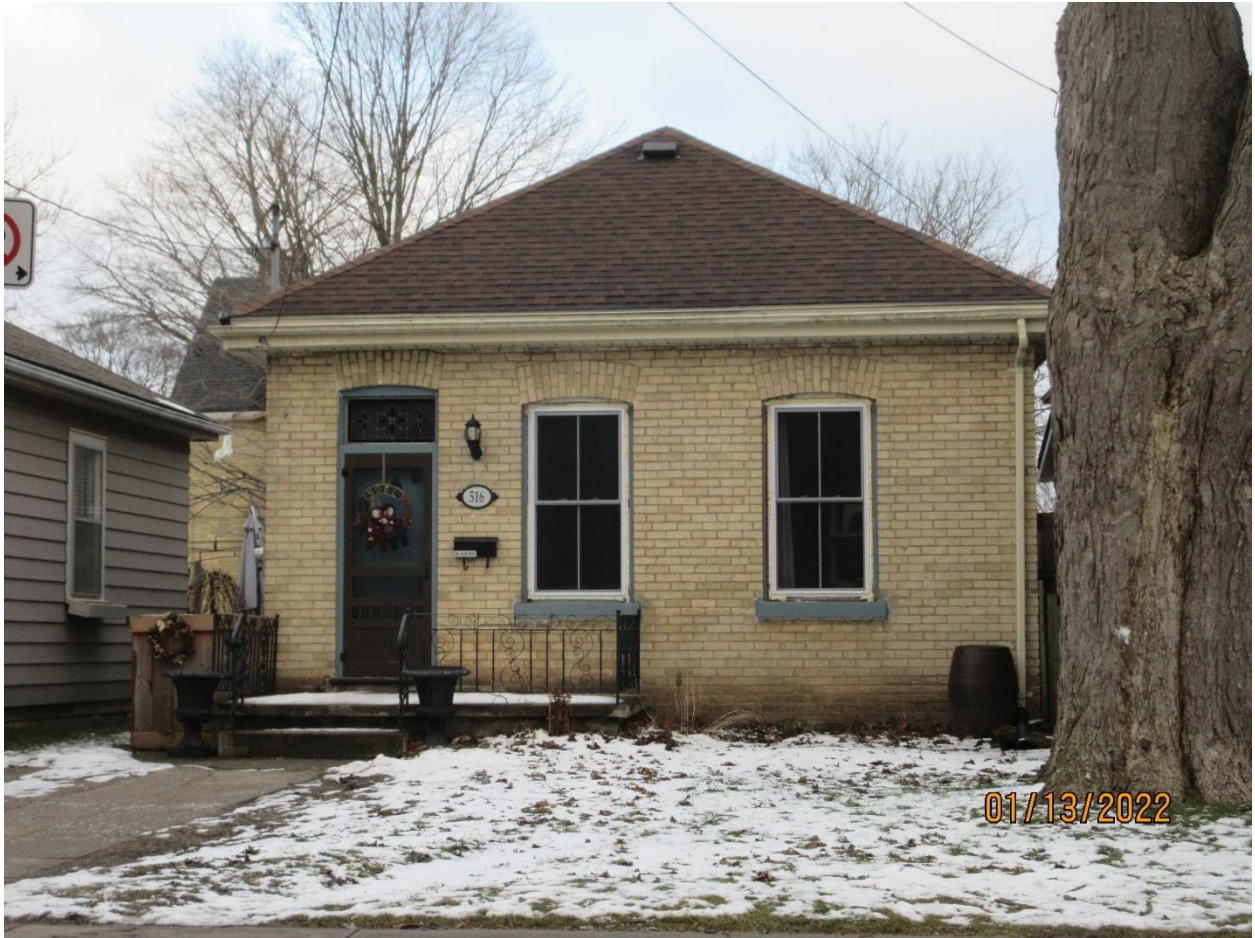
Image 3: Photograph of the house at 516 Elizabeth Street on January 13, 2022. Note the reinstated transom and replacement of the front windows.
