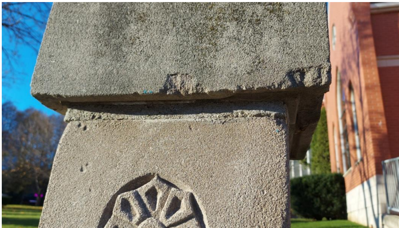
Photograph 16: View of the separate top cap of the end post with mortar layer with the end post (AECOM, November 2021)
