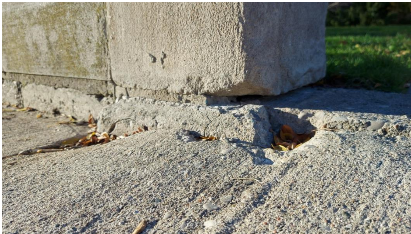
Photograph 17: End post placed on a mortar layer with a concrete foundation (AECOM, November 2021)
