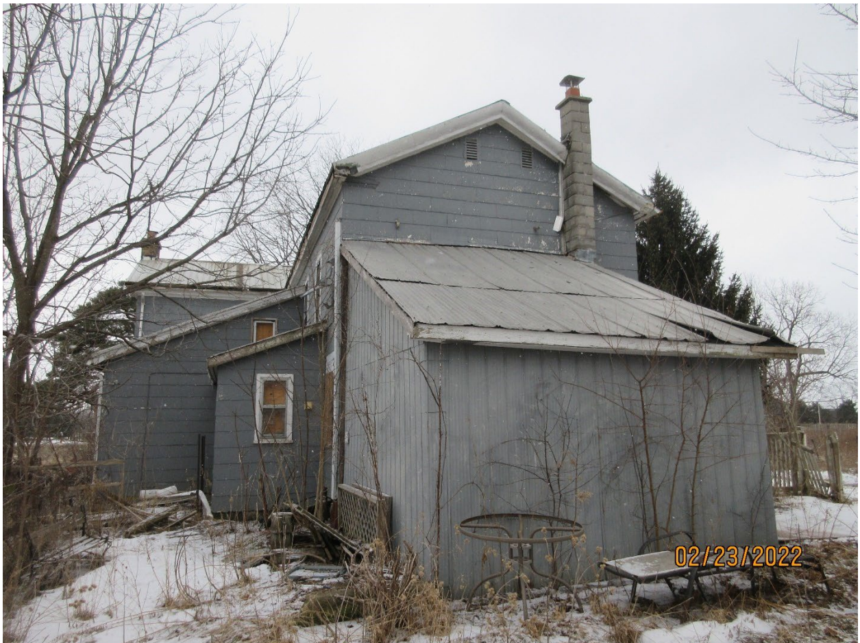
Image 6: View of the east elevation of the farmhouse at 3700 Colonel Talbot Road. Note the additions built onto the structure.
