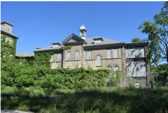
Photo 12: Infirmary south elevation of east wing looking north
