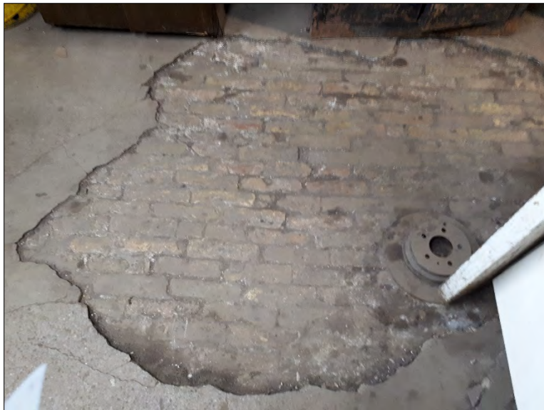
Figures 49 & 50: (above) Interior view of building Section 'C' showing corbelled brick supports in basement; (below) View of original brick flooring in basement of Section 'C' (Source:MHBC, 2019)
