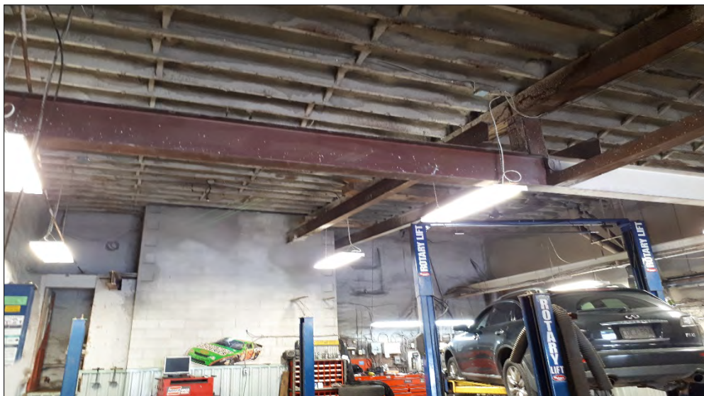
Figures 45 & 46: (above) Interior view of Florentine arched doorway within building Section 'B' (below) View of ceiling in Building Section 'B' with steel beams (Source: MHBC, 2019)
