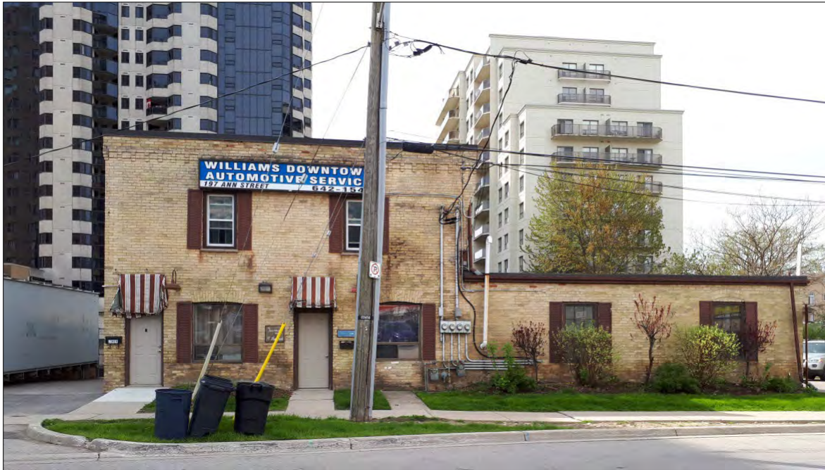
Figure 39: View of north (front) elevation (Source: MHBC, 2019)
