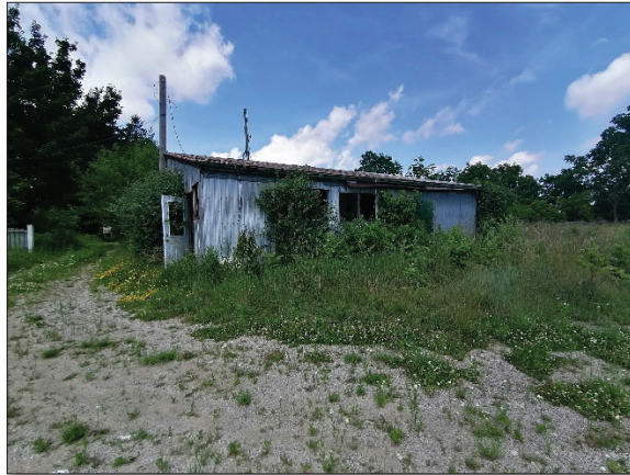
Figure 24: View of outbuilding 1 looking east (MHBC, 2021)
