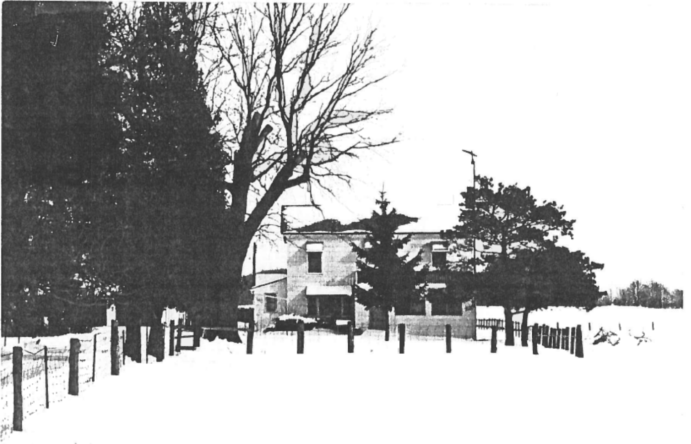
Image 1: Photograph of the property at 3700 Colonel Talbot Road from the Annexed Area Inventory (1993).
