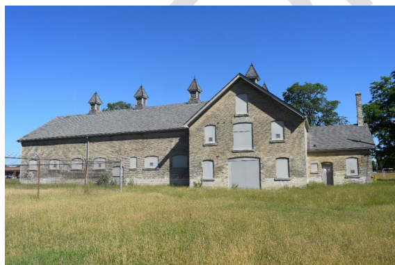
Photo 1: Horse Stable looking northwest
