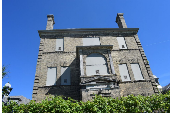
Photo 11: Infirmary south elevation of Administration Block looking north
