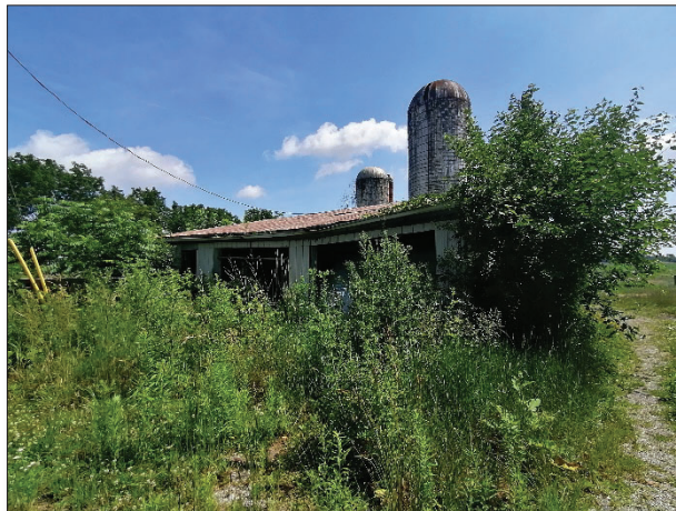
Figure 25: View of outbuilding 2 looking east (MHBC, 2021)
