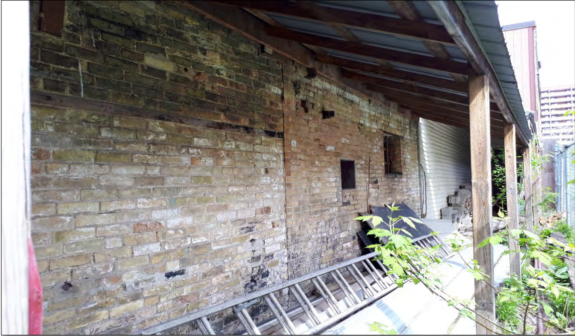
Figure 41: View of east elevation (Source: MHBC, 2019)
