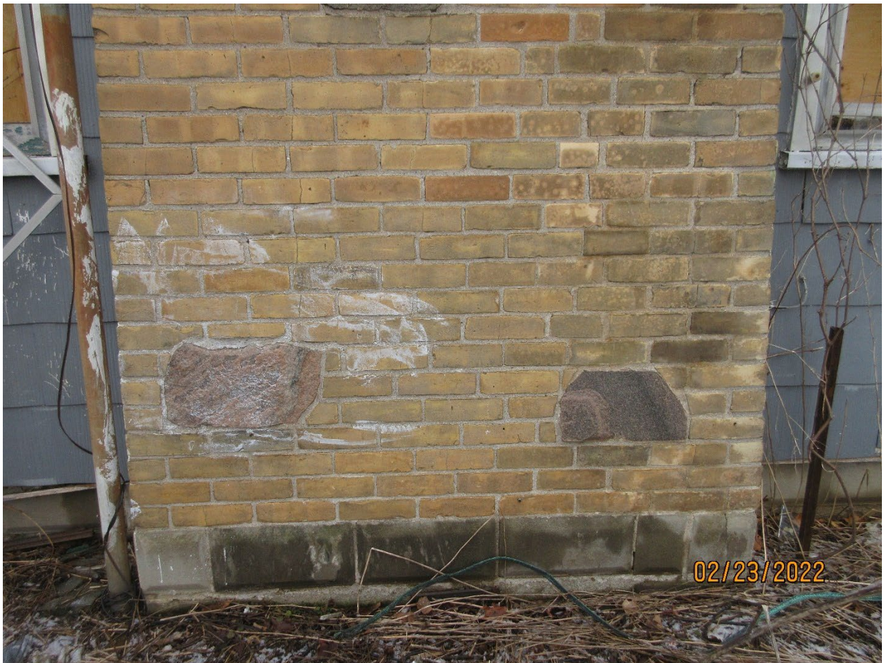
Image 10: Detail of the inset stone detailing in the brick masonry chimney on the south elevation.
