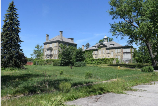
Photo 10: Infirmary south elevation looking northwest
