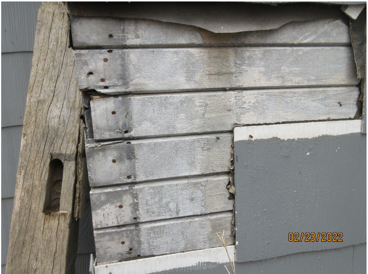
Image 8: Detail of the wood siding under the exterior cladding on the farmhouse at 3700 Colonel Talbot Road. Note the staining from previous paint, suggesting end boards.
