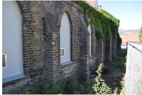
Photo 7: Chapel of Hope south elevation looking east
