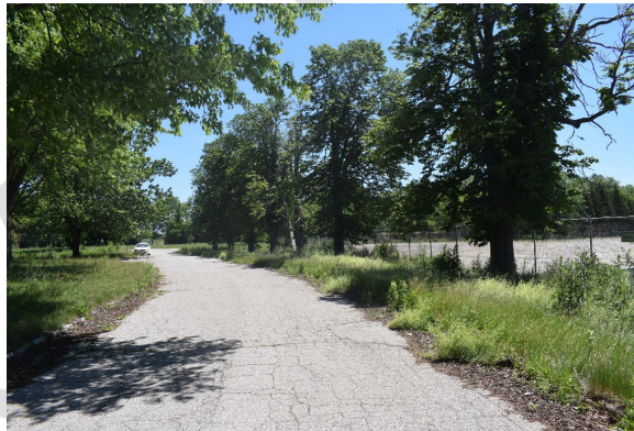
Photo 29: Driveway towards Ring Road looking southeast
