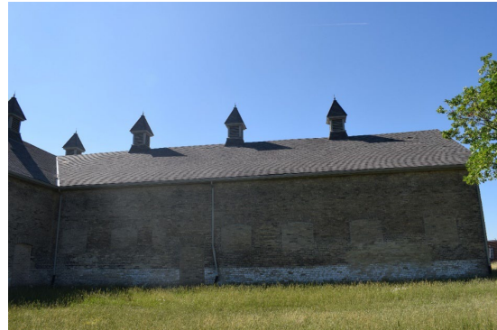
Photo 4: Horse Stable looking south
