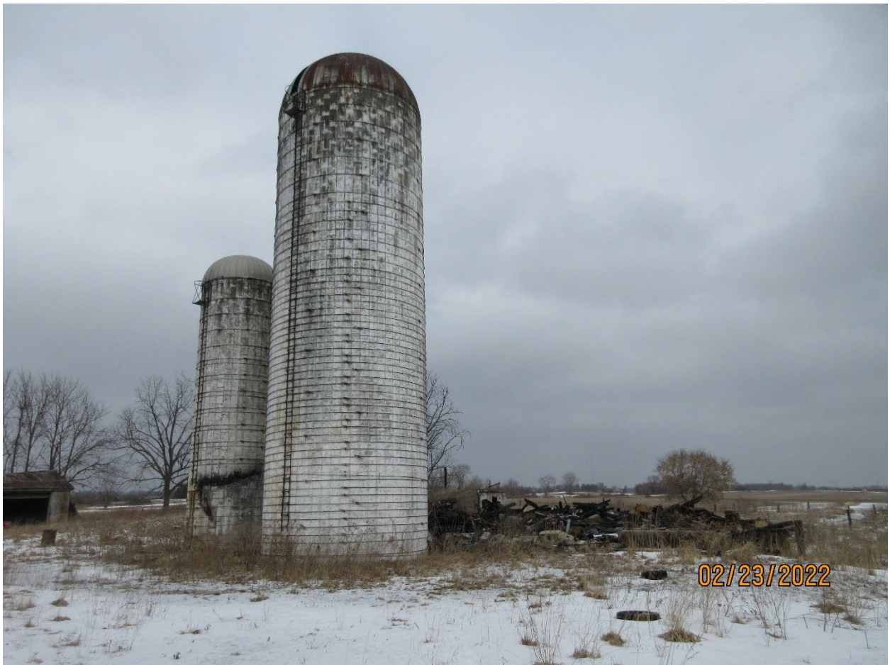
Image 14: Photograph of the two concrete block silos, with the remains of the barn at 3700 Colonel Talbot Road.
