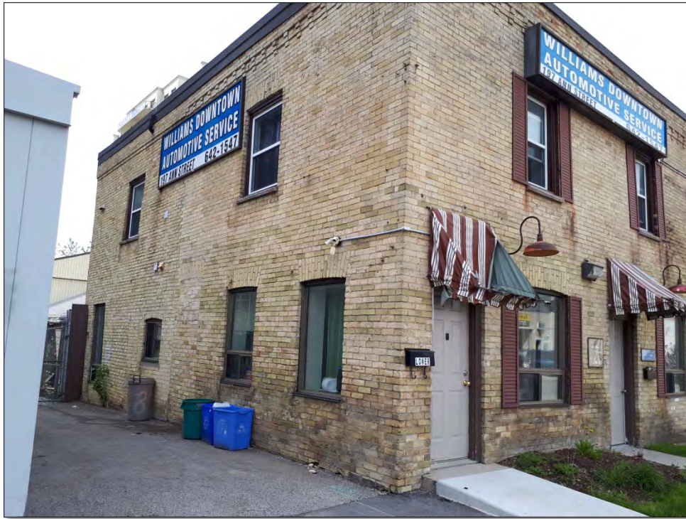
Figure 40: View of north (front) elevation (Source: MHBC, 2019)
