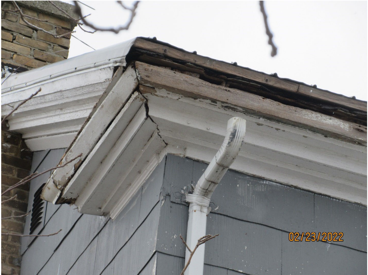
Image 9: Detail of the cornice and return eave of the farmhouse at 3700 Colonel Talbot Road.
