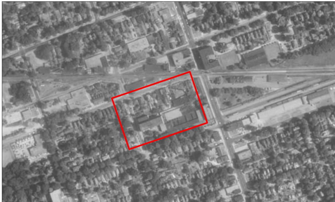
Figures 34 & 35: (above) 1945 aerial photograph; red outline identifies Ann street block bounded by Ann Street, Richmond Street, St. George Street and Mill Street; (below) above) 1955 aerial photograph; red outline identifies Ann street block bounded by Ann Street, Richmond Street, St. George Street and Mill Street; (Courtesy of Western University).
