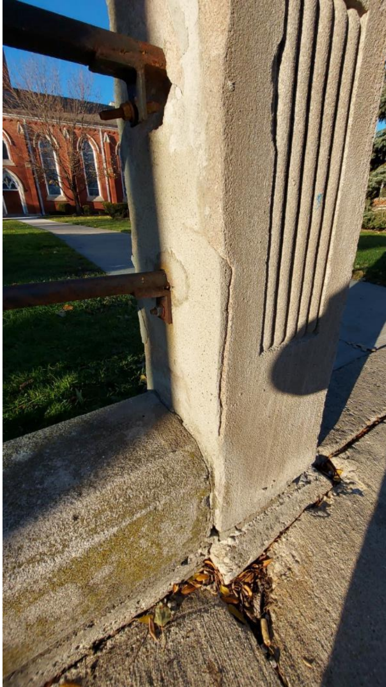
Photograph 21: End post with localized repairs (AECOM, November 2021)
