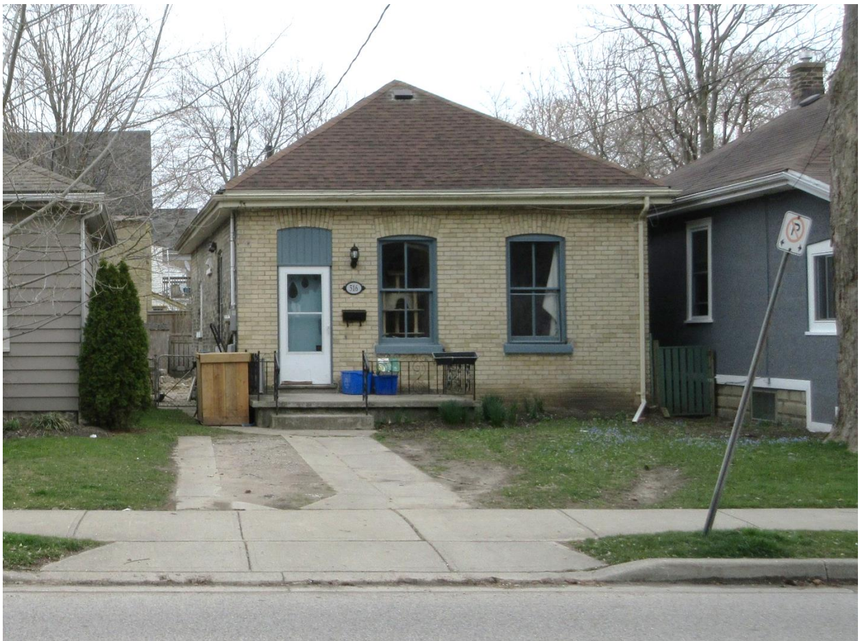
Image 2: Photograph of the house at 516 Elizabeth Street on April 24, 2020. Note the painted wood, two-over-two wood windows.
