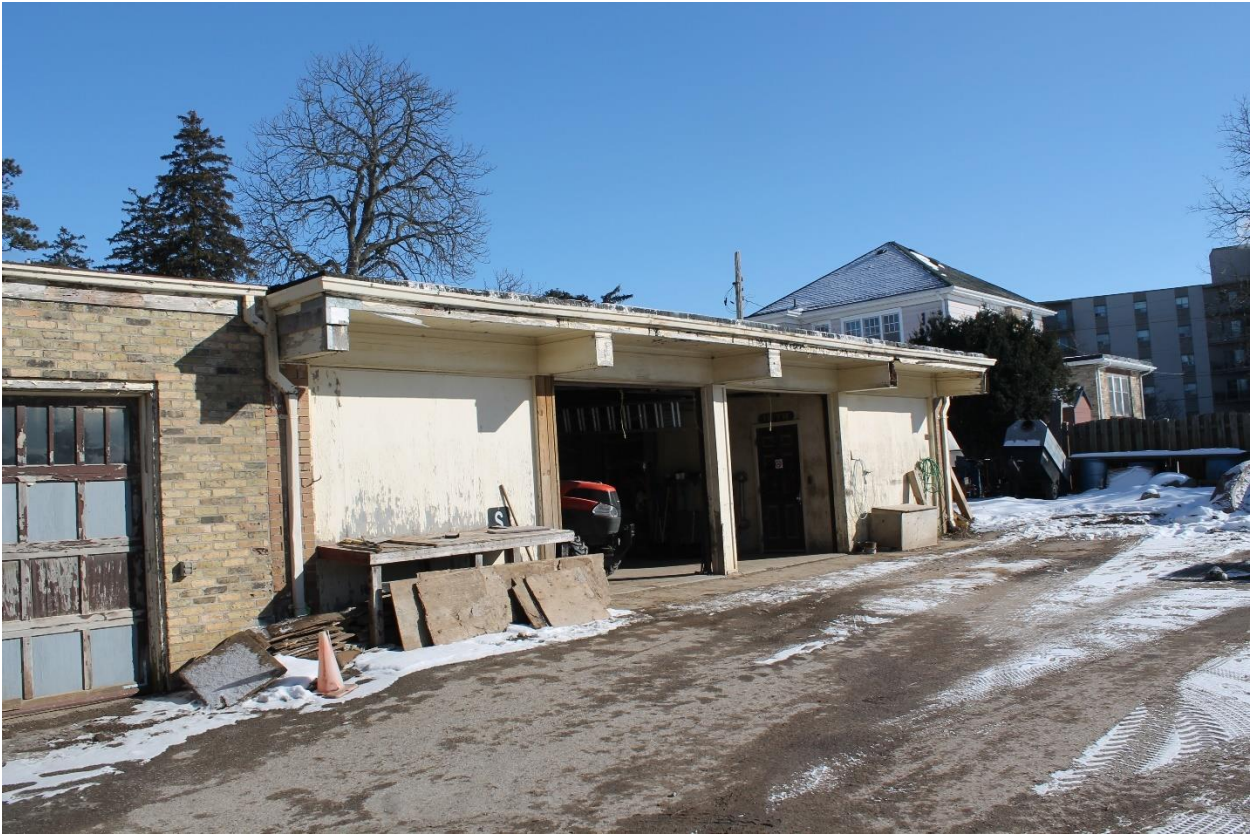
Image 11: Photograph showing the rear elevation of the maintenance garage (2022).
