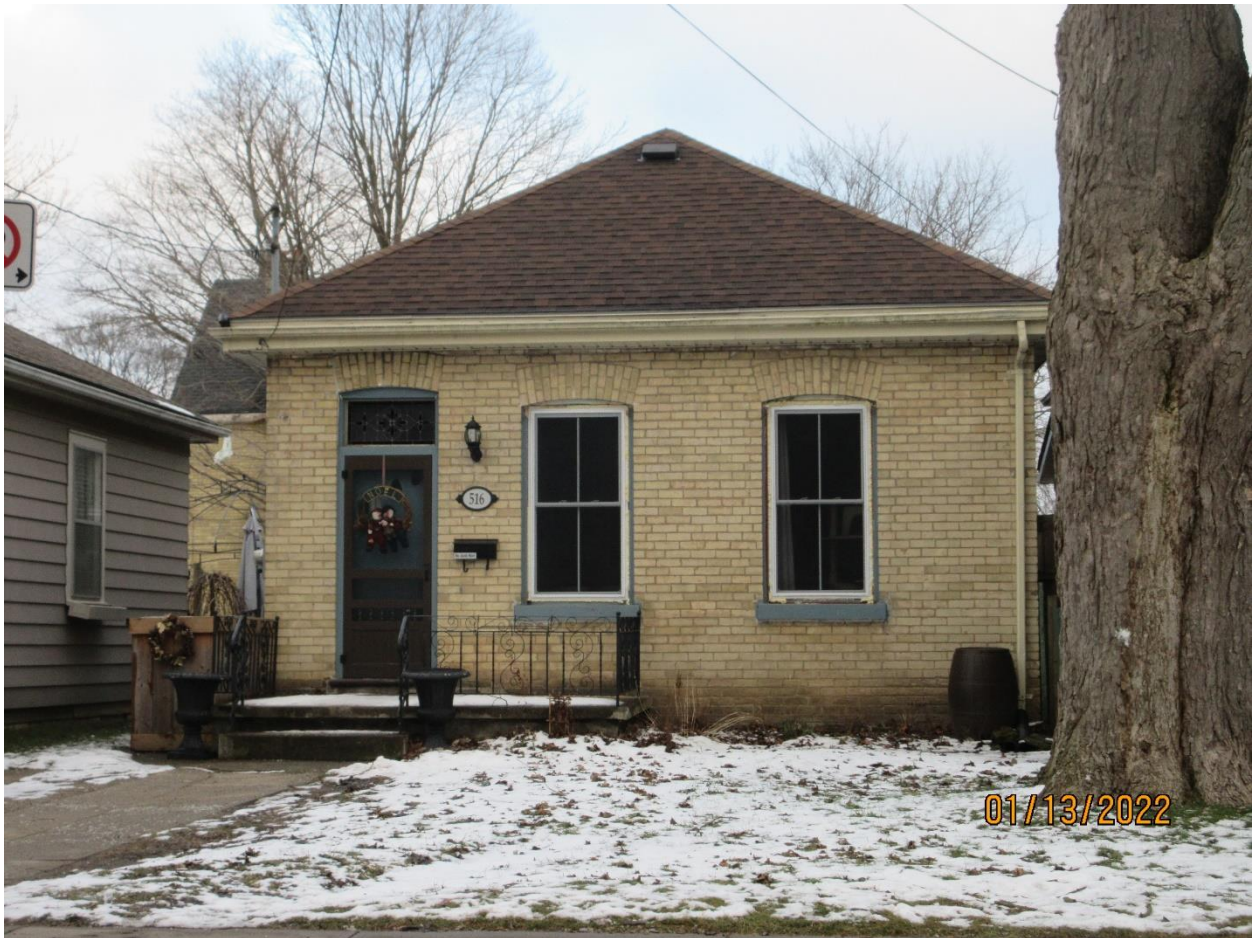
Image 3: Photograph of the house at 516 Elizabeth Street on January 13, 2022. Note the reinstated transom and replacement of the front windows.
