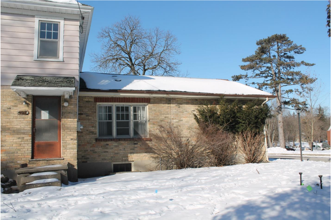
Image 6: South elevation showing front addition and original portion of the former gate house (2022).
