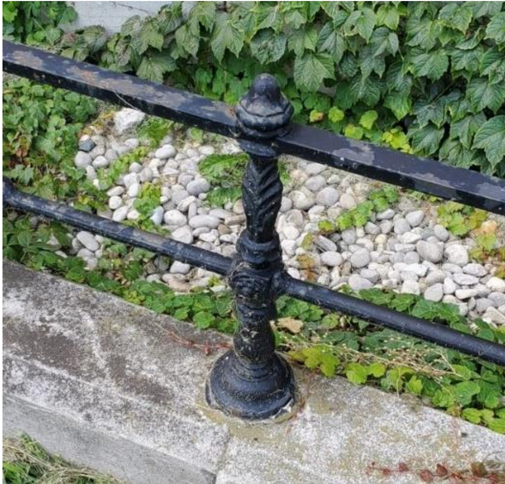
Photograph 37: Example of a vertical rail post with finial with a rounded point (AECOM, July 2021)
