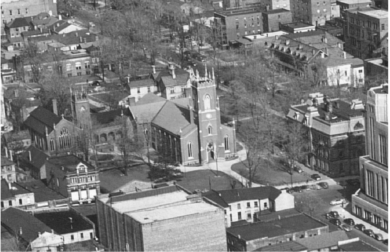
Image 1: Detail of an aerial image, showing St. Paul's Cathedral and the Customs House (Series 5, A1229, 1951-1952).
