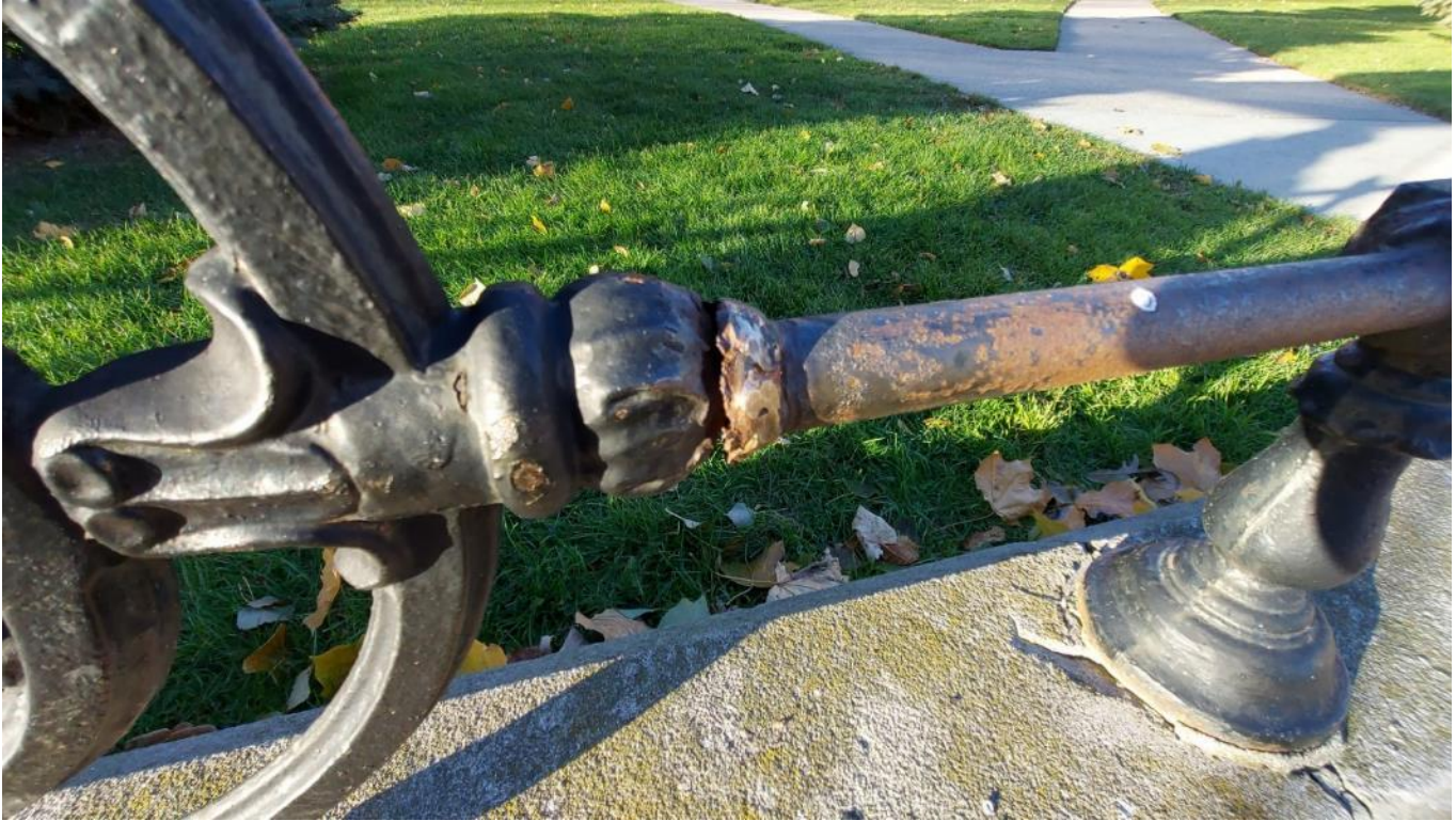
Photograph 31: The mid horizontal rail inserted into the ends of the beaver medallion and into the receiving ends of the vertical posts. The tube is welded at each location (AECOM, November 2021)
