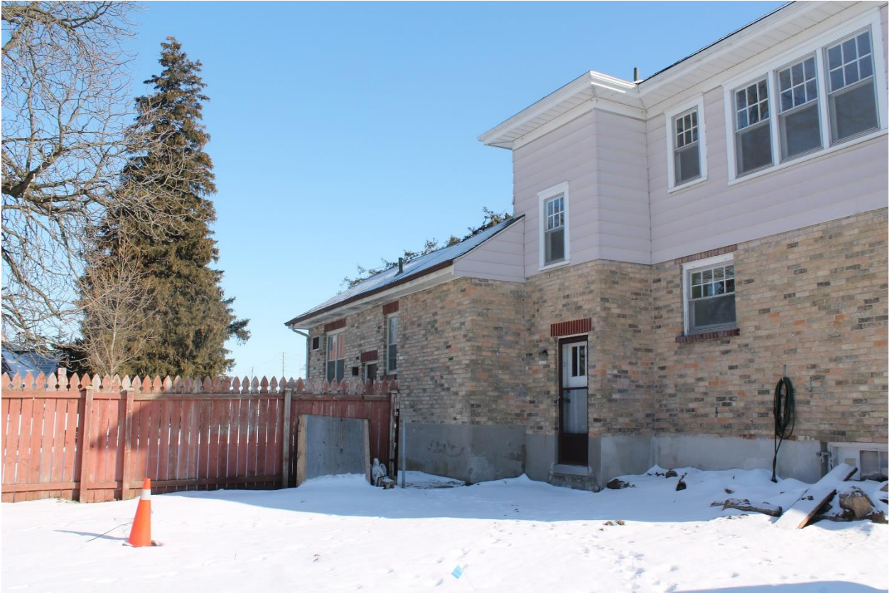
Image 8: Photograph showing north elevation of the former gate house (2022).
