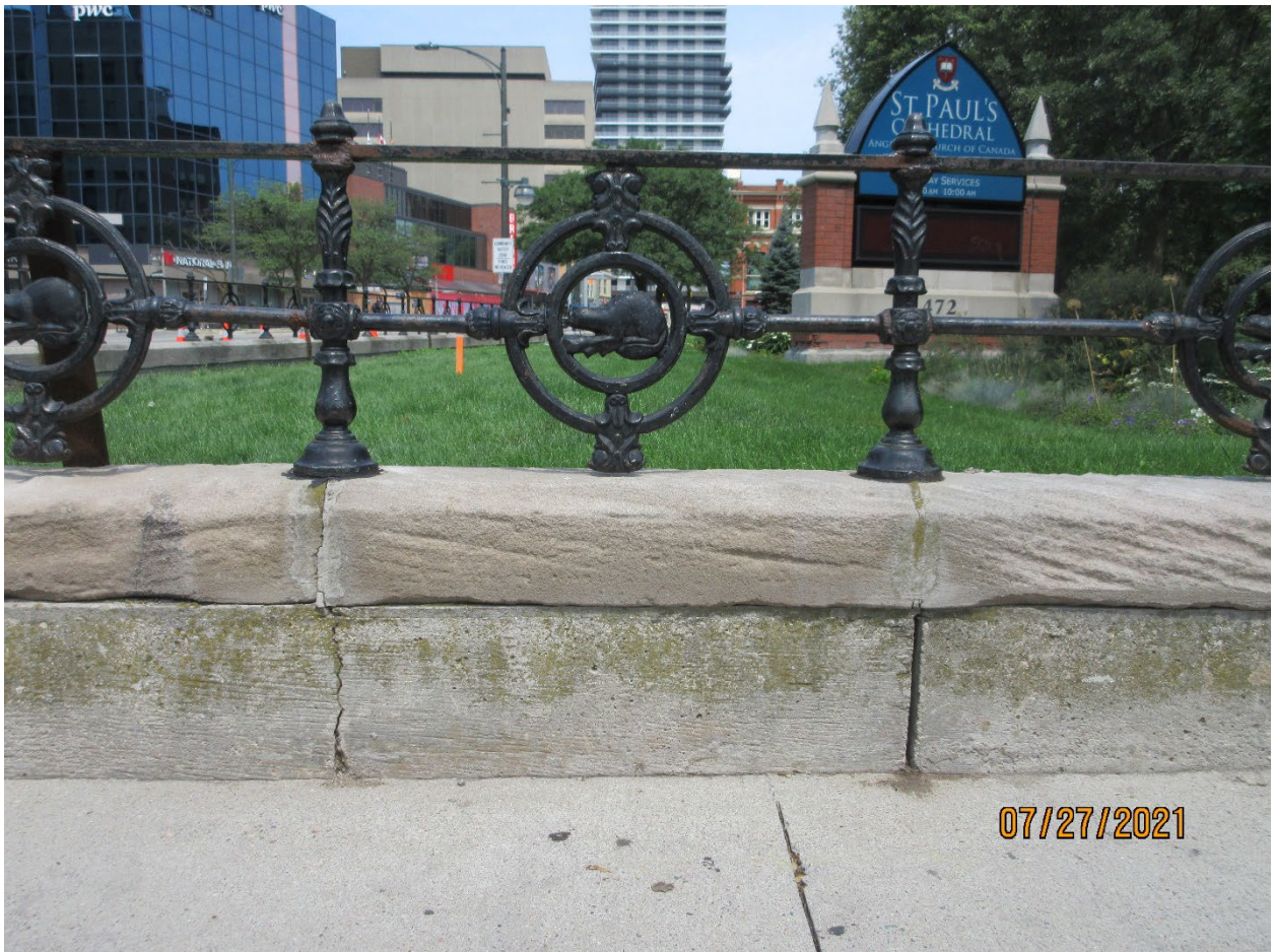
Image 4: Detail view of a typical panel of the beaver fence, composed of its cast iron posts, rails, and medallions, sandstone cap stones, and concrete foundation.
