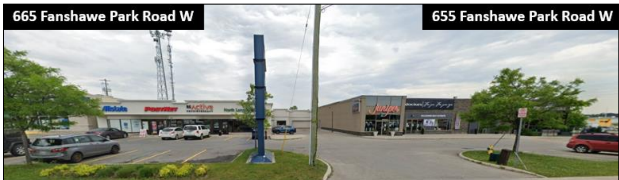
Figure 2: Subject lands and current uses (June 2021) – view from Fanshawe Park Road West, facing northeast
