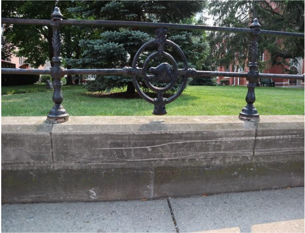
Photograph 12: Sandstone cap stones and concrete foundation of the fence on Richmond Street, south side of the main entrance path (AECOM, July 2021)
