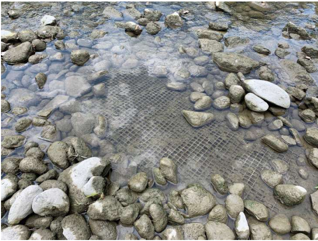
Photo 3: Partially exposed geotextile mat approximately 5 m from the east bank; Date: August 4, 2021.
