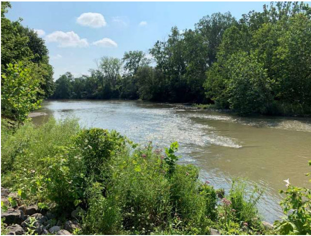
Photo 1: View of the watermain crossing from the east bank; SW aspect; Date: August 4, 2021.
