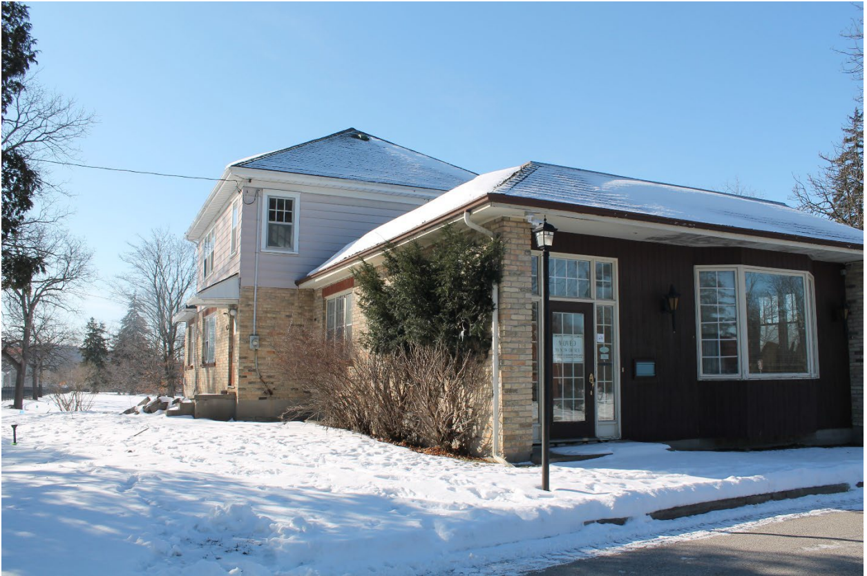
Image 5: East (front) elevation of the former gate house at Woodland Cemetery (2022).
