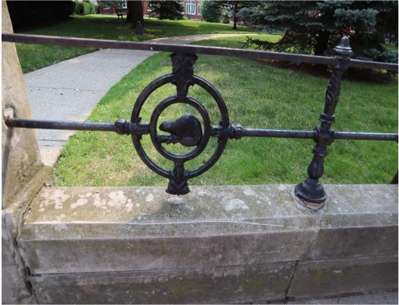
Photograph 11: Details of the cast-iron fence (AECOM, July 2021)
