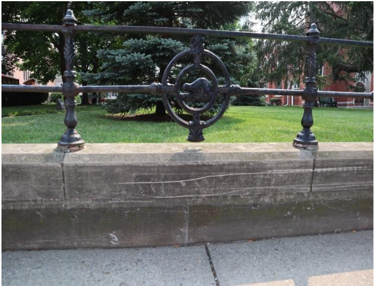
Photograph 12: Sandstone cap stones and concrete foundation of the fence on Richmond Street, south side of the main entrance path (AECOM, July 2021)
