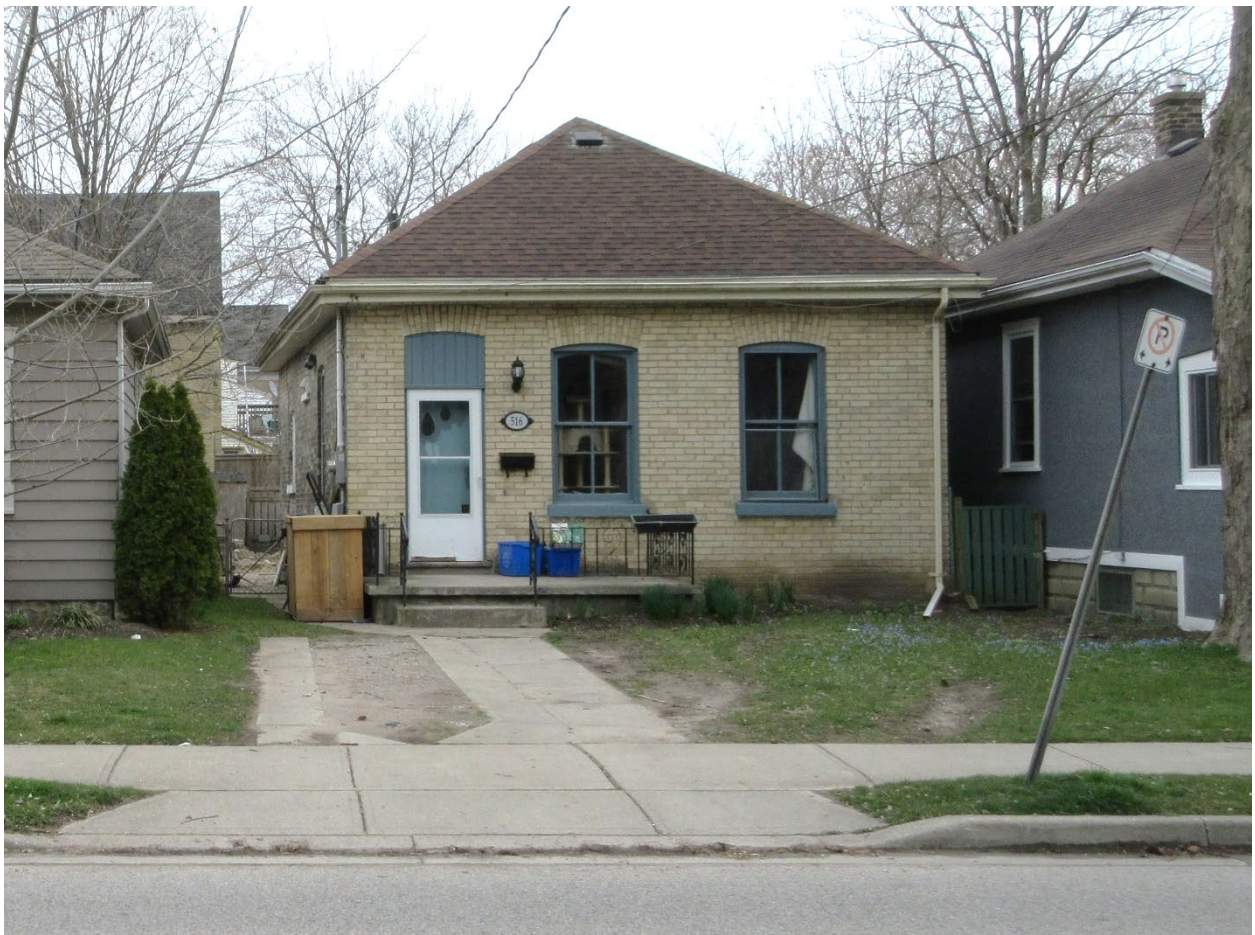
Image 2: Photograph of the house at 516 Elizabeth Street on April 24, 2020. Note the painted wood, two-over-two wood windows.
