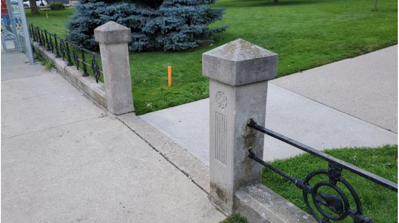
Photograph 14: The most western end posts on Queens Avenue proposed for relocation (AECOM, May 2021)
