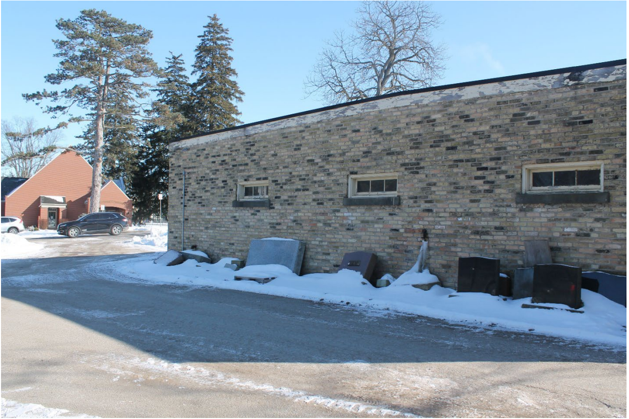
Image 10: Photograph showing the side elevation of the maintenance garage and the new administrative office at left (2022).
