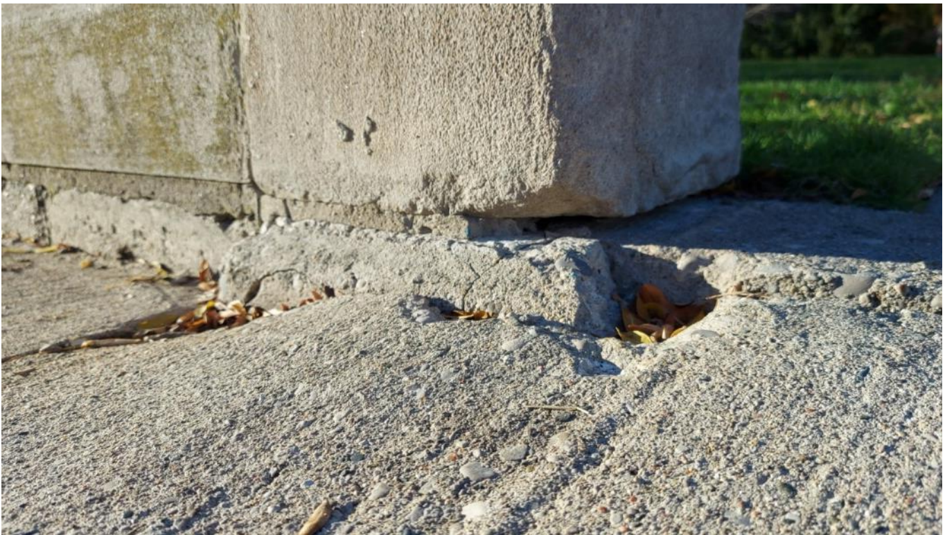
Photograph 17: End post placed on a mortar layer with a concrete foundation (AECOM, November 2021)
