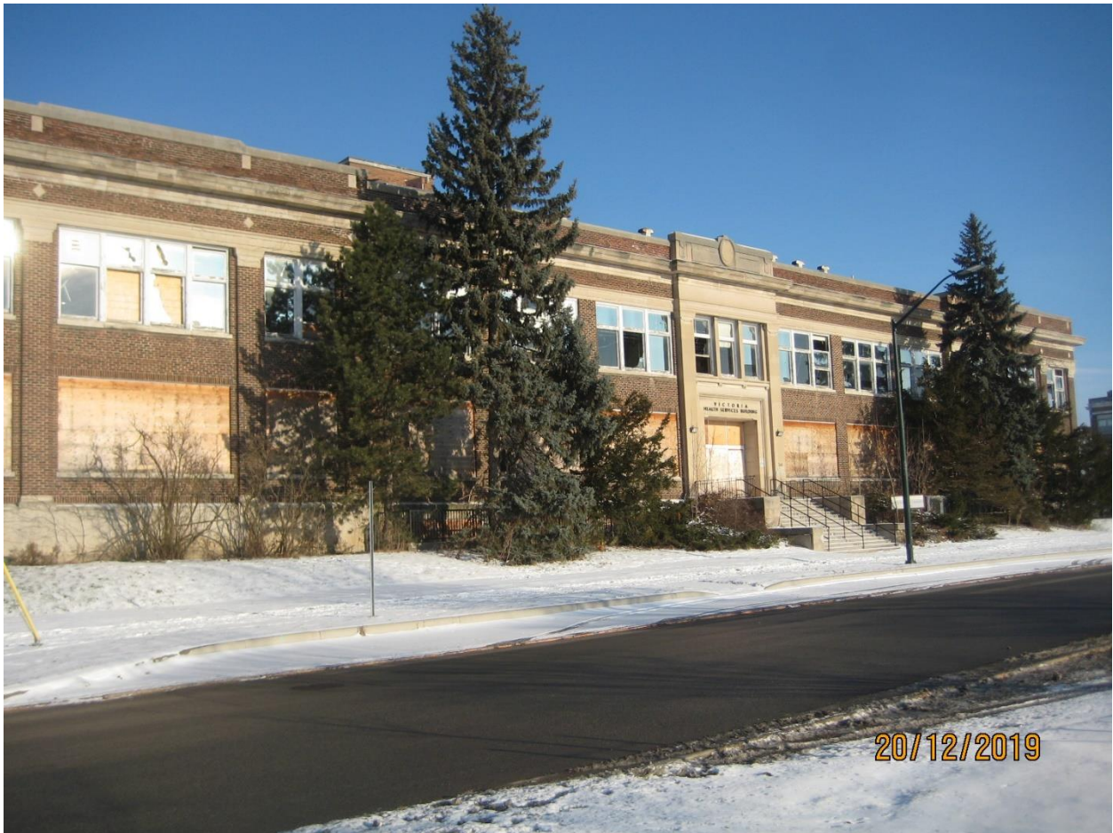
Image 1: Photograph showing the south façade of the Health Services Building located on the Old Victoria Hospital Lands.
