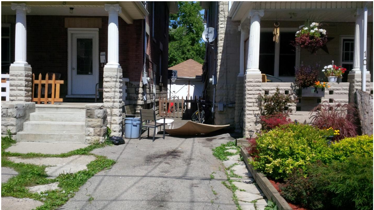
Image 1: Photograph of the dwelling at 10 Bruce Street (right) and the adjacent 8 Bruce Street (left) submitted as a part of the Heritage Alteration Permit application. Note, the concrete plinths and columns on each property are similar, but the railing systems are different.
