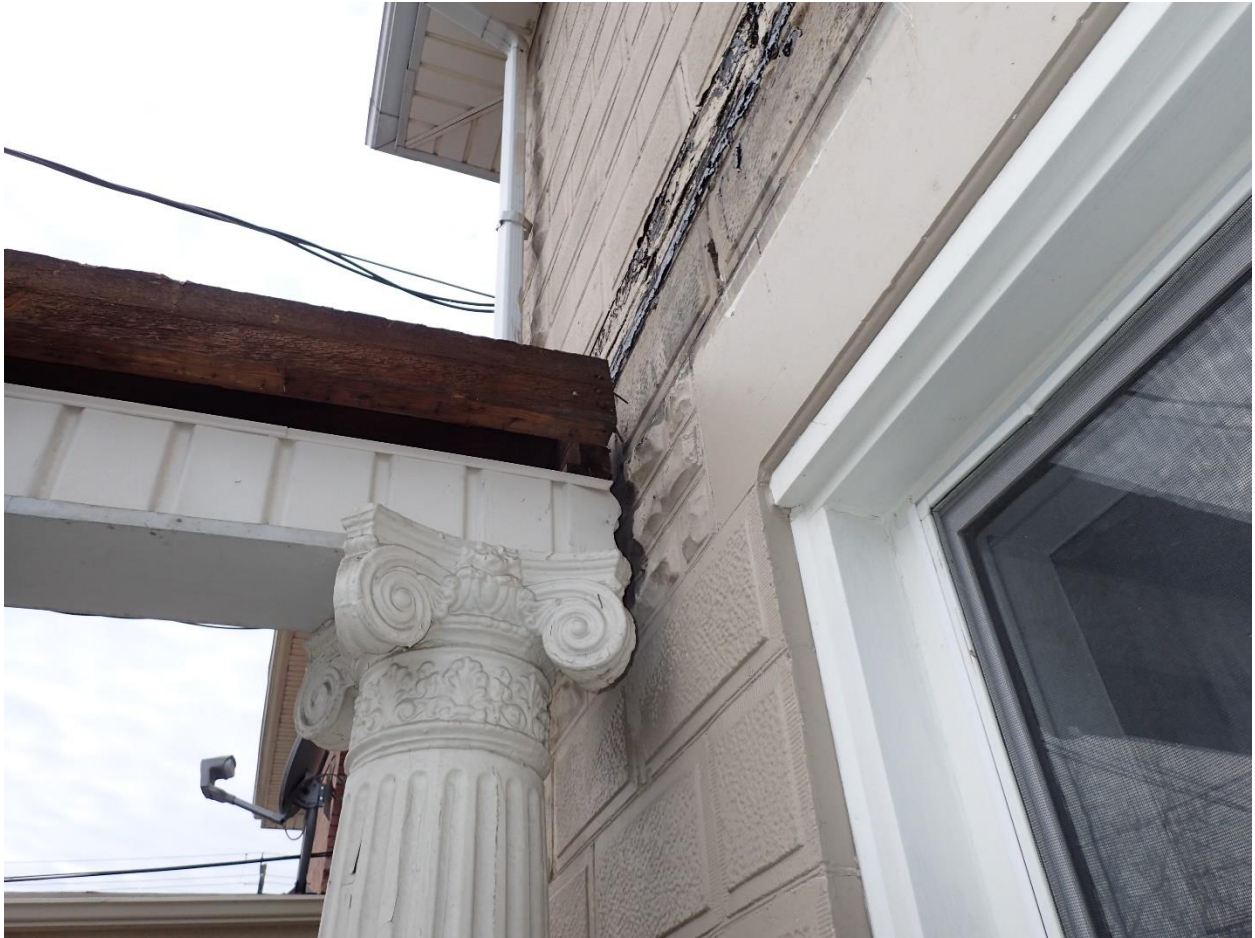
Image 3: Detail showing the previous decorative columns on the porch at 10 Bruce Street. The details of the columns are to be replicated for the new porch.
