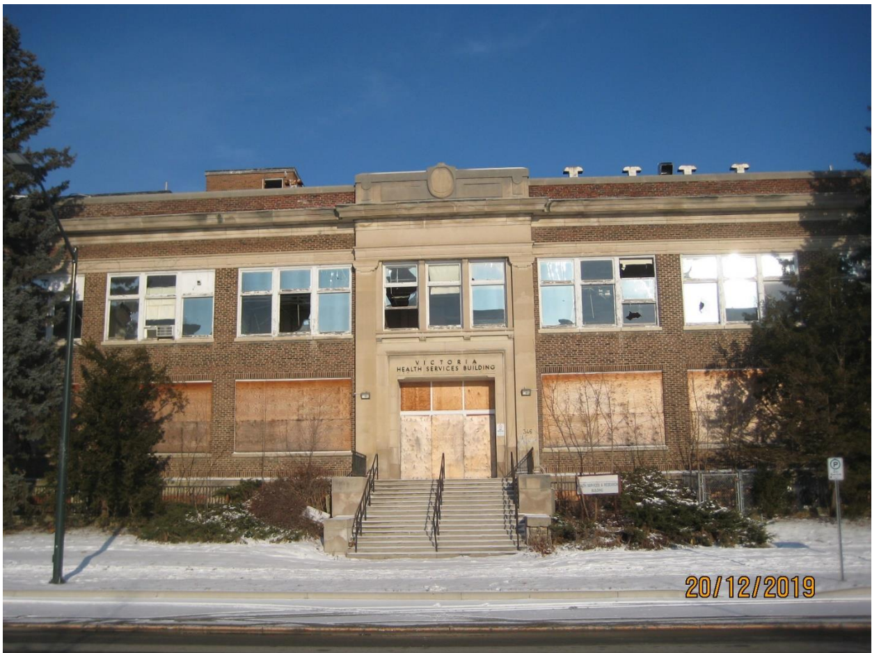
Image 2: Photograph showing the south façade of the Health Services Building located on the Old Victoria Hospital Lands.
