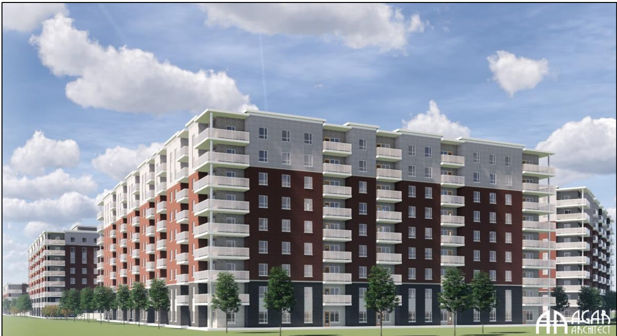
Figure 10 – Looking south onto the rear of the subject site
