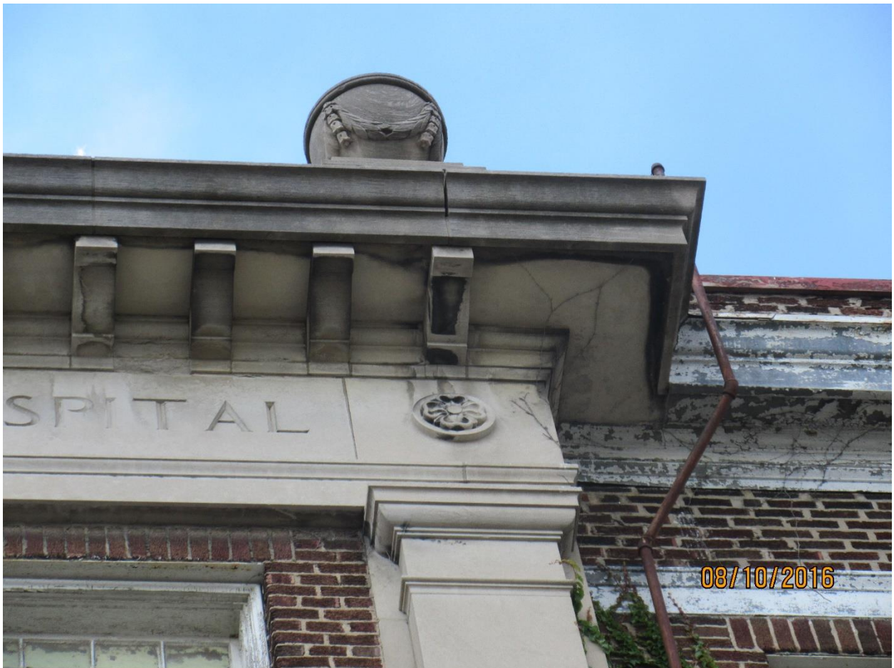
Image 14: Detail showing cornice and bracket detailing on the War Memorial Children's Hospital.
