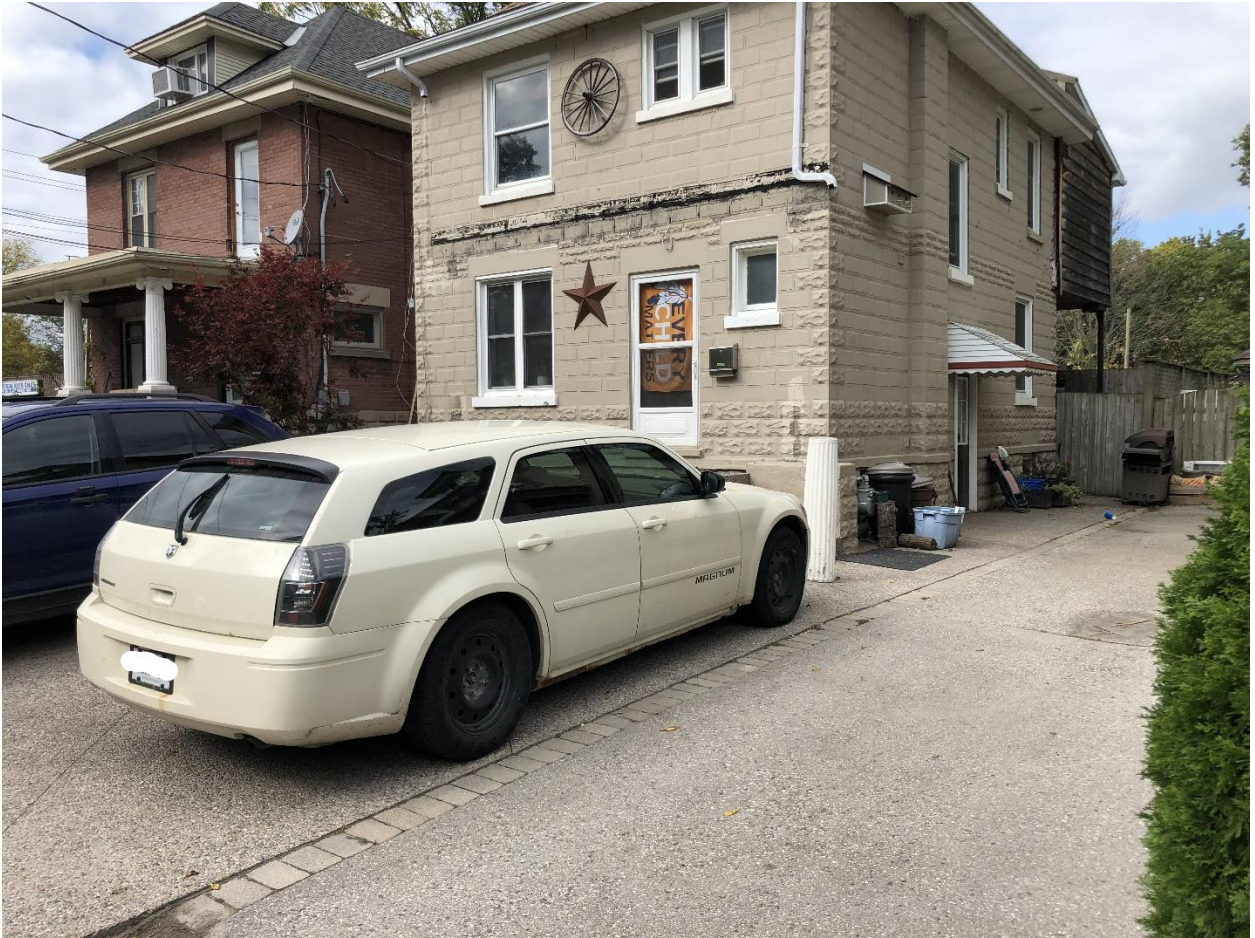
Image 5: Photograph showing the dwelling located at 10 Bruce Street following the removal of the previous porch, October 2021.
