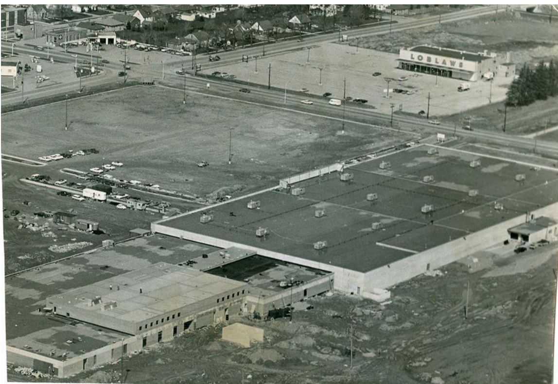
Figure 20: Aerial photograph showing the completion of the Argyle Mall in 1966. The Clarke House can be seen along the very top edge of the photograph. Courtesy London Free Press Negatives Collection, Western Archives and Special Collections.
