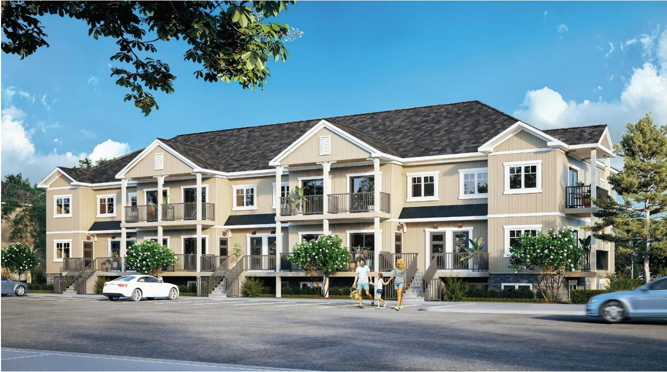
Looking at the face of one building from Maitland Street.
