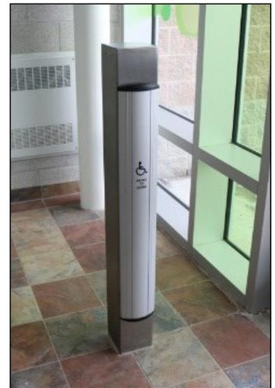
Example of large vertical extended power door operator control.
