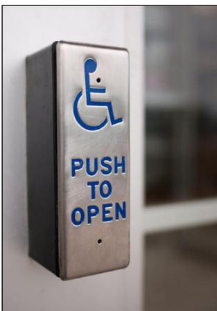
Example of rectangular shaped power door operator control to be used for retrofit situations only, where infeasible to provide larger controls.
