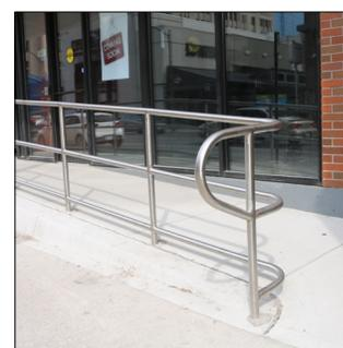
Ensure handrail extensions do not obstruct path of travel or create hazards.
