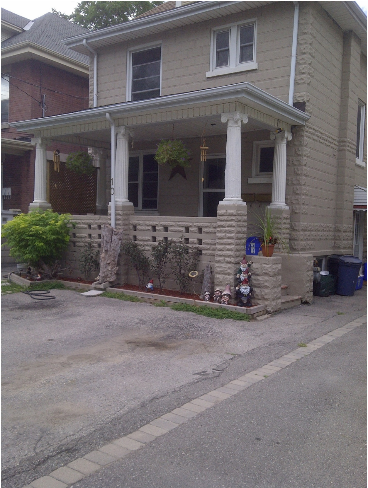
Image 2: Photograph submitted with the Heritage Alteration Permit application showing the previous appearance of the porch. The proposed alterations are to reconstruct the porch to replicate its previous design.
