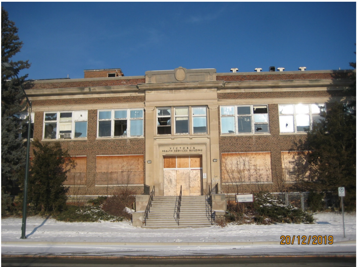
Image 2: Photograph showing the south façade of the Health Services Building located on the Old Victoria Hospital Lands.
