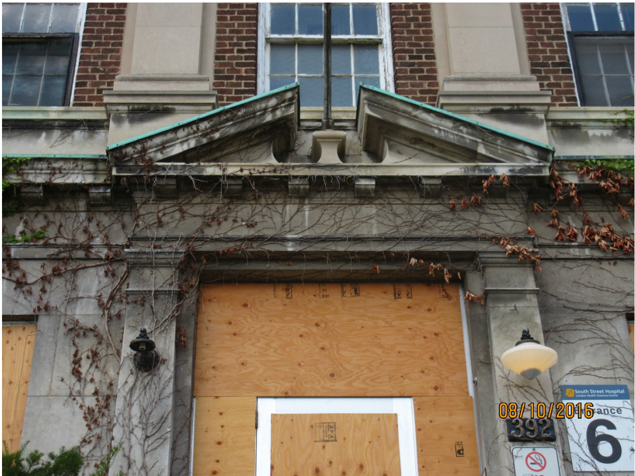
Image 12: Detail showing pediment and stone frontispiece detailing on the War Memorial Children's Hospital.
