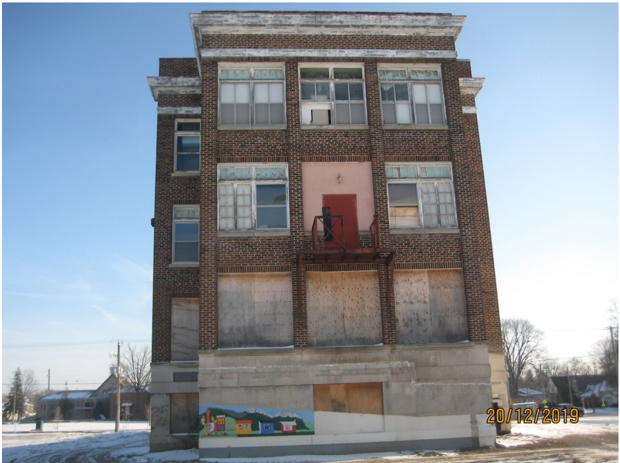
Image 10: Photograph showing the west facade of the War Memorial Children's Hospital.
