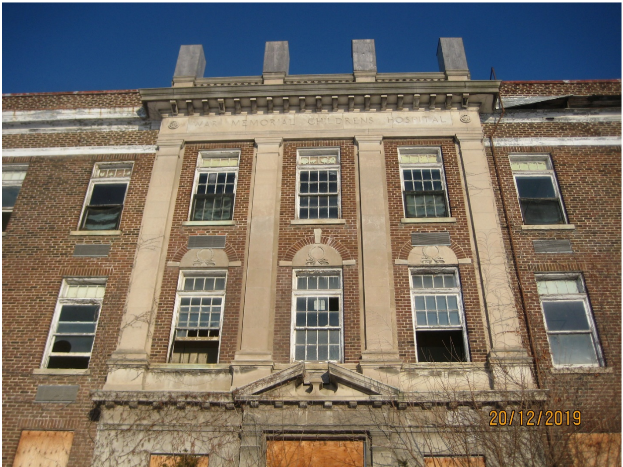
Image 8: Photograph showing the frontispiece and detailing on the War Memorial Children's Hospital.
