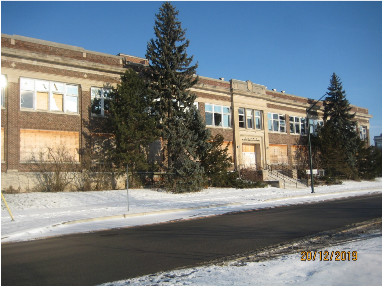
Image 1: Photograph showing the south façade of the Health Services Building located on the Old Victoria Hospital Lands.
