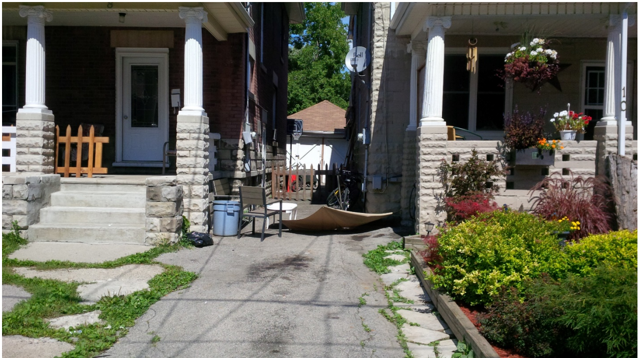
Image 1: Photograph of the dwelling at 10 Bruce Street (right) and the adjacent 8 Bruce Street (left) submitted as a part of the Heritage Alteration Permit application. Note, the concrete plinths and columns on each property are similar, but the railing systems are different.
