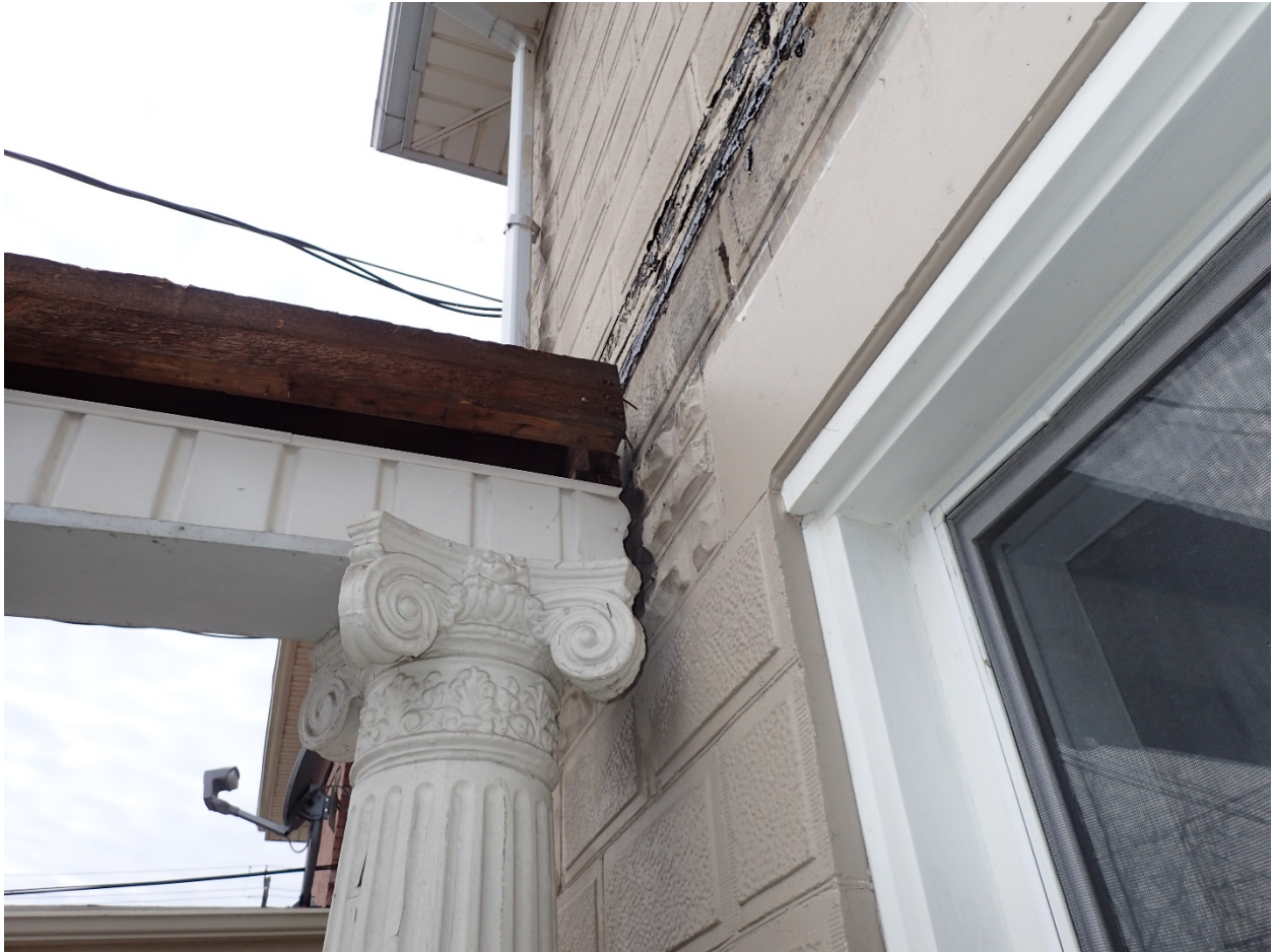
Image 3: Detail showing the previous decorative columns on the porch at 10 Bruce Street. The details of the columns are to be replicated for the new porch.
