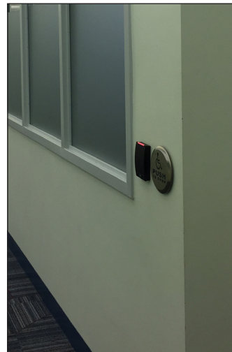
Example of proximity card reader system with high colour / tonal contrast compared to mounting surface for enhanced visibility, City of London.
