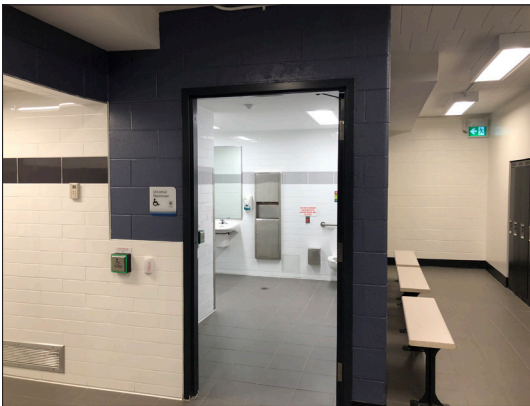
Example of a universal washroom integrated as part of an accessible change room, City of London.
