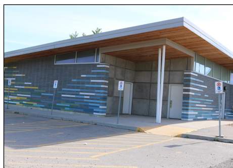
Accessible parking spaces with shared access aisle connected to pedestrian route.
