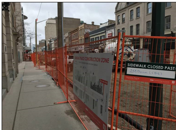
Example of typical construction fencing, City of London.
