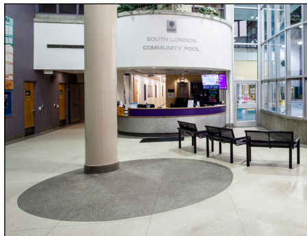
Where a structural column / support may be within an accessible route, a colour contrasted floor surface at the base helps identify its location to prevent a potential bumping hazard.
