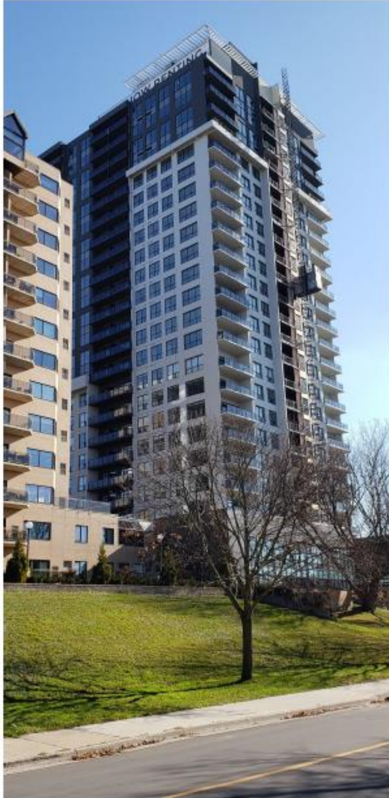
320 Thames Street, across from Ivey Park.
