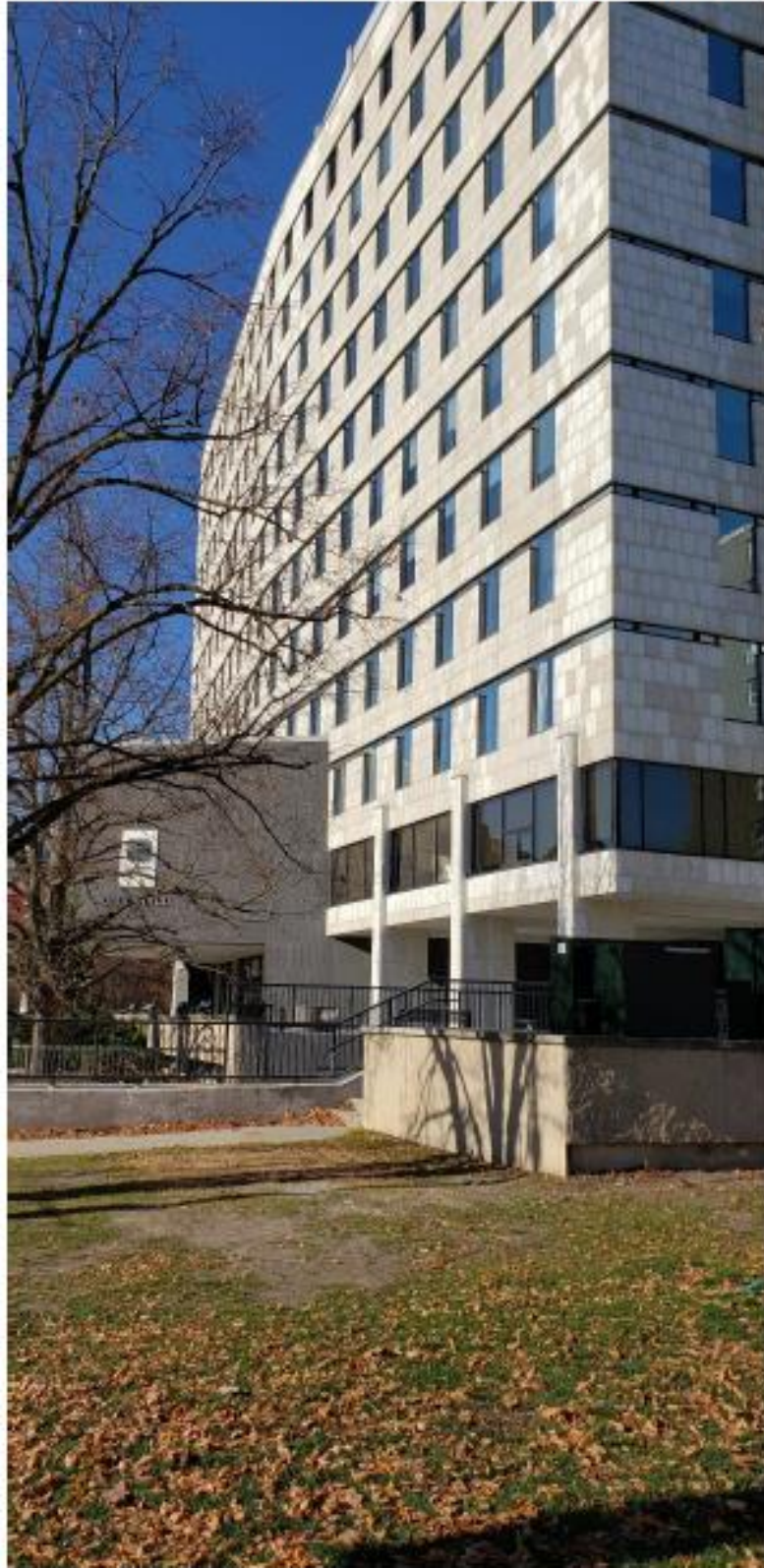
300 Dufferin, 11-storey City Hall, across from and overlooks Victoria Park
