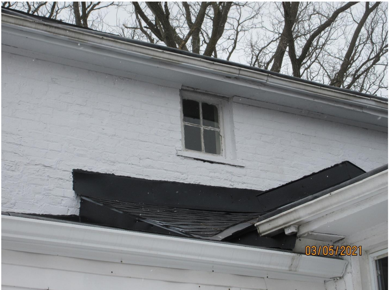
Image 8: The small, four-lite window on the north elevation, under the eaves, in the second storey of the Clarke House.
