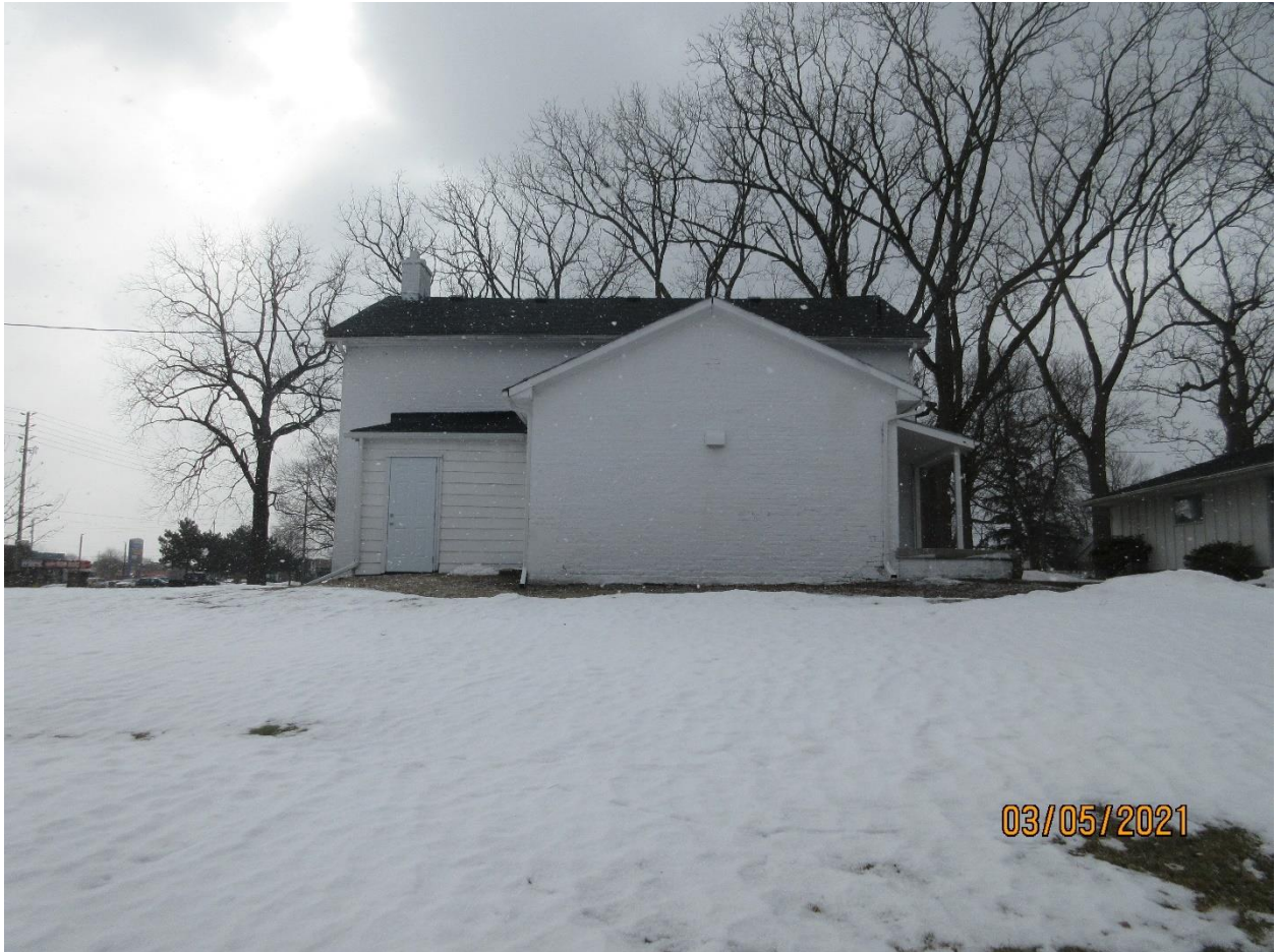
Image 9: View of the rear (north) elevation, as seen from Avalon Street.
