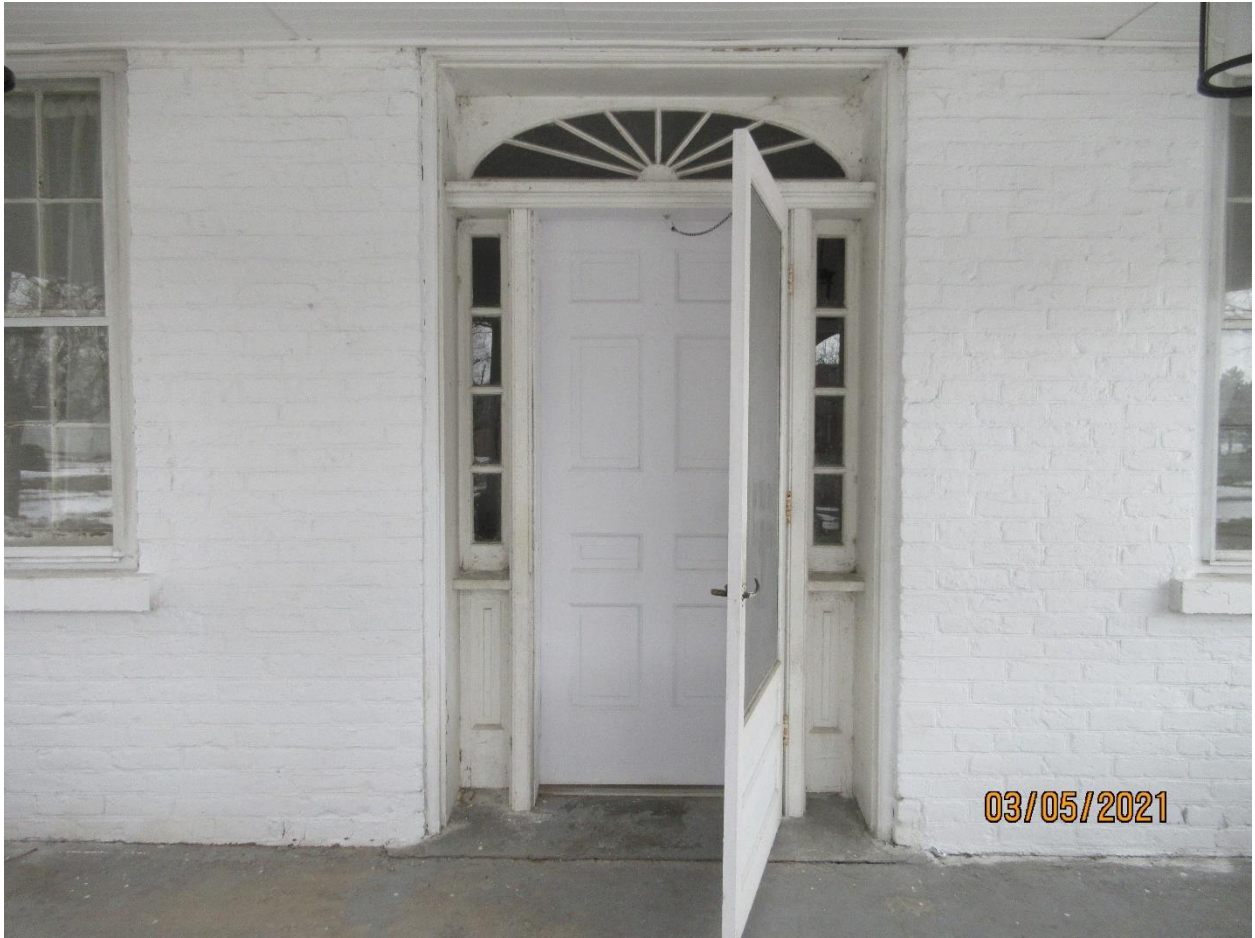
Image 15: Detail of the front doorway of the Clarke House.
