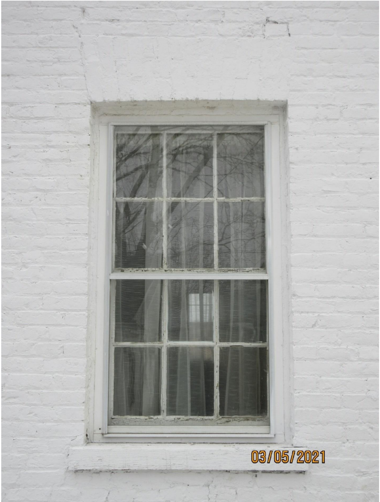
Image 17: Representative image of the six-over-six wood windows on the ground storey and gable ends of the Clarke House. The dormer windows closely resemble these windows.
