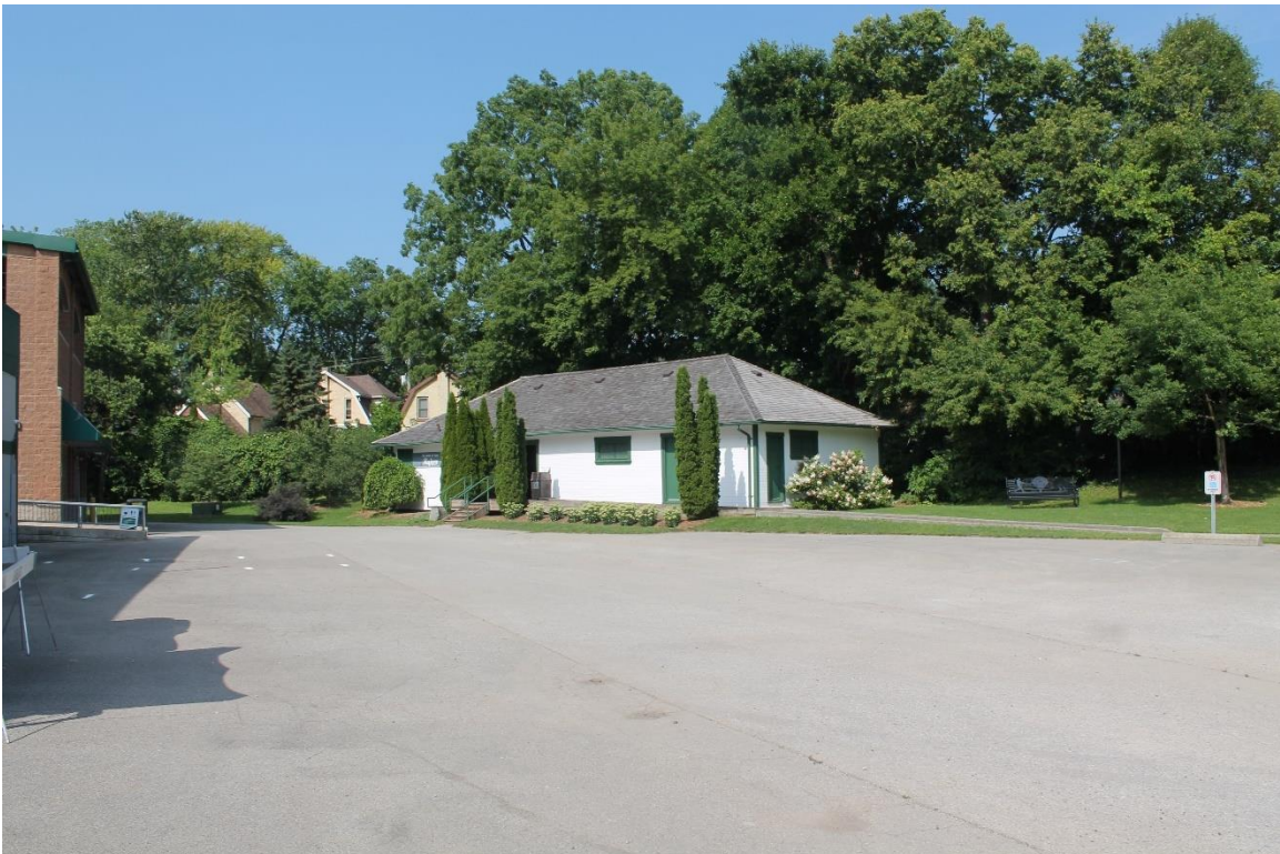
Image 10: Photograph showing the Roy McKay Clubhouse, constructed in 1937, located behind the grandstands along the third baseline.
