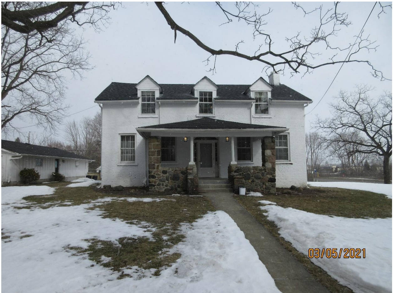
Image 4: View of the main (south) façade of Clarke House. The detached garage is shown on the left.
