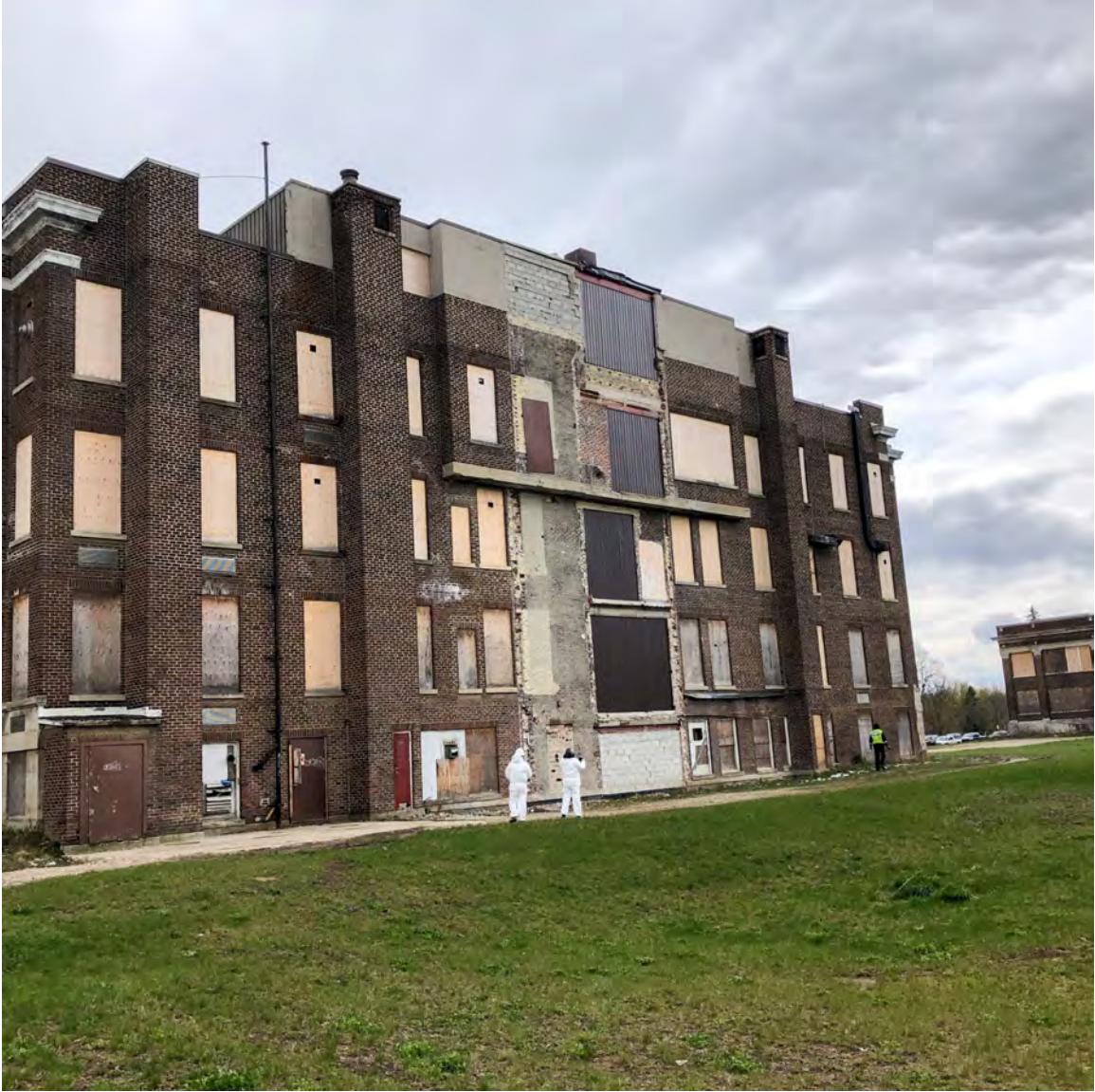
REAR ELEVATION – the Health Sciences Building is visible on the right side of the photo
