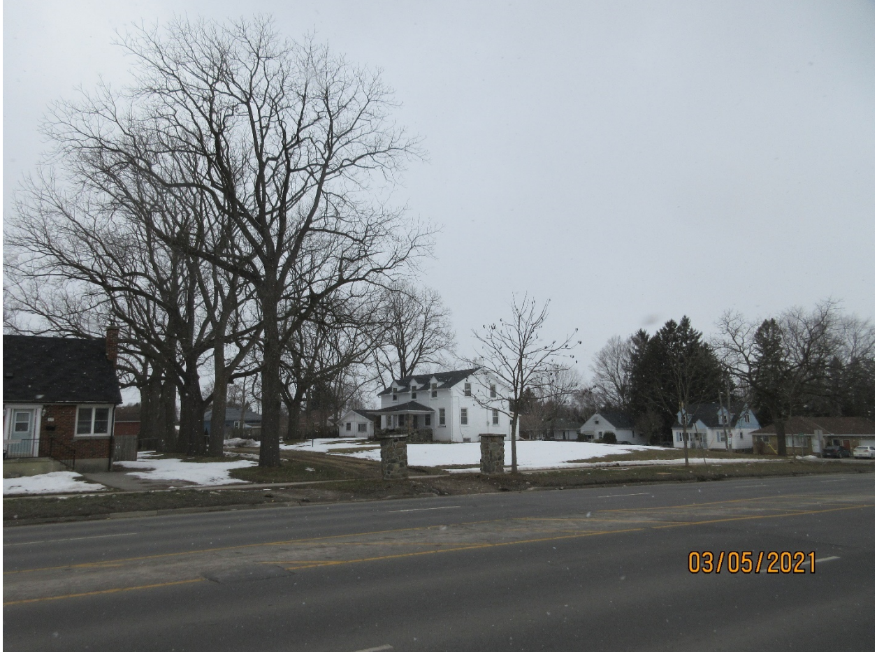
Image 1: Clarke House, as seen from the east side of Clarke Road looking northwest towards the property at 1903 Avalon Street (Clarke House).
