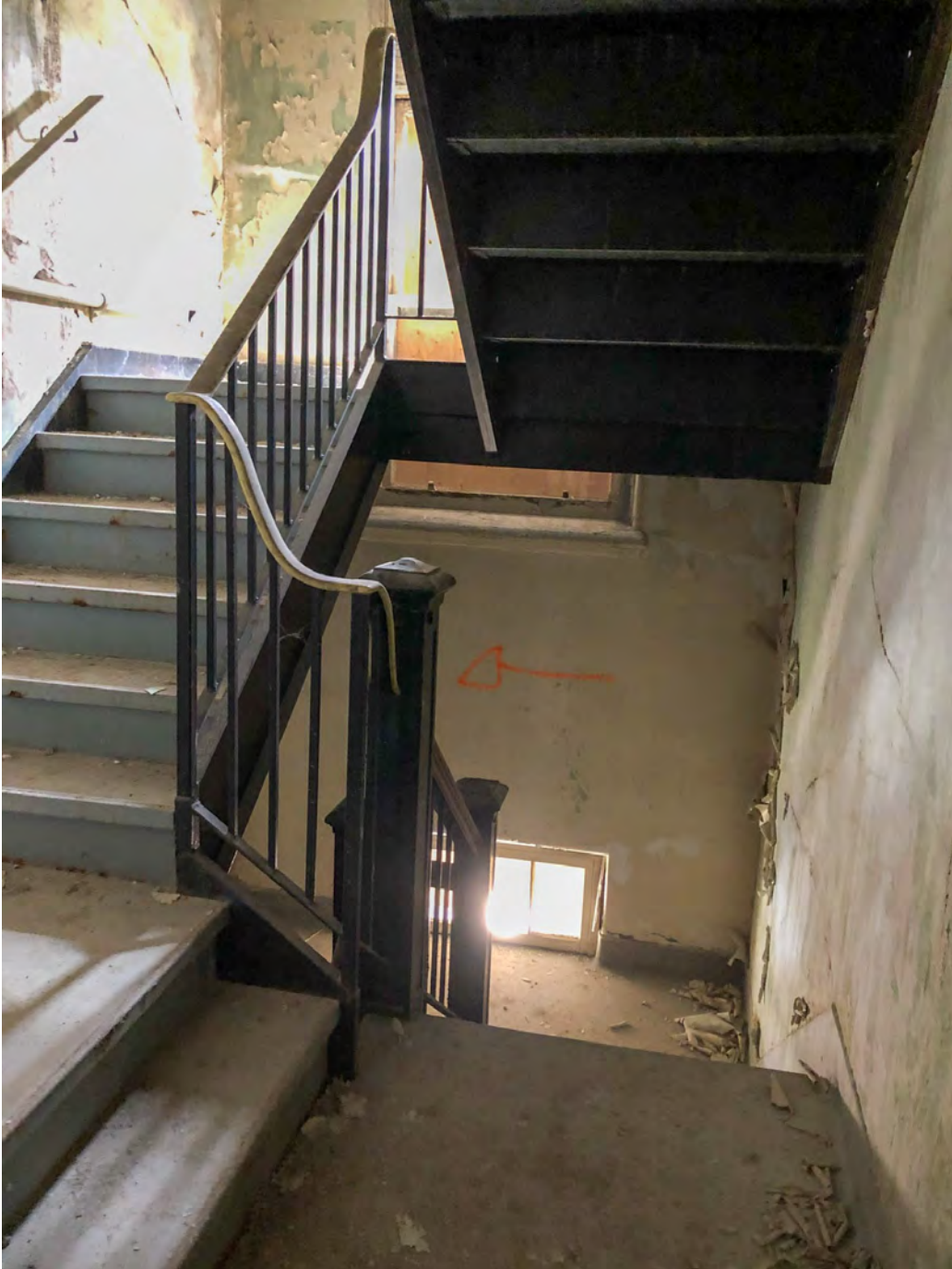
STAIRWELLS – the steel stairs with wooden handrails are in fair condition
