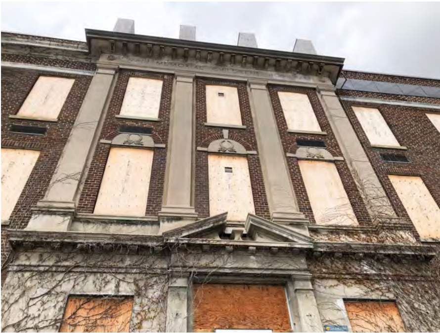
MAIN ELEVATION - Classical detailing
