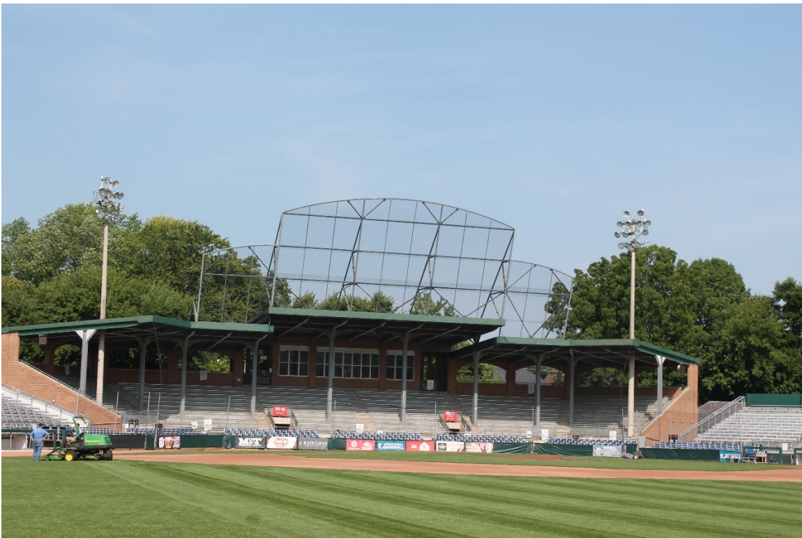
Image 2: Detail looking west from the outfield showing the infield and grandstand.
