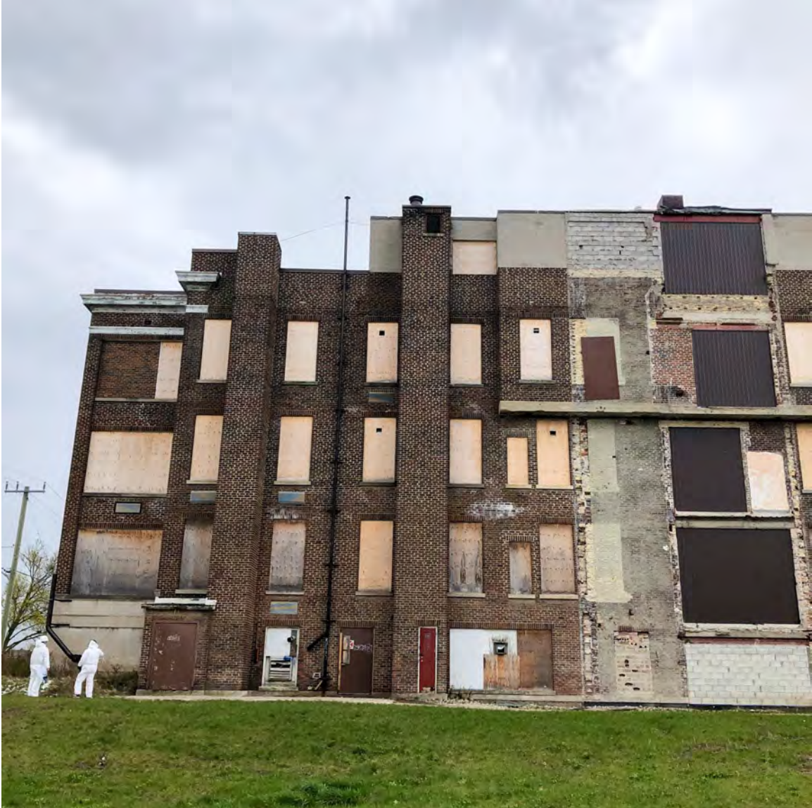
REAR ELEVATION – rear additions have been demolished
