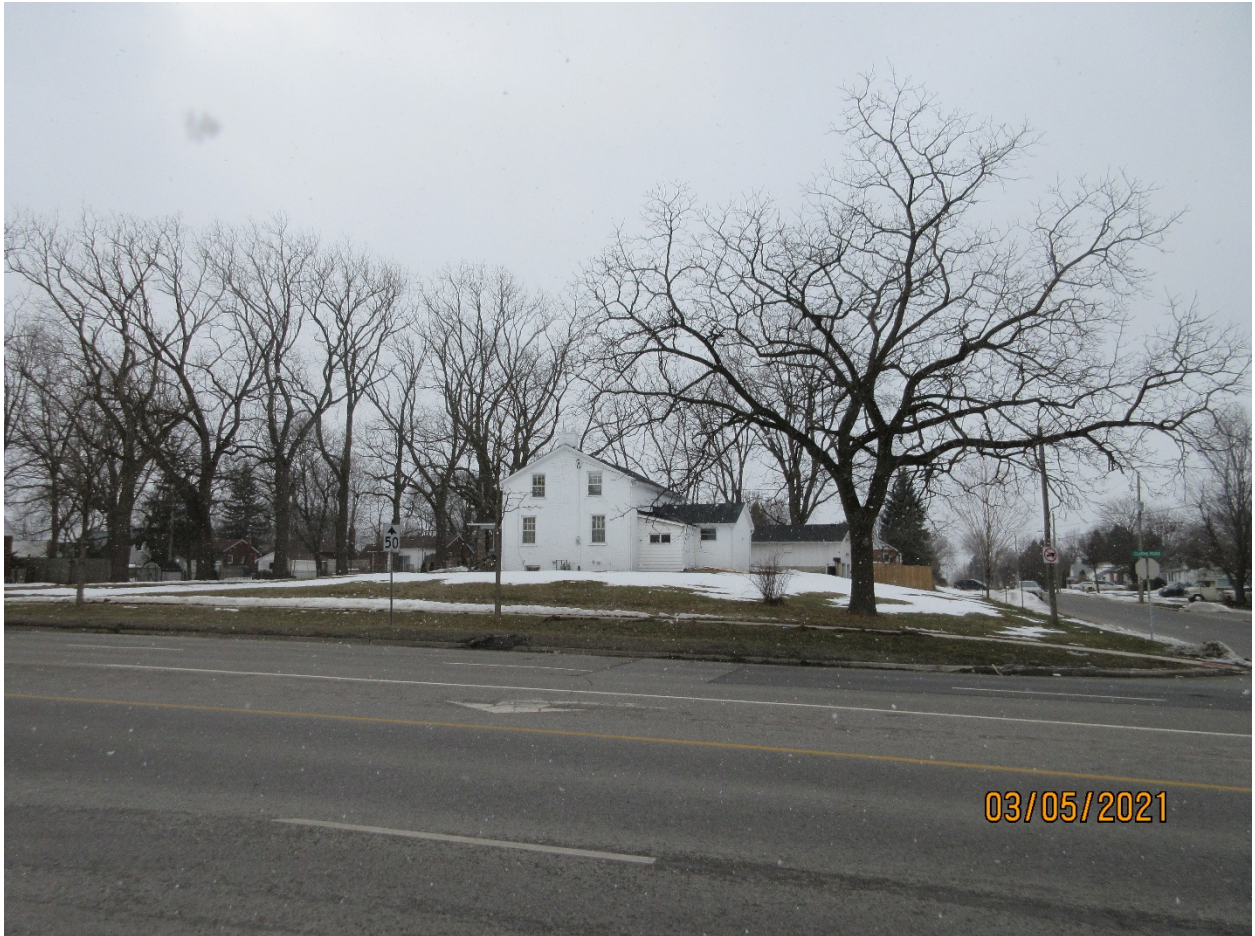
Image 3: View of the Clarke House from the east side of Clarke Road, with the intersection of Avalon Street shown.
