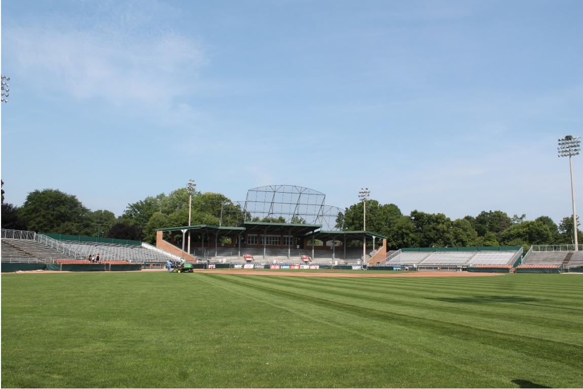
Image 1: Photograph looking west from the outfield towards the grandstands at Labatt Memorial Park.
