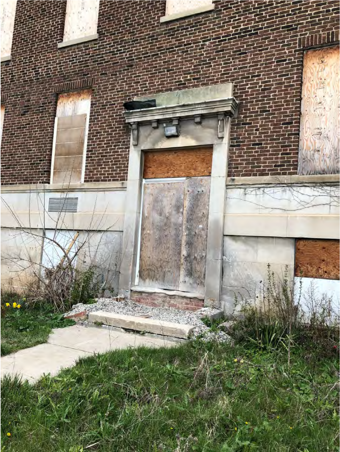
MAIN ELEVATION - SECONDARY ENTRANCE
