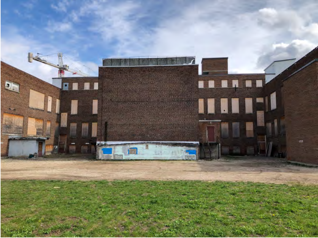
REAR ELEVATION - AUDITORIUM
