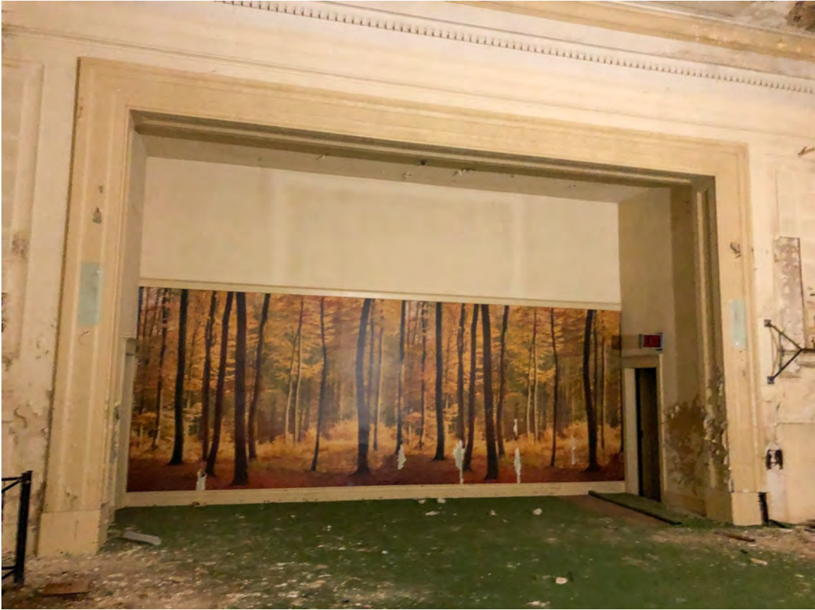
AUDITORIUM – proscenium arch
