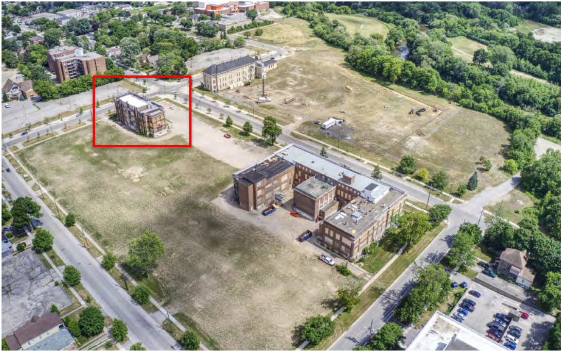
AERIAL VIEW – REAR ELEVATION
