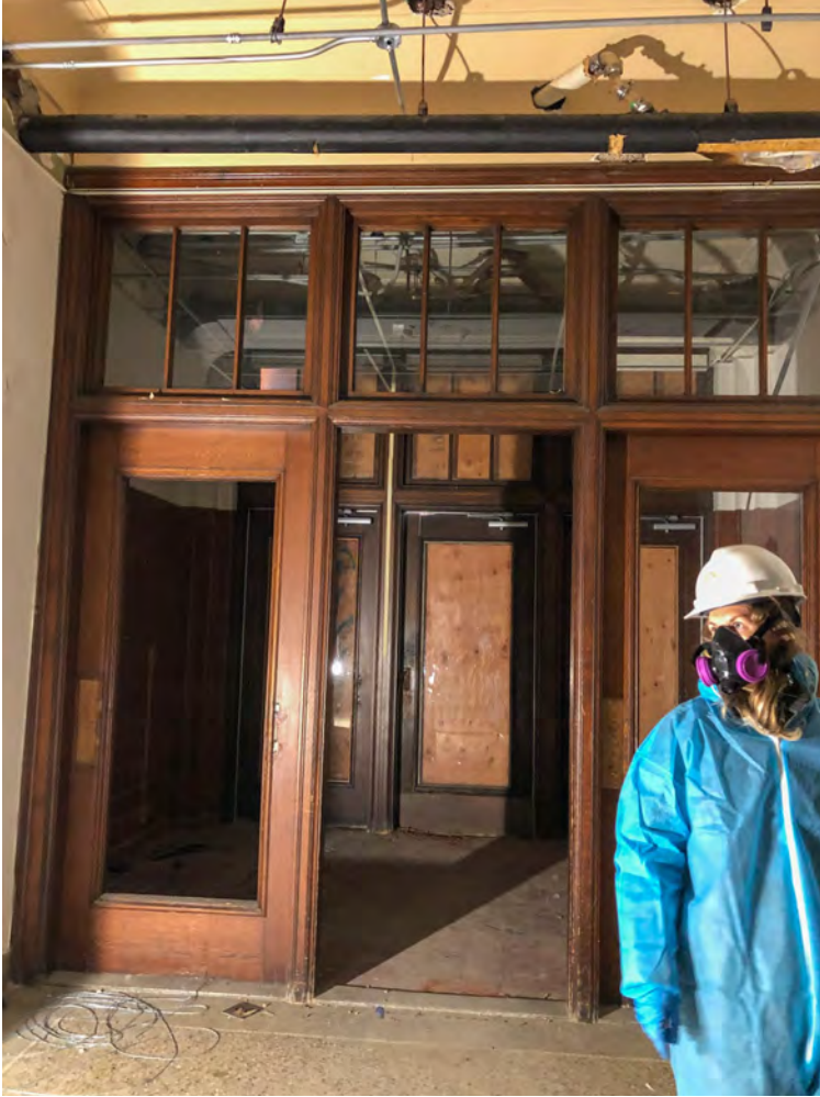
ENTRANCE VESTIBULE - DOUBLE SET OF WOOD DOORS WITH GLAZED TRANSOMS
