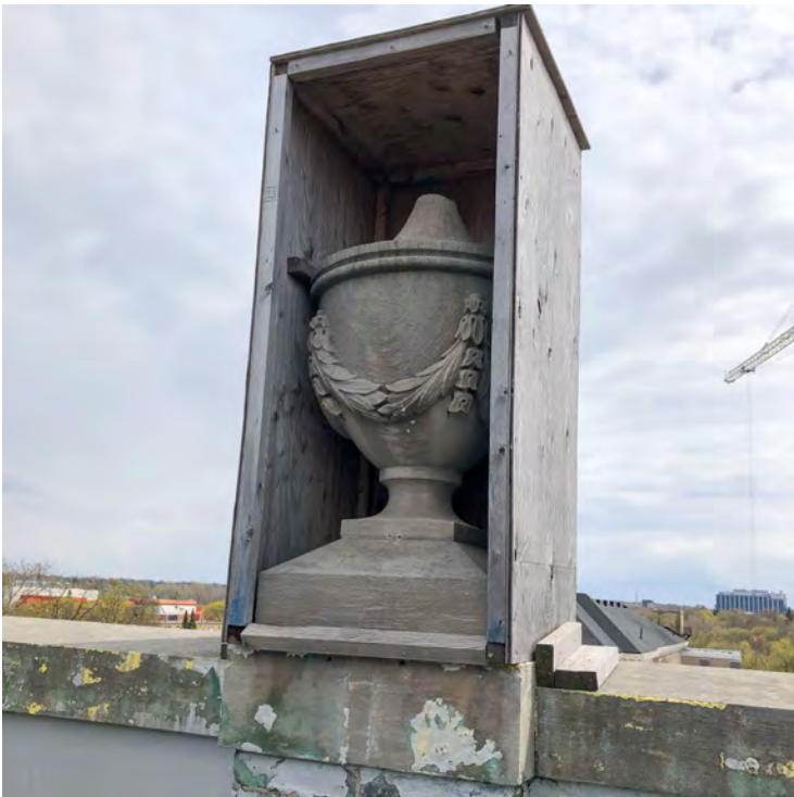
MAIN ELEVATION – classical urn on the roof
