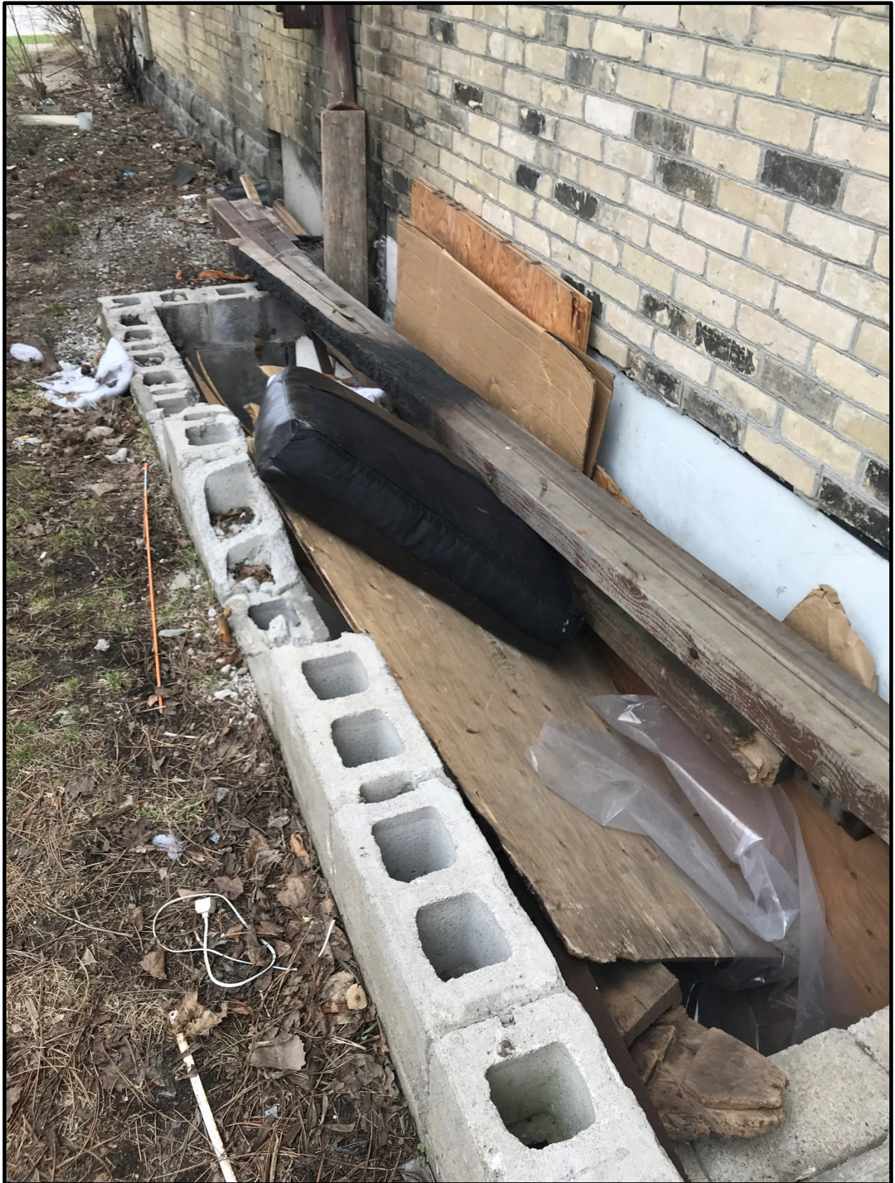
Photo 4 – 72 Wellington St – south side of building (facing river and bike path)
