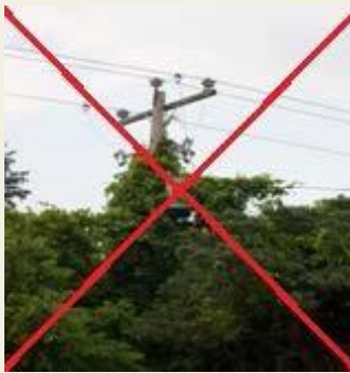
Overgrown vines around electrical equipment
