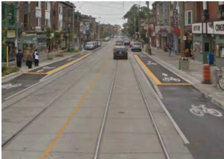
Figure 5.20 – Cycle Facility at Transit Stop (Roncesvalles Avenue, Toronto)
