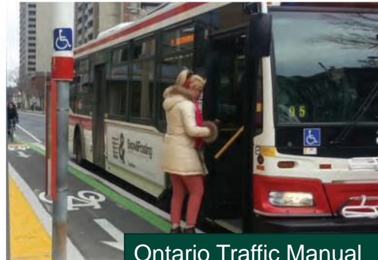
Figure 5.21 – Cycle Facility at Transit Stop (Sherbourne Street, Toronto)
