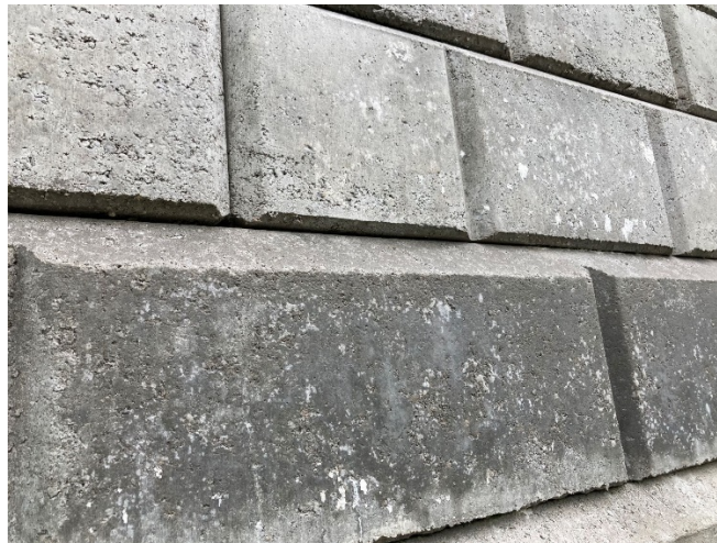
Figure 2: Phase 3 anti-graffiti coating
