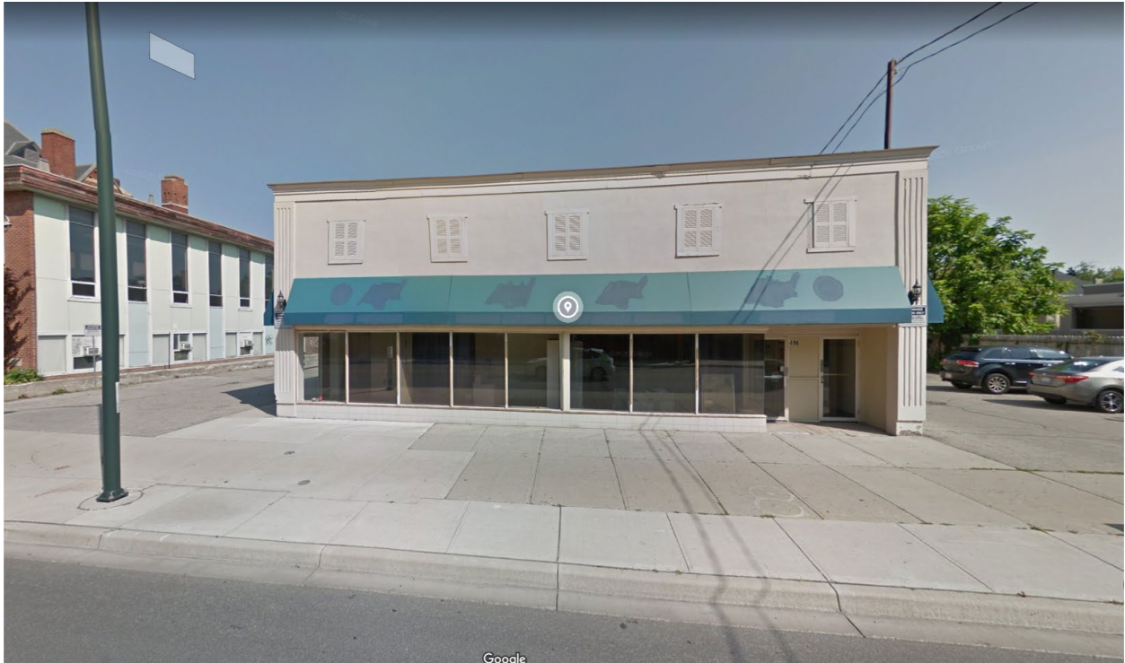
Figure 1: Structure at 496 Dundas Street, facing north.
