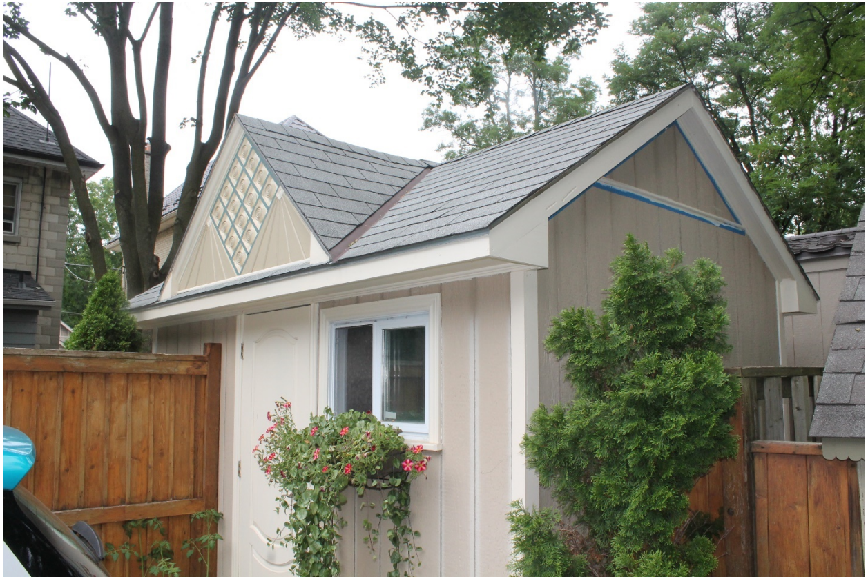
Image 16: Photograph showing rear outbuilding with decorative gable detailing, similar to that found on the projecting gable and porch of the dwelling.
