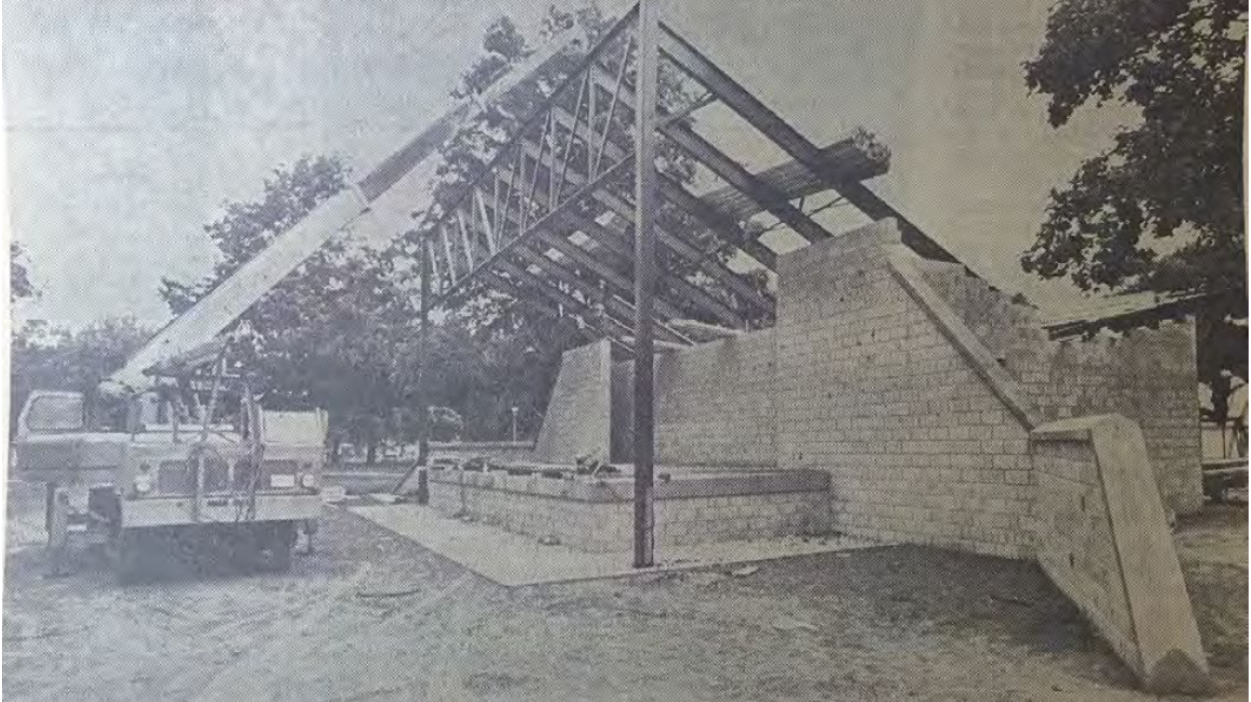
Image 1: Photograph showing the construction of the park stage at Queen's Park, as shown in the London Free Press, September 3, 1971.
