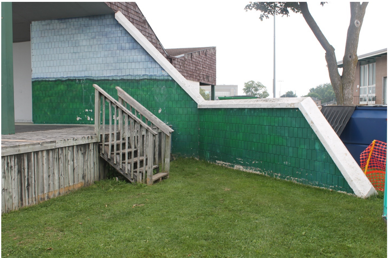
Image 4: Photograph showing the access to the south side of the Anne Eadie Park Stage, 2021.
