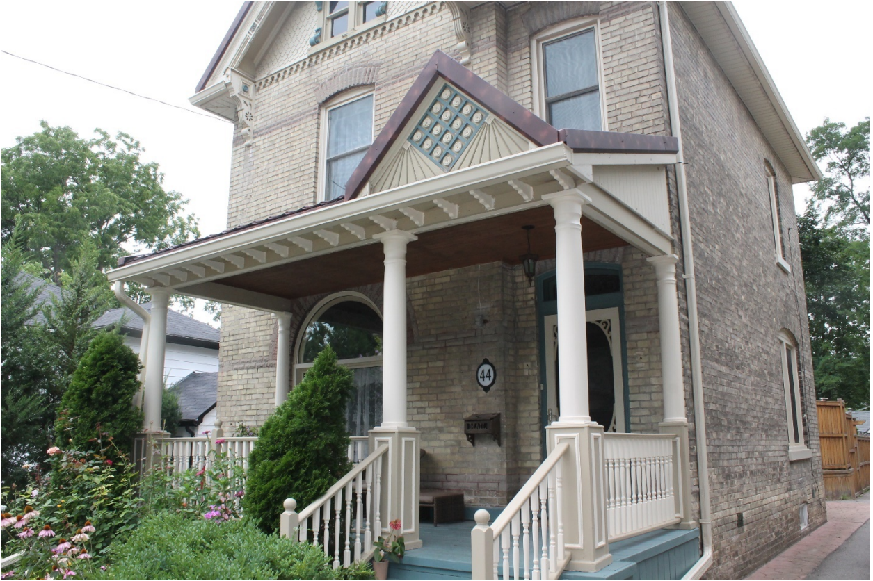
Image 13: Photograph showing porch located on the dwelling at 44 Bruce Street.
