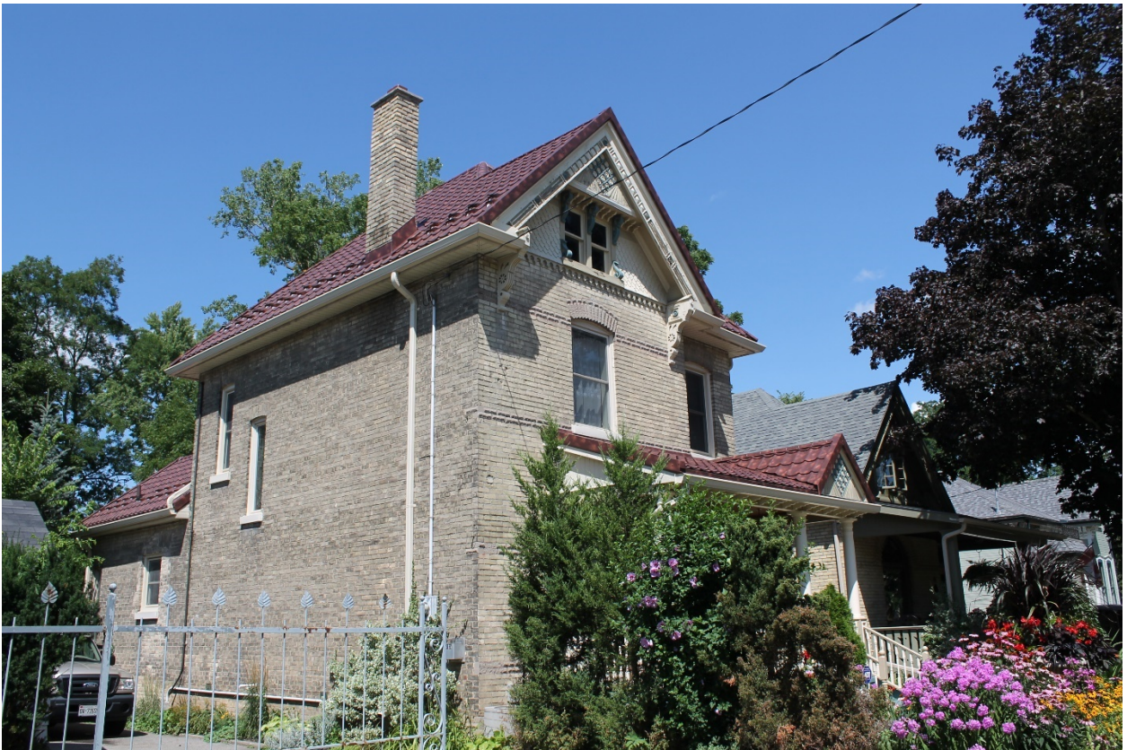
Image 2: Photograph of the west facade of the dwelling at 44 Bruce Street.
