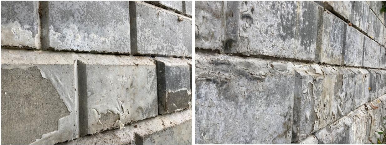
**Figure 1: Peeling and degraded anti-graffiti coating from Phase 1 and Phase 2**
