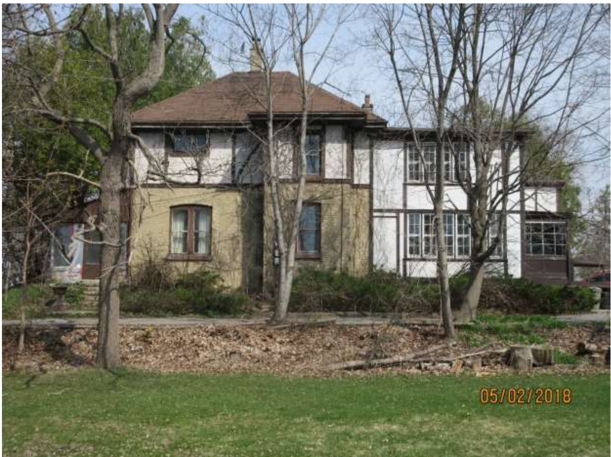
Image 6: View of the south façade of the house located at 2154 Richmond Street. Note the difference in exterior cladding materials and roof forms, which helps to articulate alterations to the original brick masonry building.
