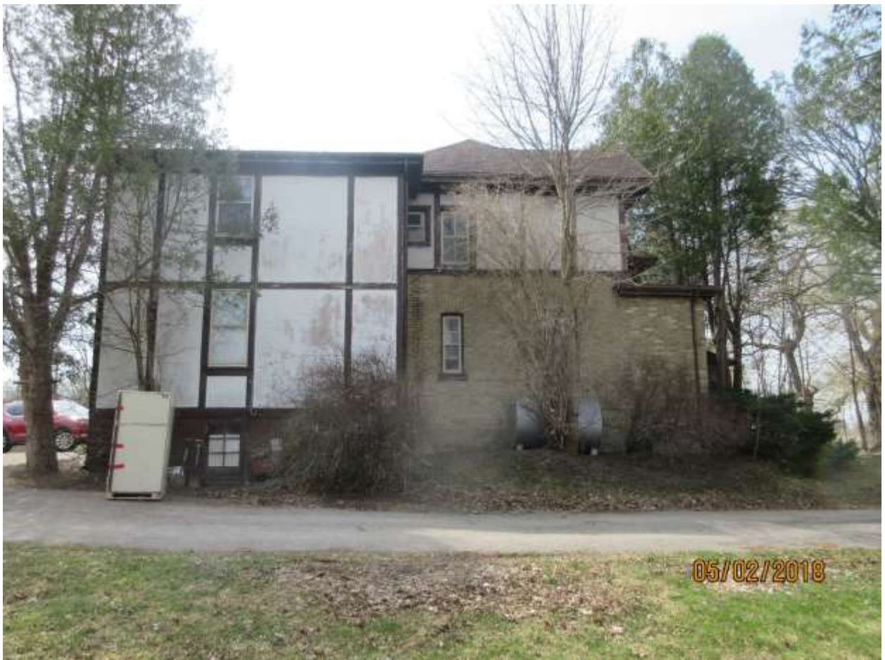
Image 8: View of the north façade of the house located at 2154 Richmond Street.
