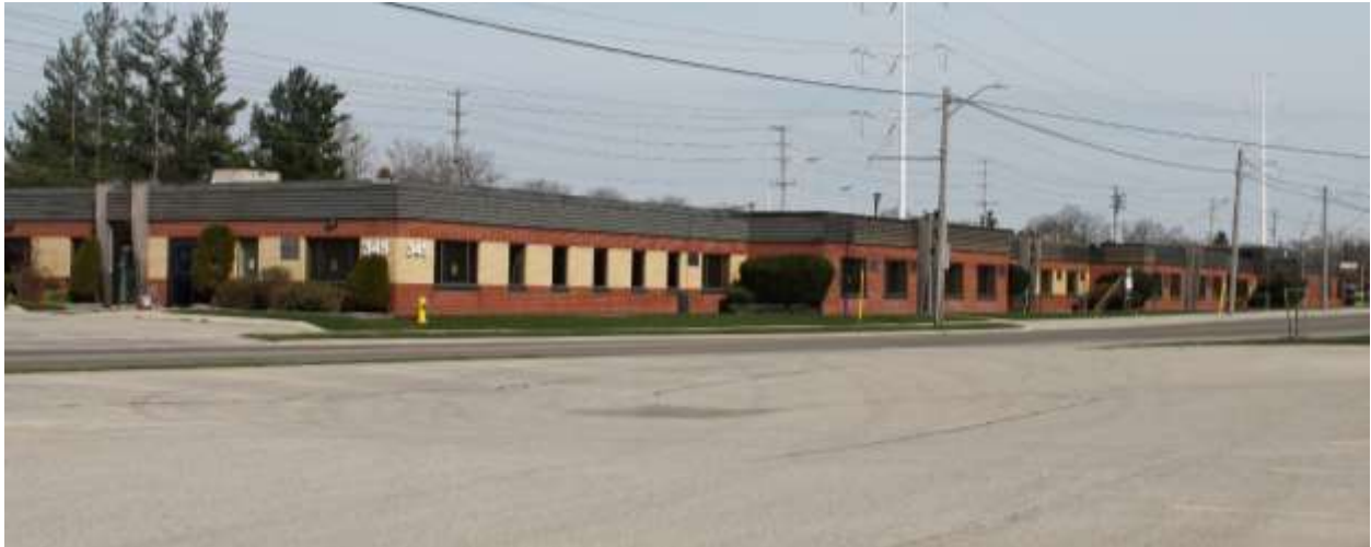
Figure 1: 335-385 Saskatoon Street (West Side) Looking North
