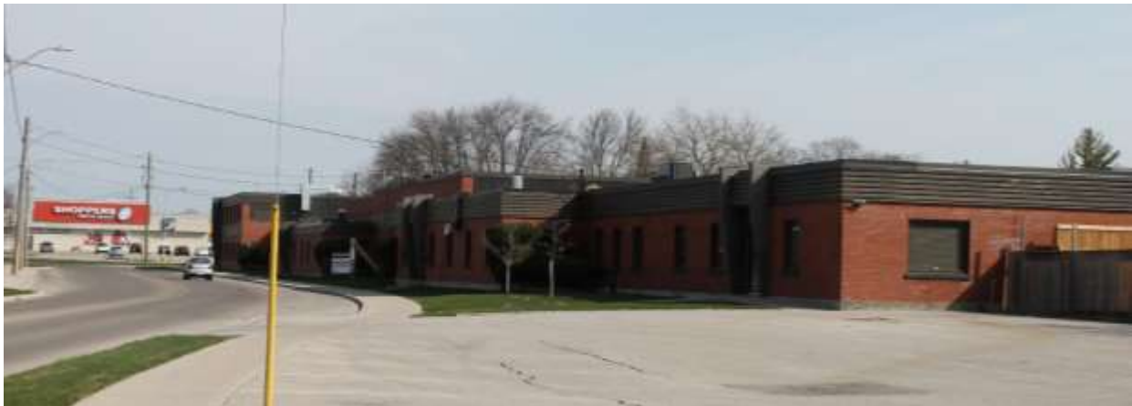
Figure 2: 340-390 Saskatoon Street (East Side) Looking North to Whitney Street
