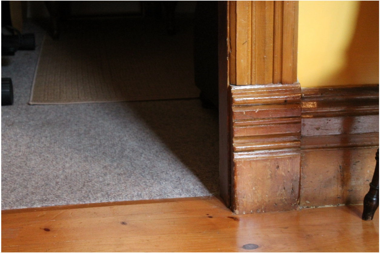
Image 17: Photograph showing detail of the baseboards on the interior of the dwelling.
