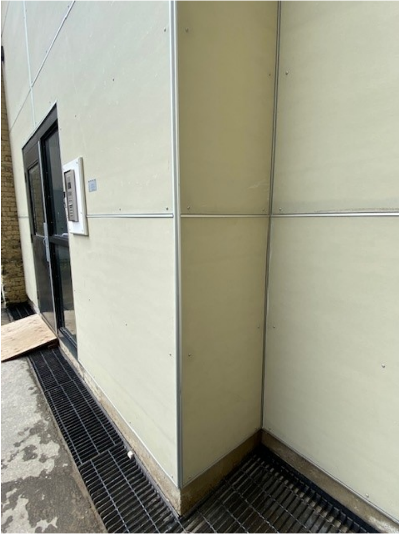
Image 6: Detailed view of cladding material (July 29, 2021)
