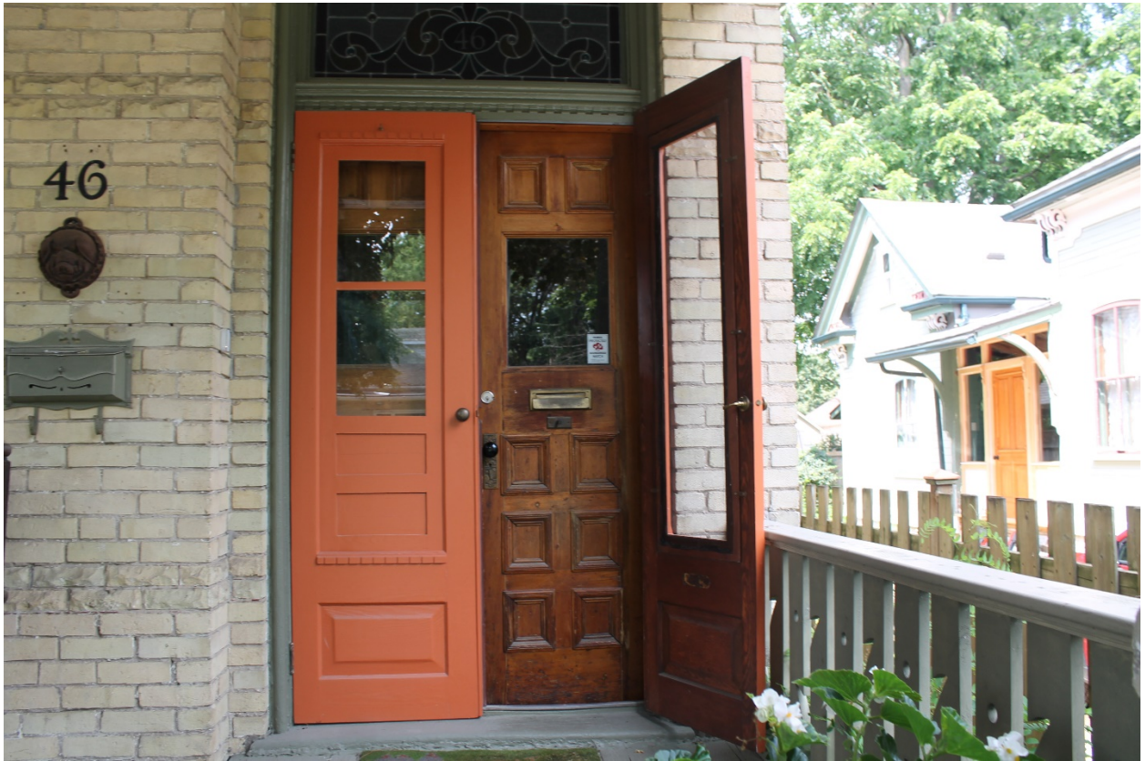
Image 6: Photograph showing the double-leaf front doors and storm doors.
