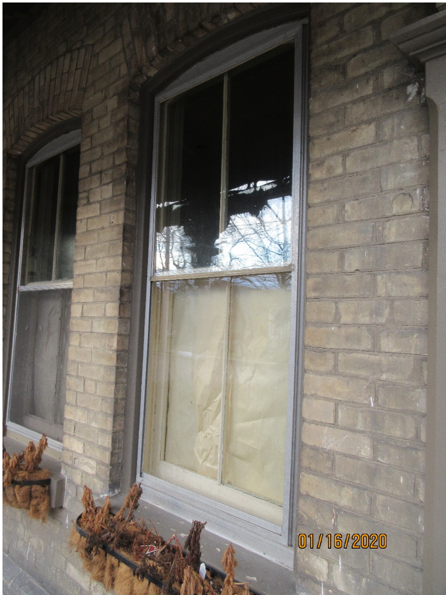
Image 4: Detail photograph of the windows under the porch on the property at 42 Askin Street. Note that the window openings are topped by a segmented arch brick voussoir; the wood windows feature a segmented arch top sash which is obscured by the rectangular aluminum storm window applied over top.
