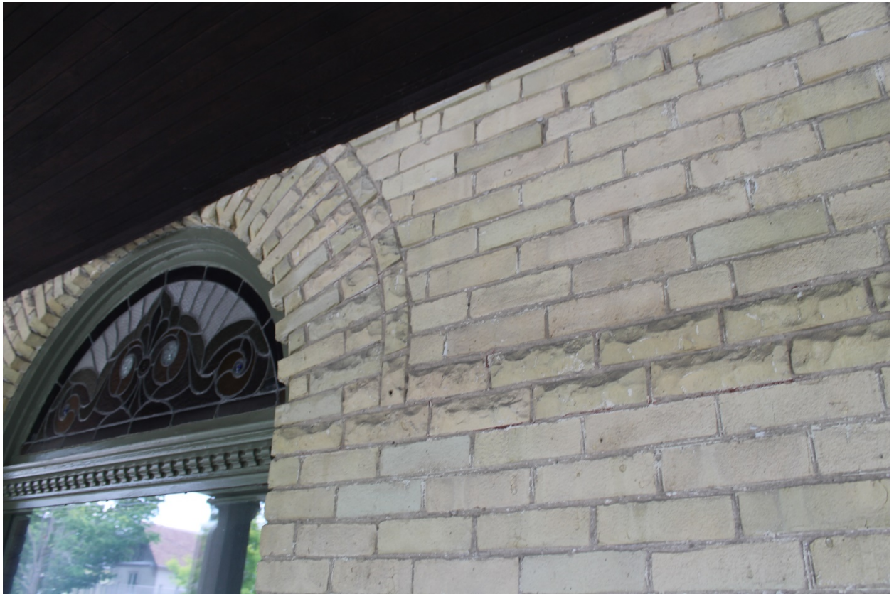
Image 4: Detail showing the rusticated buff brick string course and details of voussoirs.
