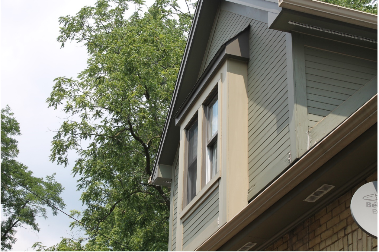
Image 10: Photograph showing the gable dormer on the west side of the dwelling.
