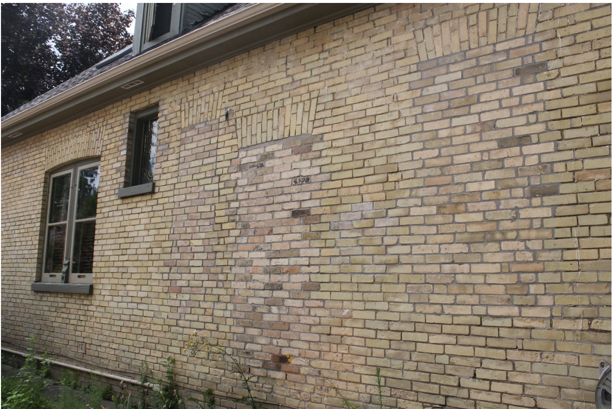
Image 14: Photograph of the east facade of the dwelling showing the remnants of former window openings and the existing windows.
