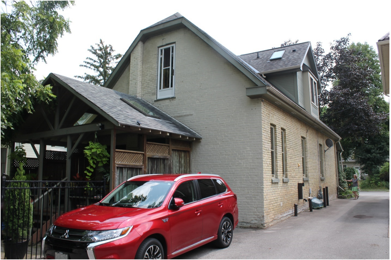
Image 13: Photograph showing the north (rear) facade of the dwelling, showing hipped gable roof, dormer on the west side of the dwelling, and rear covered porch.
