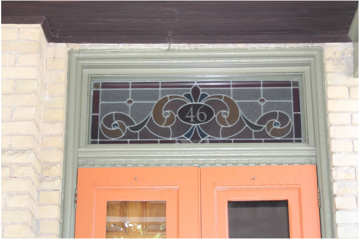
Image 3: Detail showing the heavy wood trim of the doorway, dentil detailing, and stained-glass transom window.
