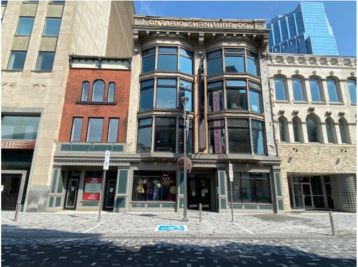
Image 1: View of Dundas Street façade (July 29, 2021)
