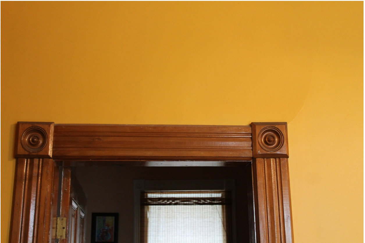
Image 16: Interior detail showing example of the wood trim and details found around the windows and doors on the interior of the dwelling.
