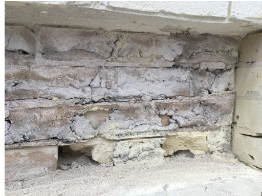
Test Cut showing Mortar between Wythes
