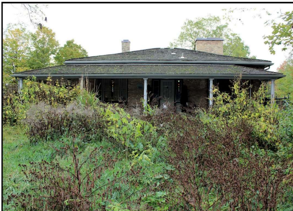
14. The front (west) elevation of Park Farm cottage from the front lawn.
