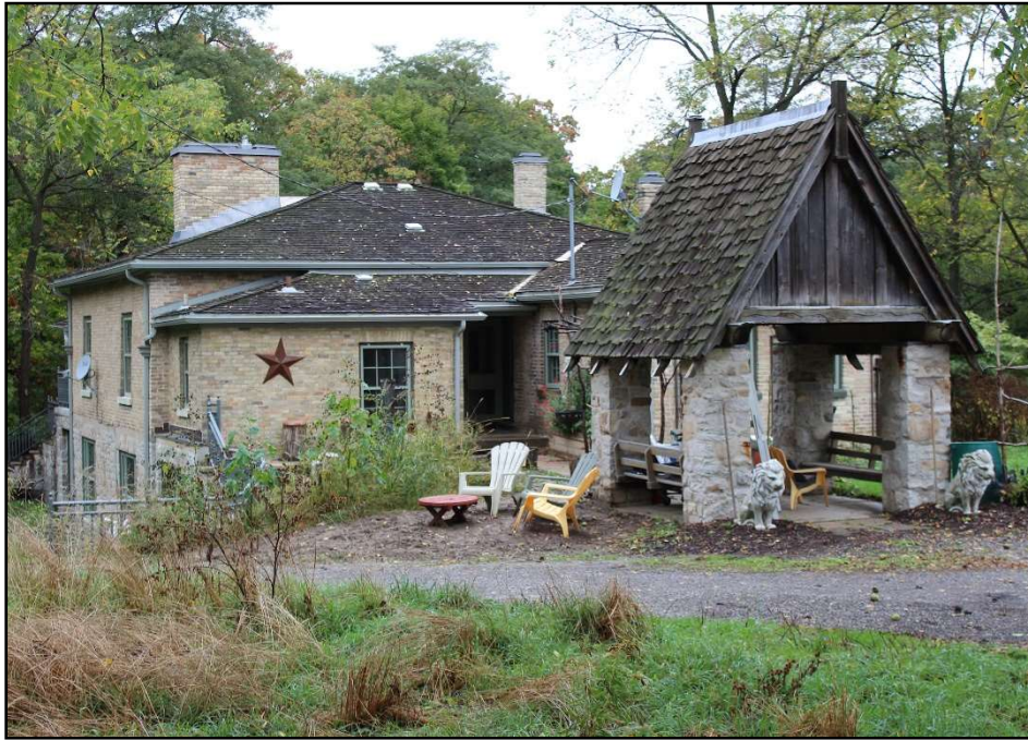
16. The rear (east) elevation of Park Farm cottage and lychgate viewed from the rear yard.
