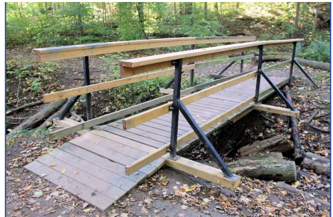
43. Walking trail bridge in Meadowlily Woods ESA.
