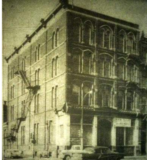
*View of 329 Richmond Street from East
