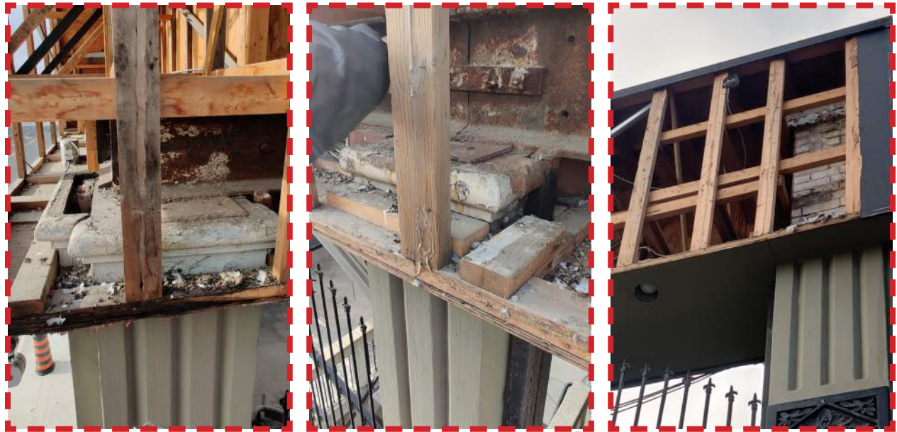
329 Richmond Street - Current Condition Detail Views
