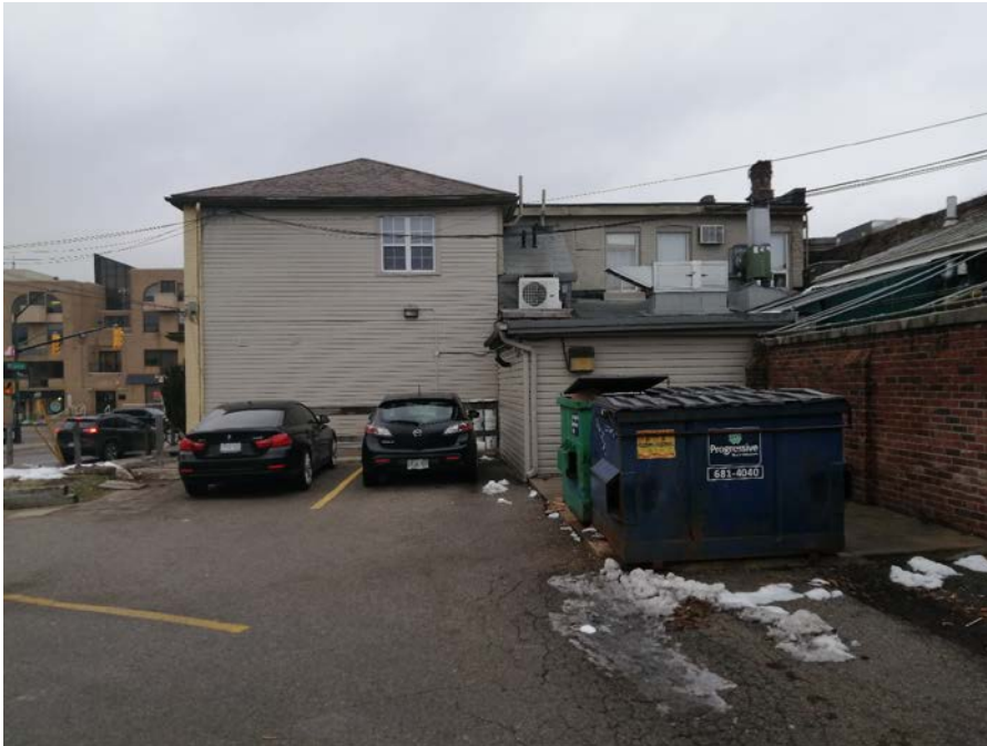
Figure 39: View of west elevation (Source: MHBC, 2020)
