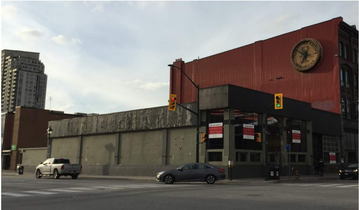
329 Richmond Street - Current Condition View of South Elevation from Southeast
