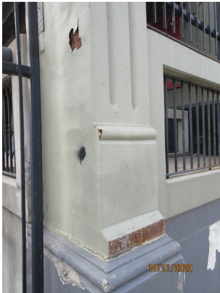
Image 2: Detail photograph of the cast iron column at 329 Richmond Street.
