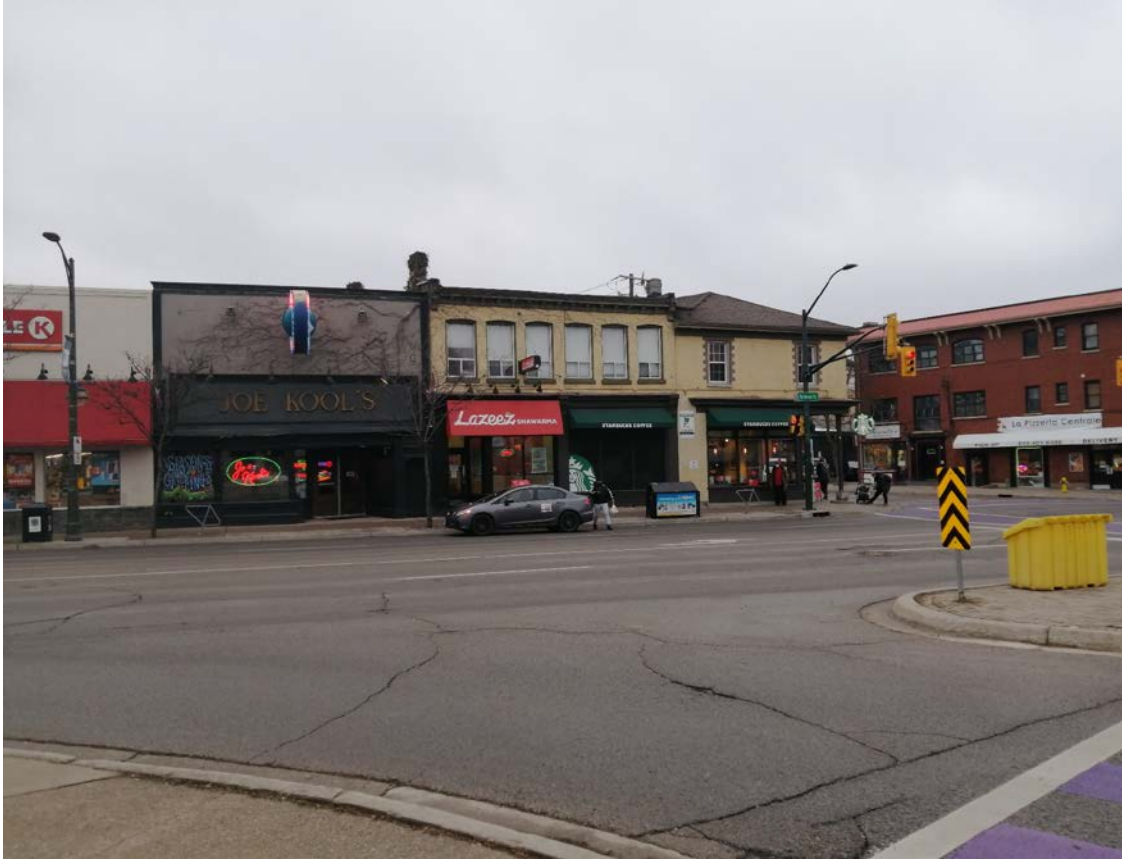
Figure 5: Streetscape view of 595, 599-601 Richmond Street from corner of Victoria Park (Source: MHBC, 2020)
