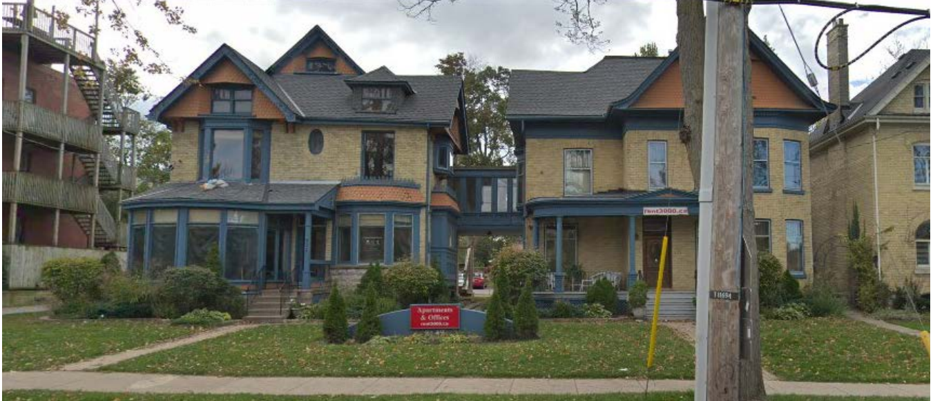
Image 6: 551-555 Waterloo Street: East/Front Elevation. Note two and a half storey massing, decorative gables, woodwork and projecting bay/window forms and window details. These aspects are significant within the HCD as they contribute to the visual consistency of the district as identified in the architectural character elements within the designation under Part V (OHA). Some original features appear to remain, while many have been replaced. The two properties have been modified with the addition of a contemporary pedway at the second storey (rear). The overall heritage value lies in its location and grouping, and remaining architectural merit as Victorian style residences, contributing to the overall context of the value of the HCD. Google Streetview, 2020.
