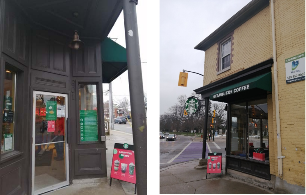
Figures 34 & 35 – (left) View of entrance to 601 Richmond Street via south-west corner of the intersection at Richmond Street and Central Avenue. (right) View of front façade looking south, (right) View of entrance at corner of the intersection looking south-east (Source: MHBC, 2020).
