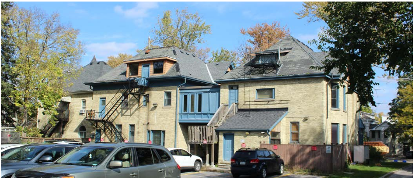
Image 7: 551-555 Waterloo Street: West/Rear Elevation with parking area. A contemporary dormer with an access door has been added to the upper half storey at the rear of 555 Waterloo Street, and a small addition added to the ground floor of 551 Waterloo Street at grade. The pedway can be seen connecting the two properties at second storey with a pathway below. Contemporary additions and exit staircases have also been added to the rear. Google Streetview, 2020.
