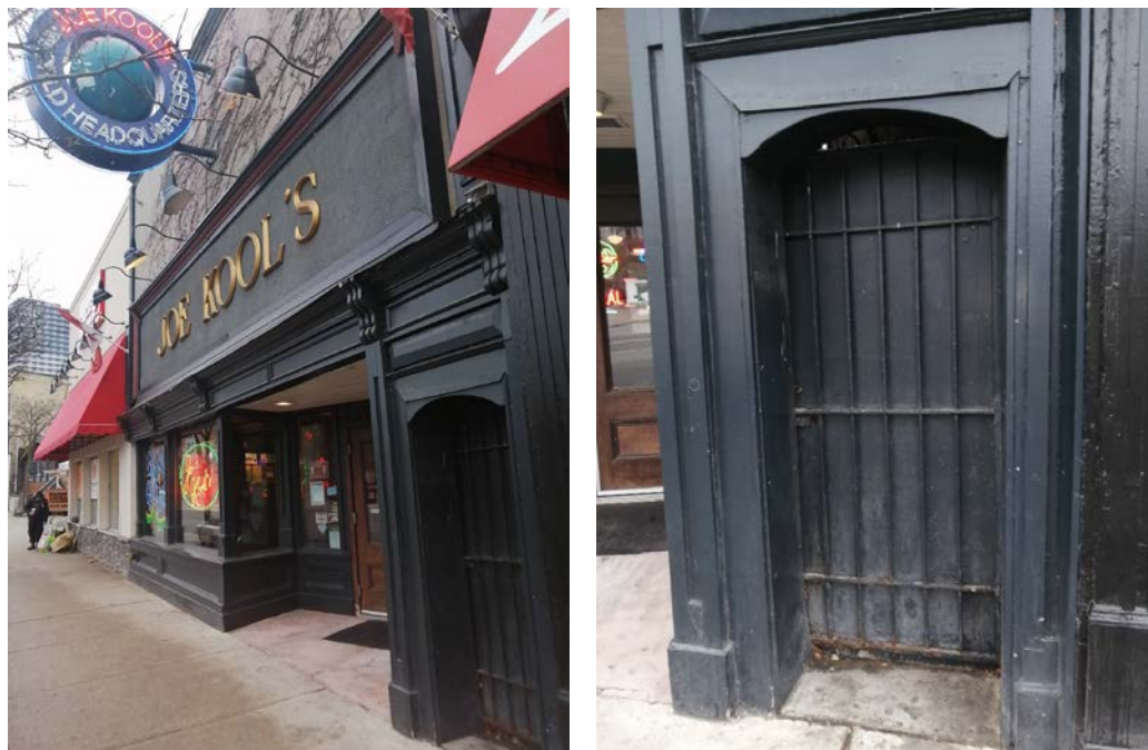
Figures 41 & 42– (left) View of front façade of 595 Richmond Street including restaurant “Joe Kool’s” to the north and “Circle K” to the south; (right) View of door opening/ access that leads to alleyway to brick ancillary structure to the rear of 595 Richmond Street (Source: MHBC, 2020)
