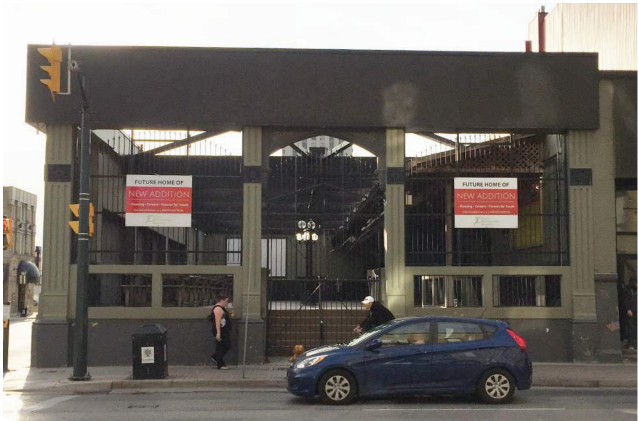
329 Richmond Street - Current Condition East Elevation
