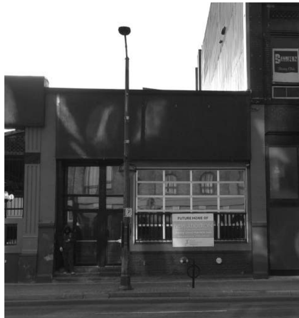
2016 - 331 Richmond Street, East Elevation
