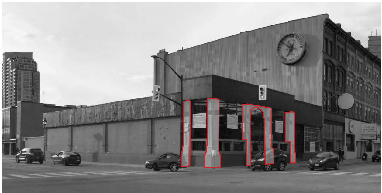
Figure 1.4 - 333 Richmond Street Historic Attributes View looking Northwest from York Street
