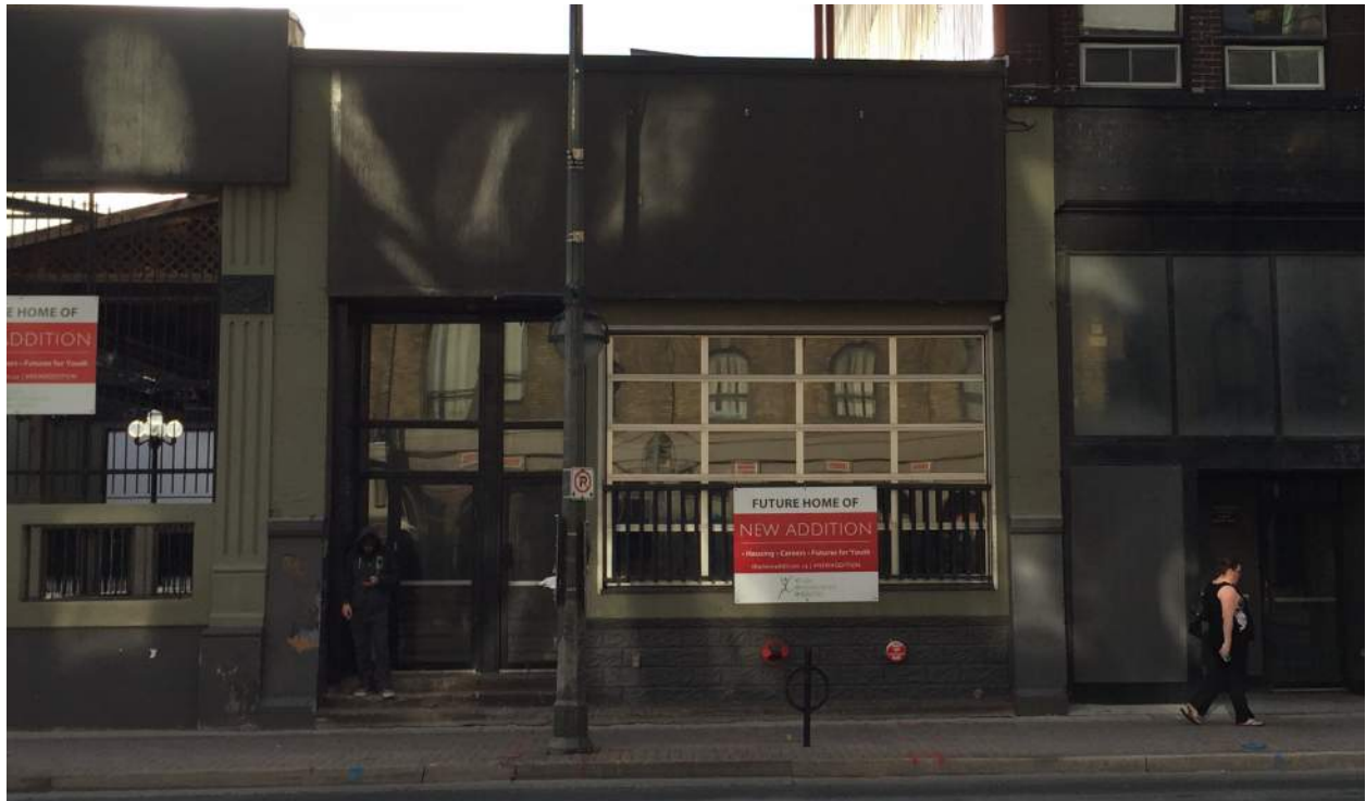
331 Richmond Street - Current Condition East Elevation
