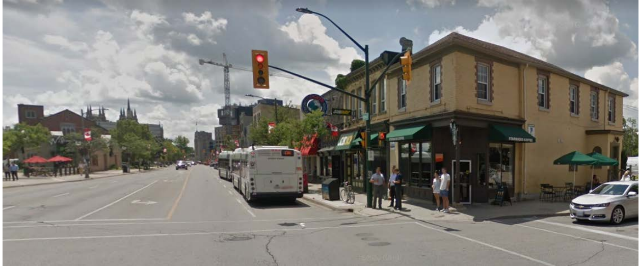
Figure 59- Kinetic view of existing built heritage on subject lands travelling southwards along Richmond Street (Source: Google Earth Pro, 2020)
