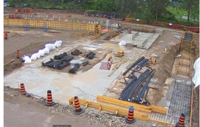
Site Photo of Construction at 122 Base Line Rd West
