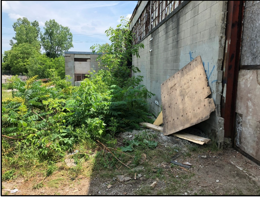
Photo 1 - rear of abandoned building
