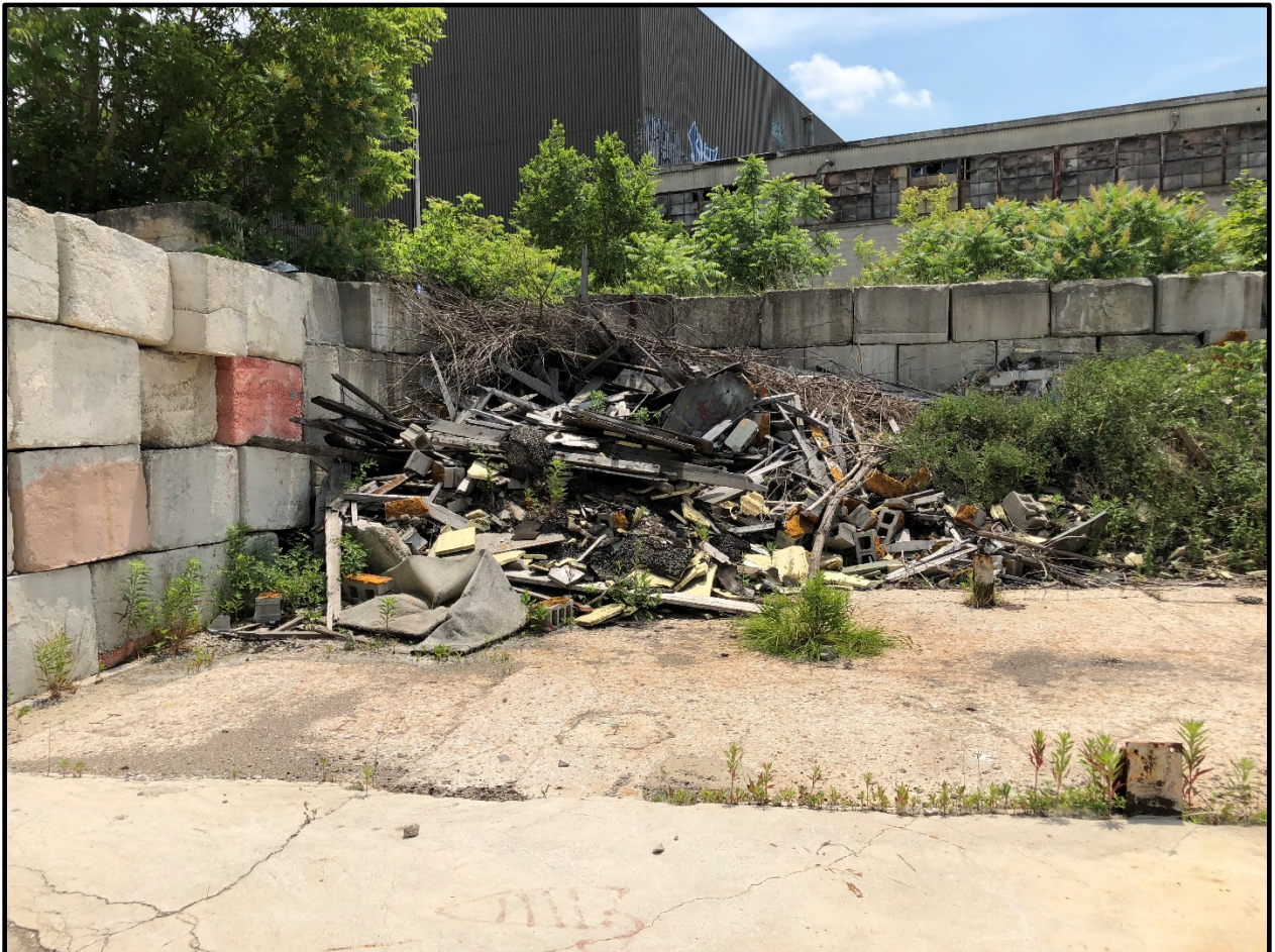
Photo 2 - rear of abandoned building
