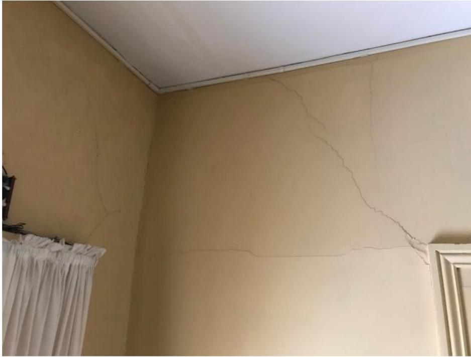
*Areas of the house where structural damage could be worsened are illustrated by the existing weaknesses in wall plaster, with an underlying structural cause*
