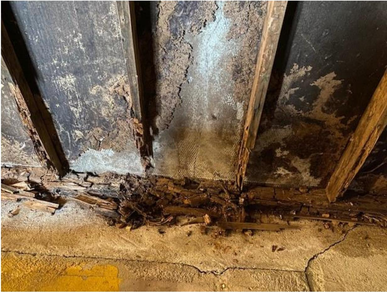
Image 5: Interior view of detached garage showing degradation of wood sill and wall studs (April 22, 2021)
