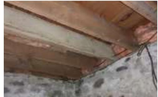
Image 8: Existing basement joists on rubble/fieldstone foundation. Photo Source: HIS, Stantec Consulting Ltd, April 2018.
