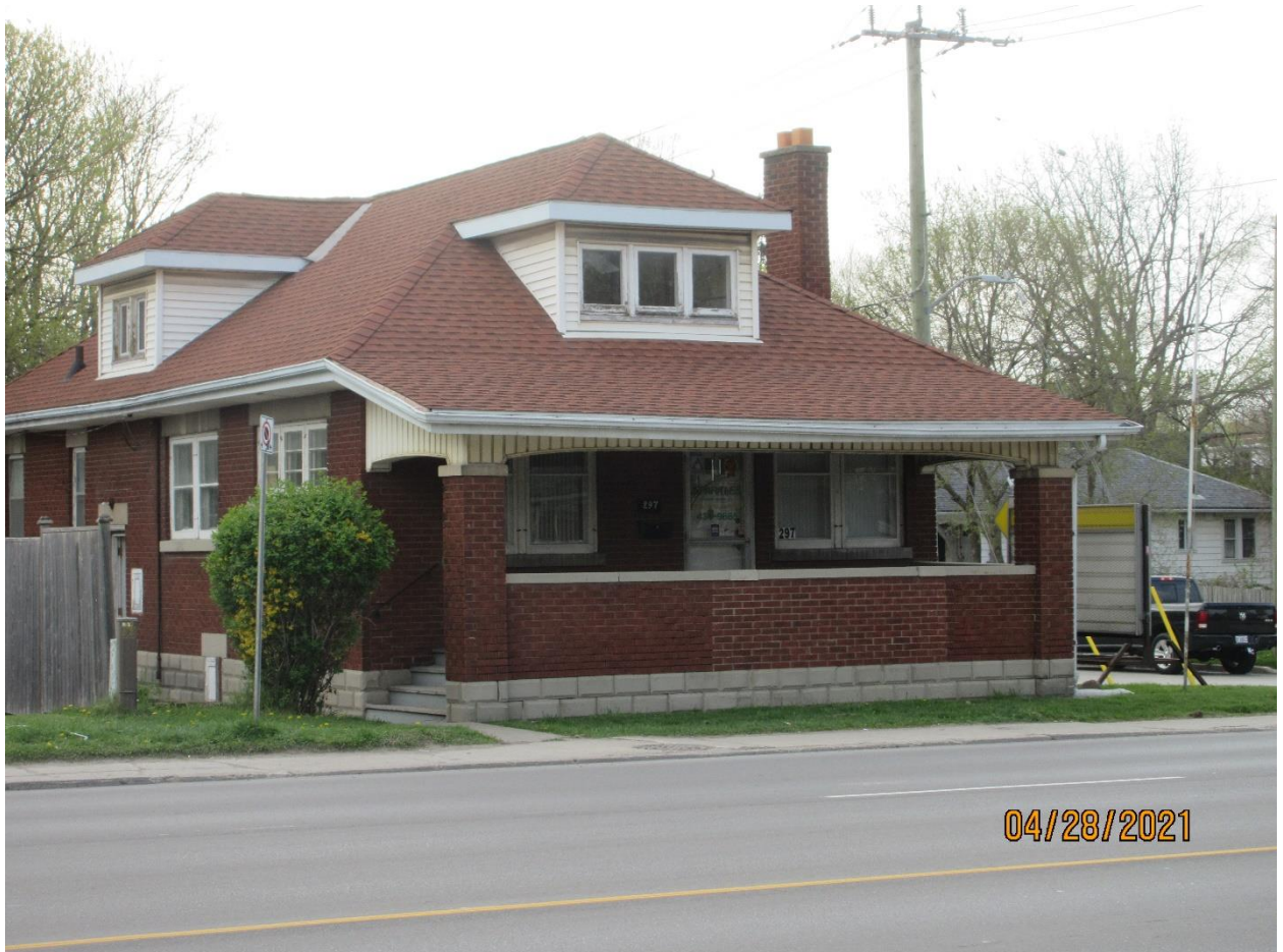
Image 34: Subject property at 297 Wellington Road.
