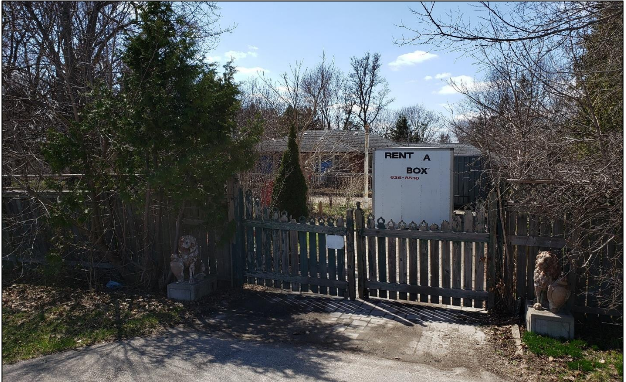
Figure 1: 1697 Highbury Avenue North (view of house from Highbury Avenue North)
