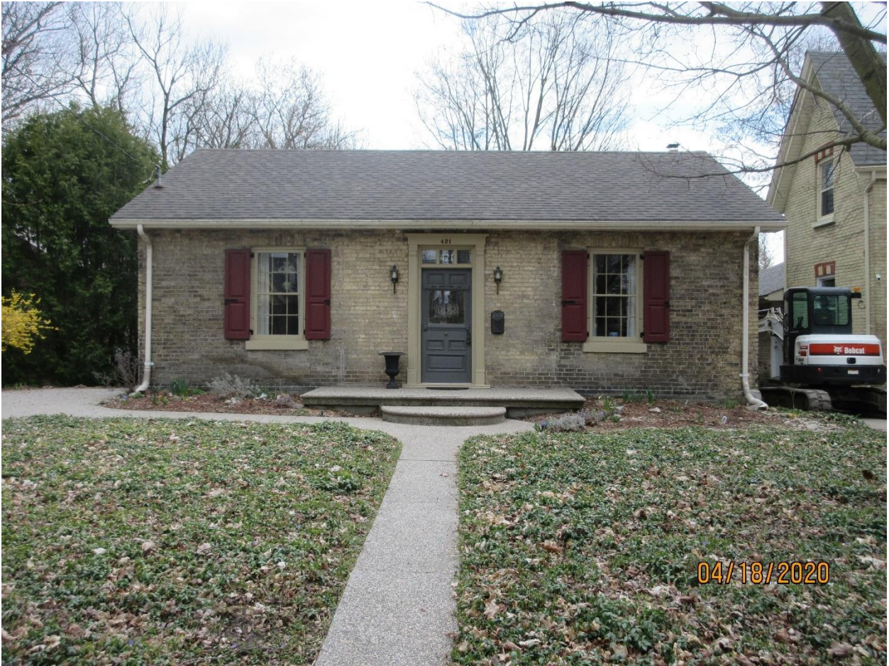
Image 20: Photograph showing the dwelling located at 421 Pall Mall Street, a heritage listed property.
