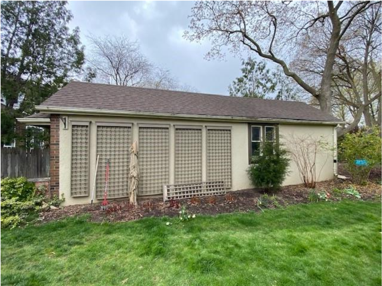
Image 3: Side view of detached garage, west elevation (April 22, 2021)
