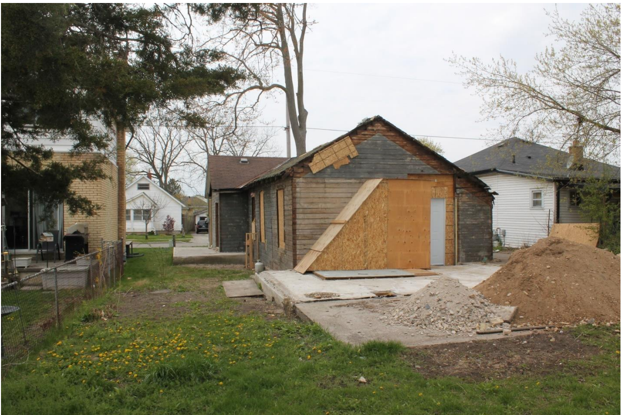
Image 12: Photograph looking east from the rear of the lot showing the back of the rear addition and footprint of the previously demolished two-storey addition, 2021.
