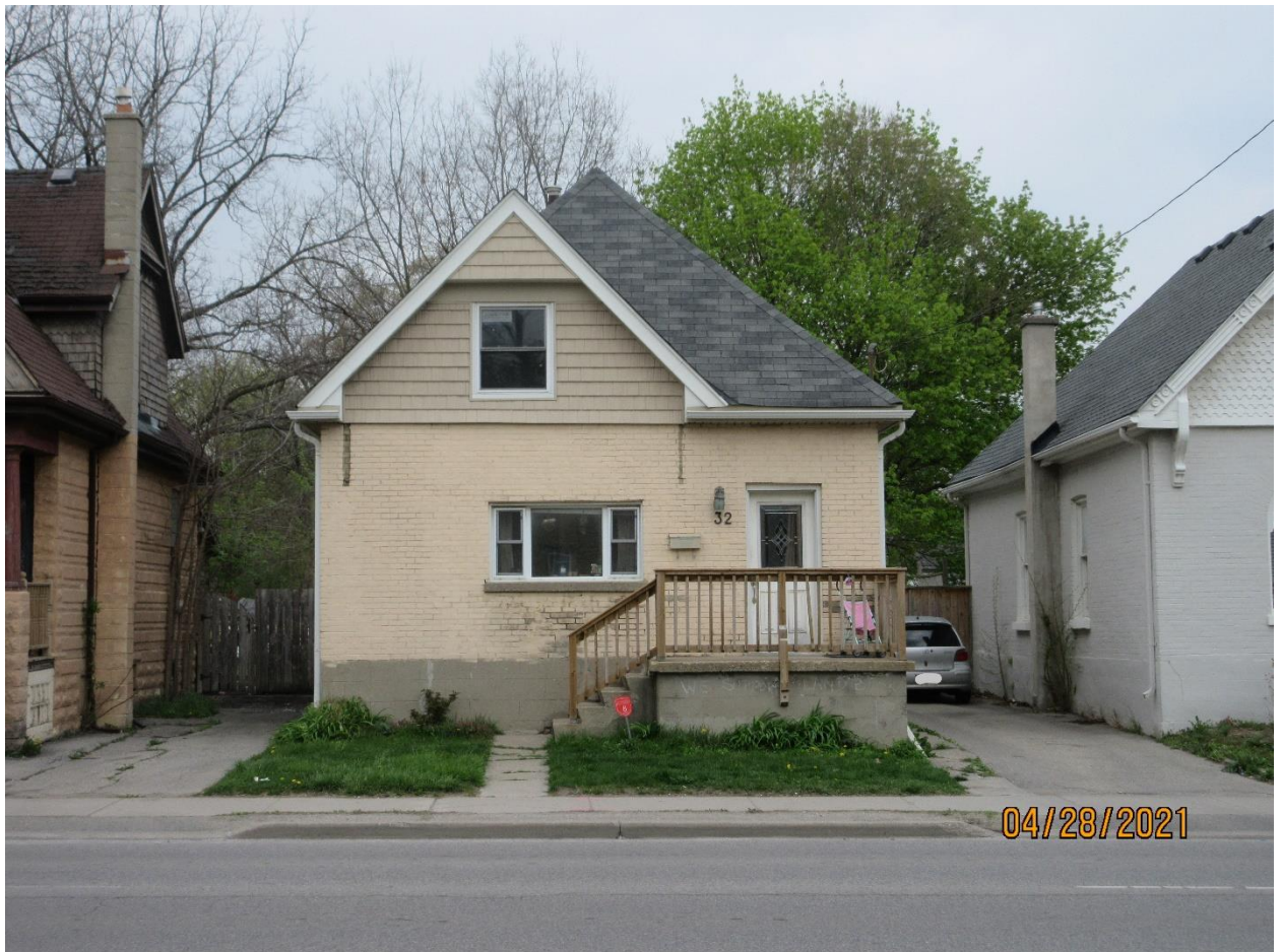
Image 4: Subject property at 32 Wellington Road.
