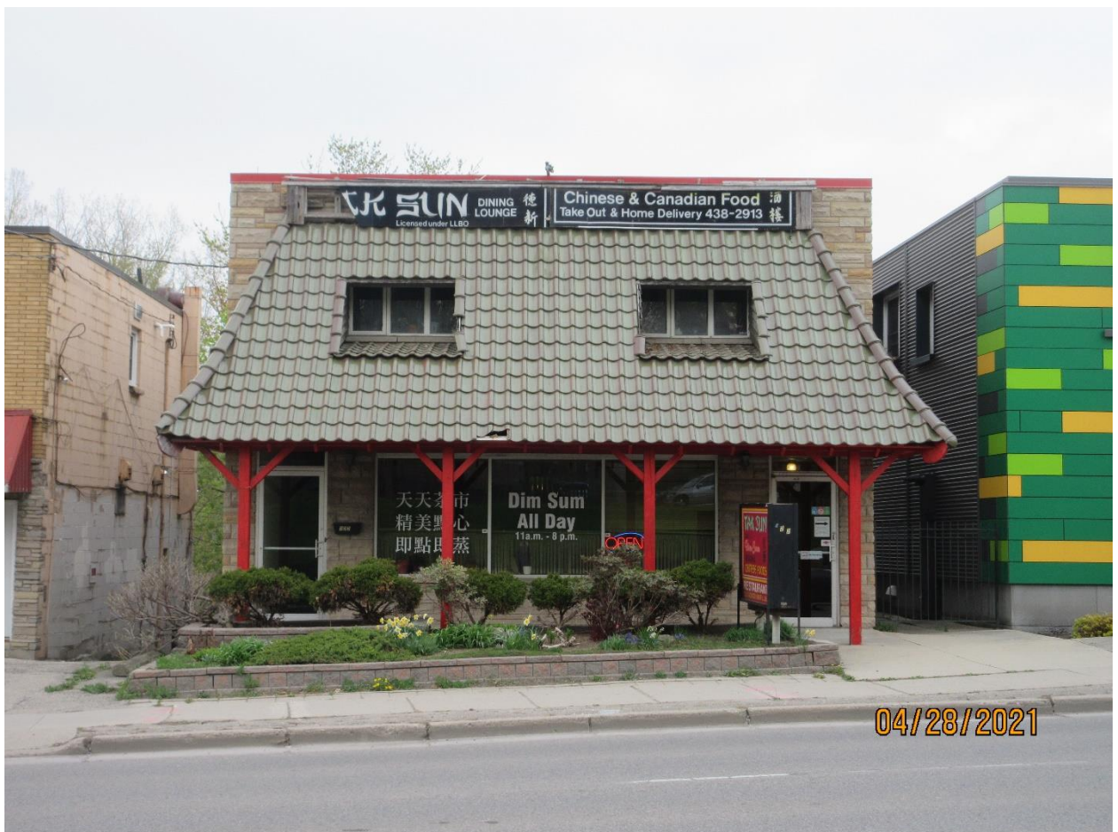
Image 10: Subject property at 120 Wellington Road.
