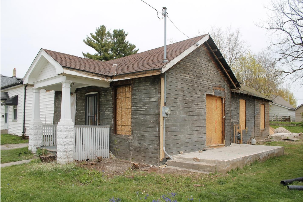
Image 8: Photograph showing the west (front) facade and the south facade of the dwelling. The rear addition is visible, 2021.
