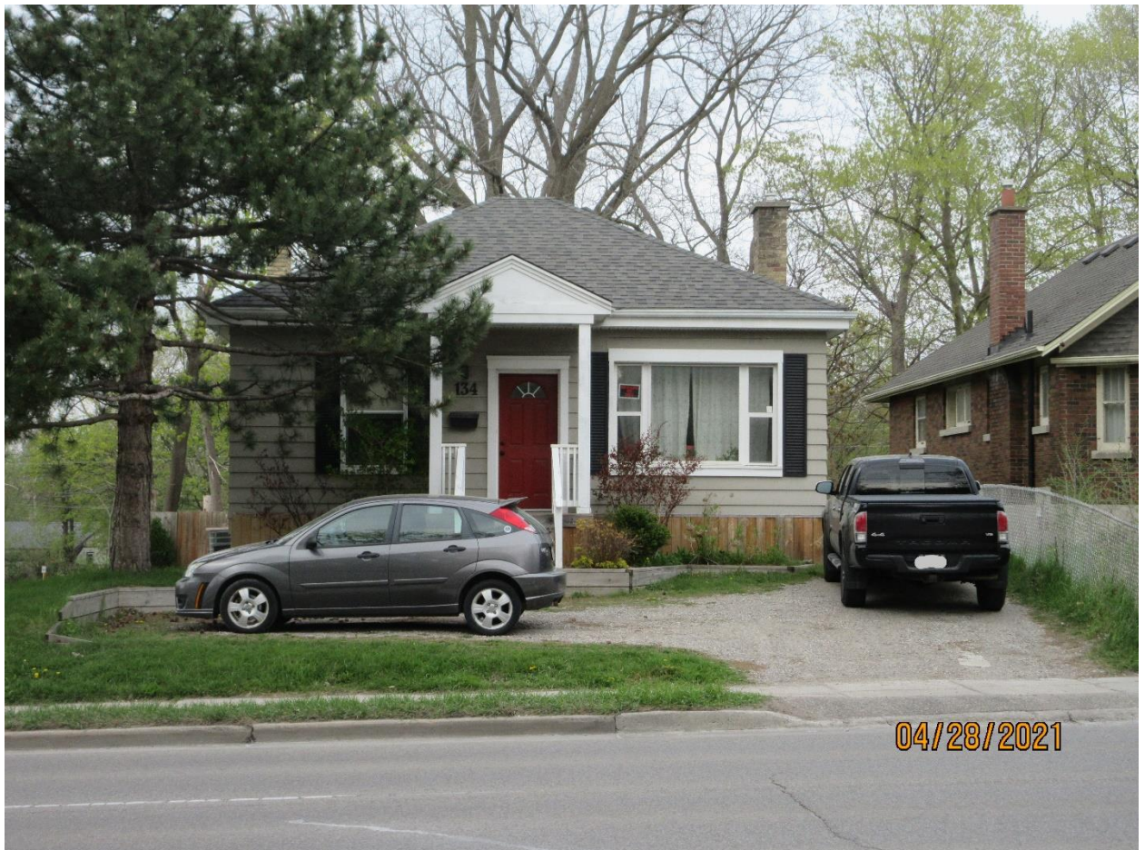
Image 12: Subject property at 134 Wellington Road.
