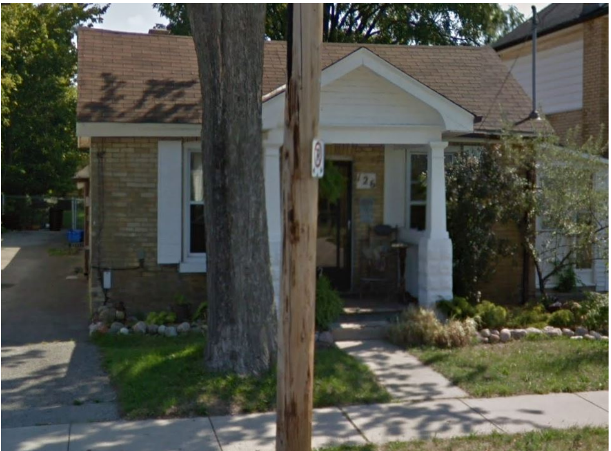
Image 2: Image showing the dwelling located at 126 Price Street, 2012 (Google Street).
