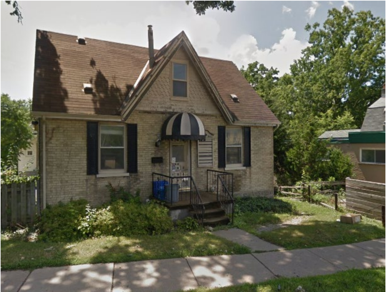
Image 18: Photograph showing the dwelling located at 2 Oxford Street West, included within the Blackfriars/Petersville Heritage Conservation District (Google Street).
