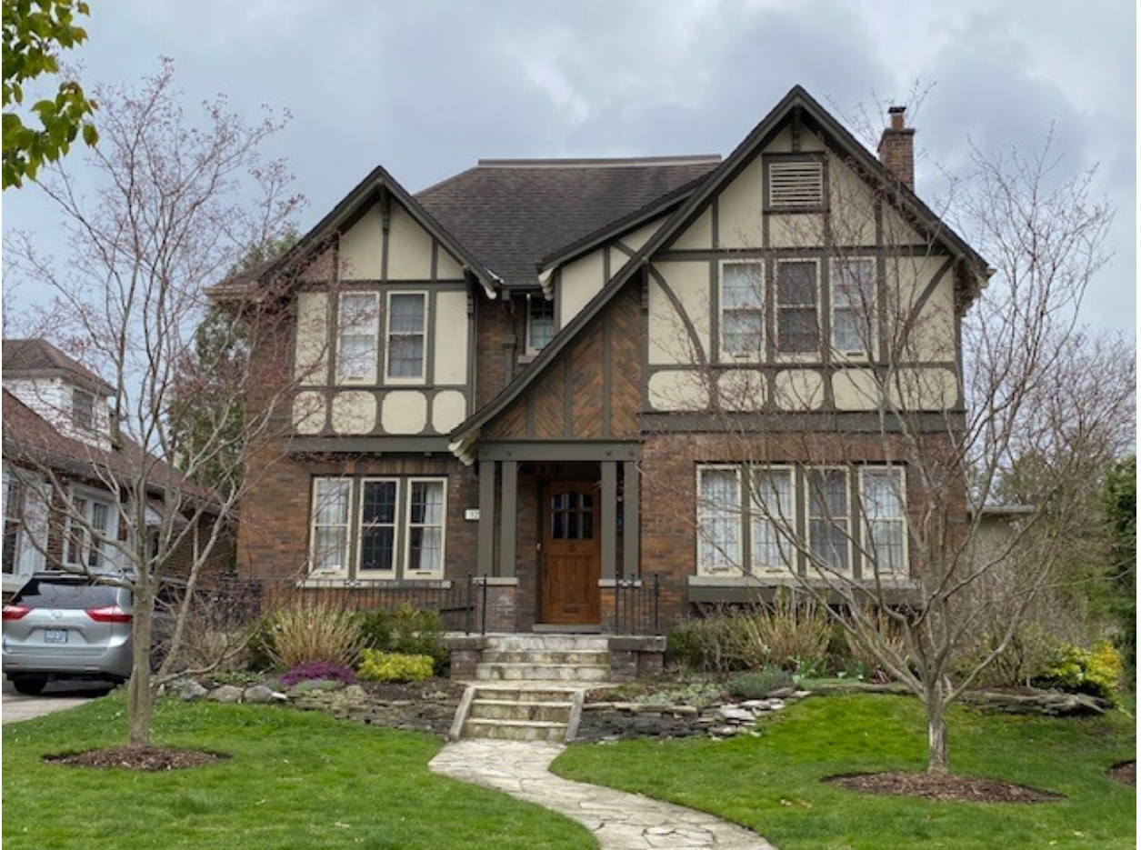
Image 1: Façade of residence at 325 Victoria Street, north elevation (April 22, 2021)
