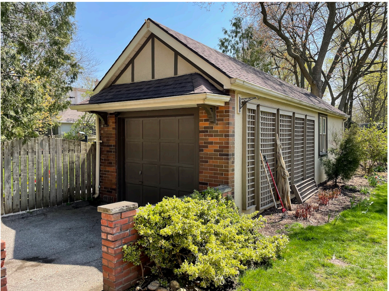
Image 2: Front-side view of detached garage, north-west elevations (April 22, 2021)
