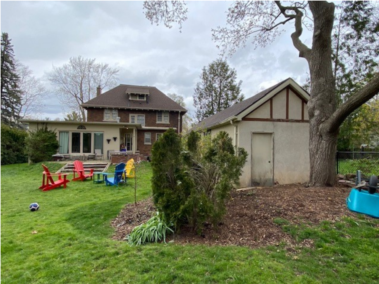
Image 4: Rear view of residence and detached garage, south elevations (April 22, 2021)
