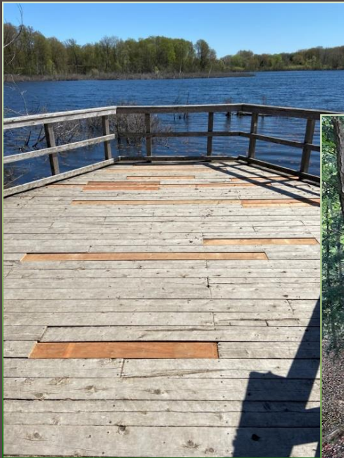
Saunders Pond viewing platform
