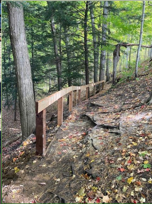
New railing in Kains
