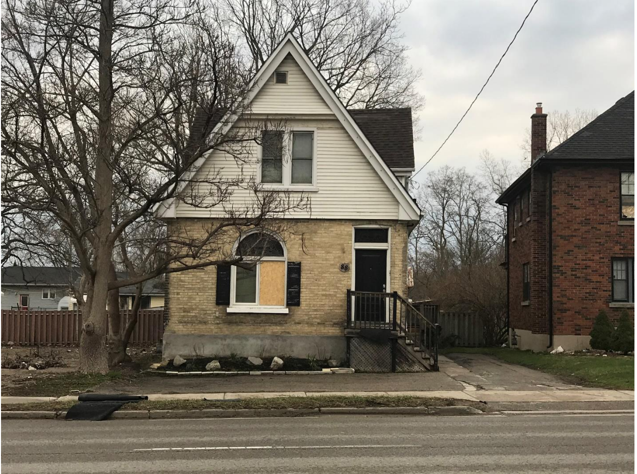
Image 1: Photograph of the subject property at 88 Wellington Road, seen from the west side of Wellington Road looking east (April 5, 2021).
