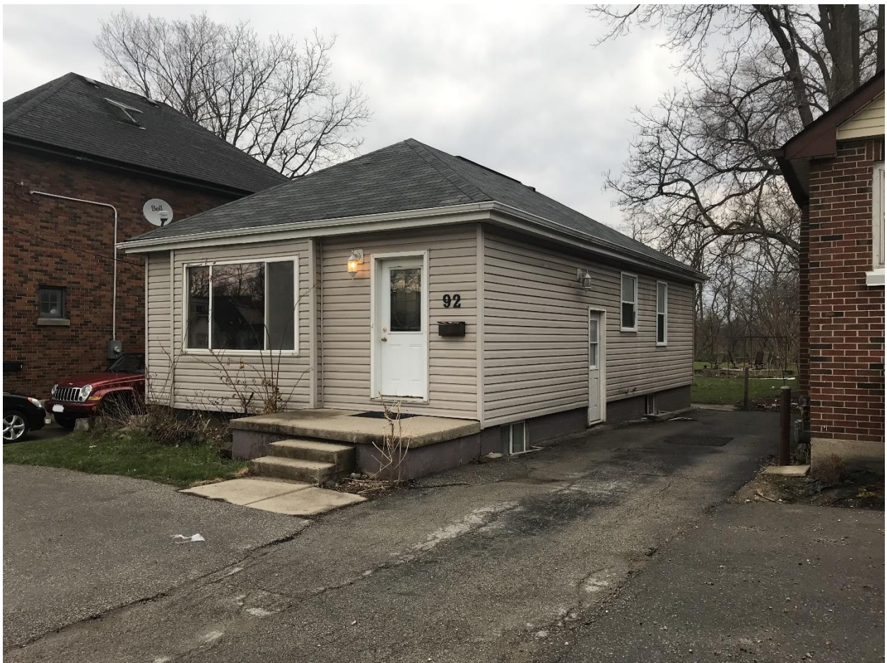
Image 2: Detail photograph of the subject property at 92 Wellington Road, showing the front (west) and south elevations (April 5, 2021).
