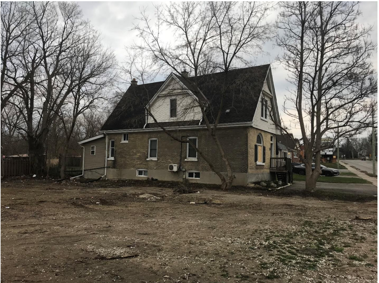
Image 2: Photograph showing the north and west (main) elevations of the building at 88 Wellington Road (April 5, 2021).
