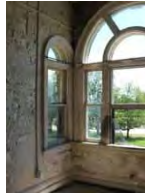
Arched window, 2 nd floor
