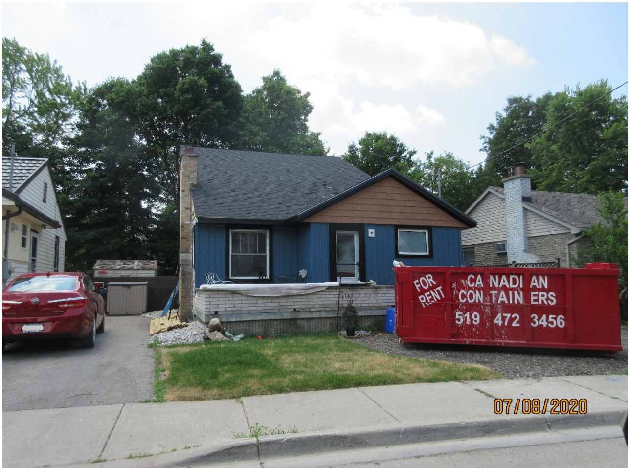
Image 4: Photograph of the subject property, on July 8, 2020, when non-compliance with the Heritage Alteration Permit was identified. Note the change in the exterior cladding, including gable, and the front door replacement. The shutters were also removed.
