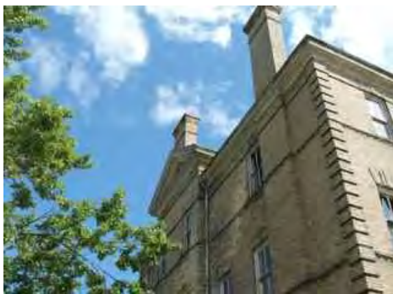
West elevation, central block
