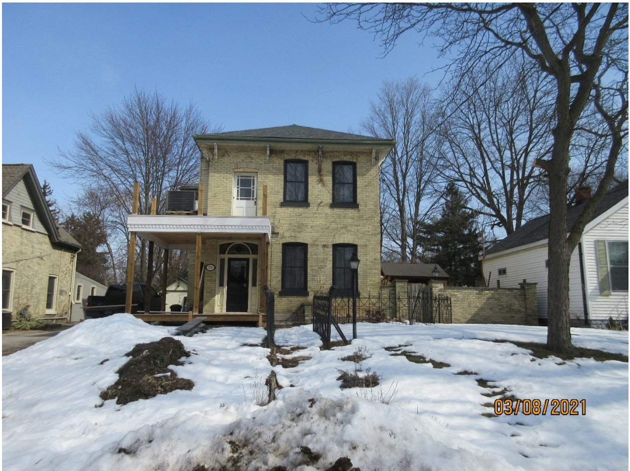
Image 4: Photograph of the property at 574 Maitland Street showing completed window alterations, March 2021.
