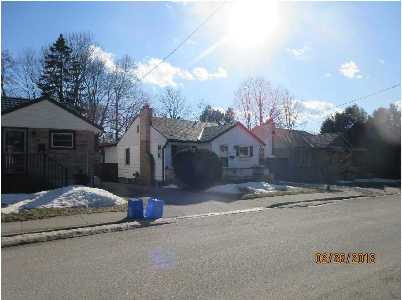
Image 3: View southwest showing the Contributing Resource at 16 Cummings Avenue prior to alterations on February 26, 2018.
