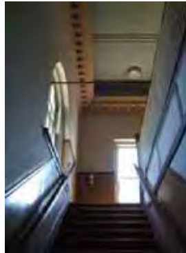
Stairs to gallery
