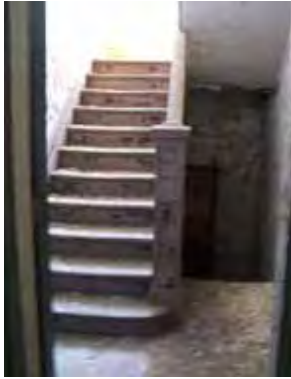
East stair, main level
