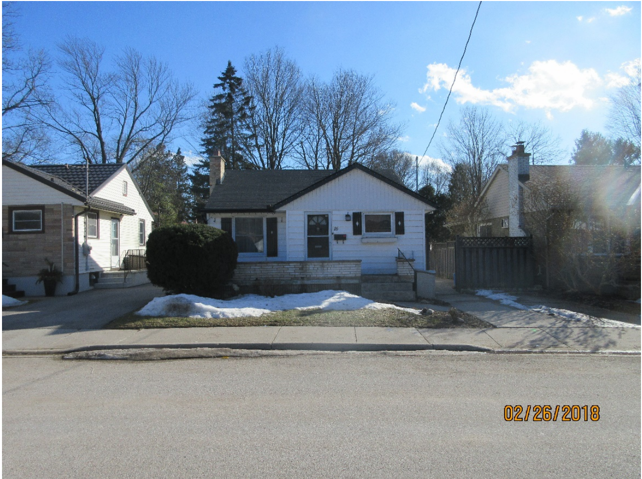
Image 1: Photograph showing the subject property, 16 Cummings Avenue, prior to alterations, on February 26, 2018.
