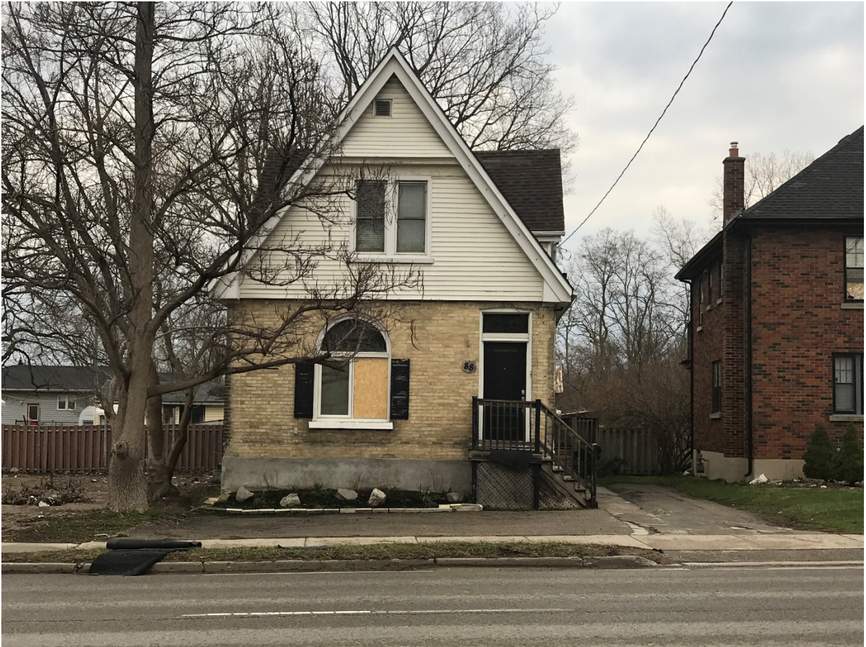
Image 1: Photograph of the subject property at 88 Wellington Road, seen from the west side of Wellington Road looking east (April 5, 2021).
