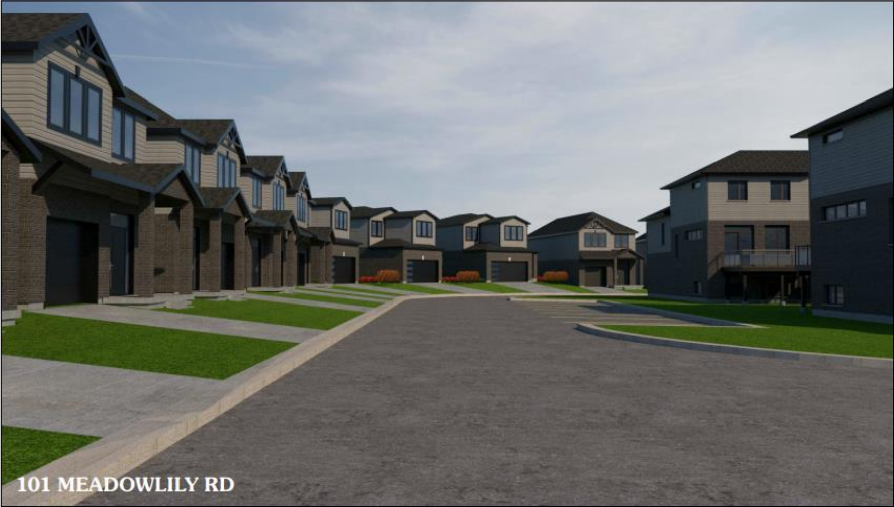
View Looking West Along Private Street 'A'
