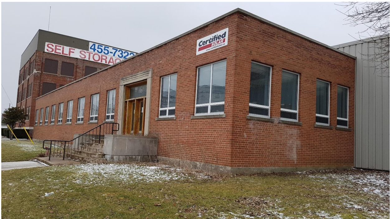
Figure 1: Front of 1153-1155 Dundas Street (facing Dundas Street)
