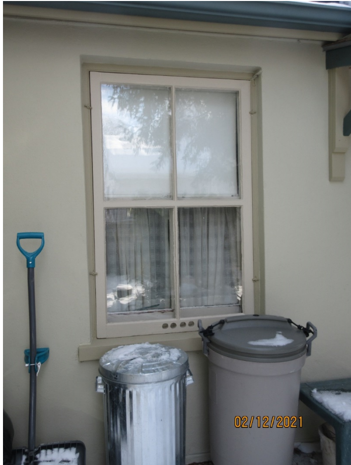
Image 25: Photograph showing the two-over-two painted wood window and storm window in the kitchen wing.
