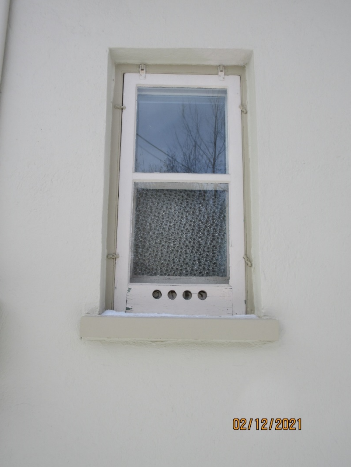
Image 32: Photograph of the bathroom window on the east façade with patterned glass in the lower lite and clear glass in the upper lite of the hung window with a storm window and wood sill.
