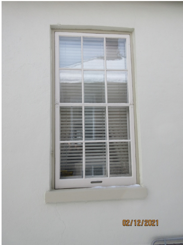
Image 34: Photograph of the six-over-six double hung painted window with matching storm window and wood sill on the east façade.
