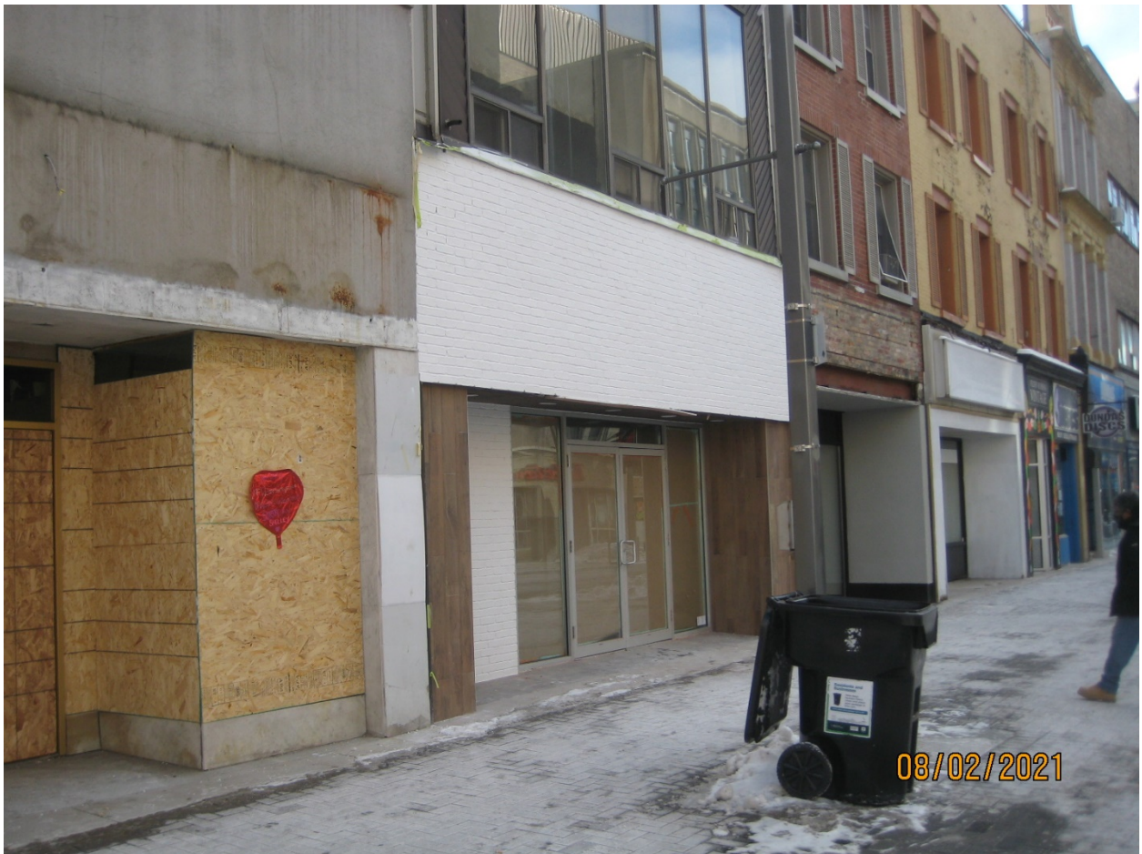
Image 6: Photograph of the property at 181 Dundas Street showing the unapproved alterations including painted brick veneer and faux wood grain porcelain tile.
