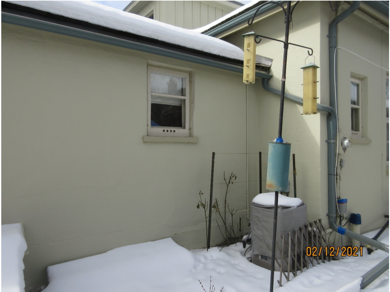
Image 31: Showing the junction of the kitchen wing and the house along the easterly façade of Carfrae Cottage.
