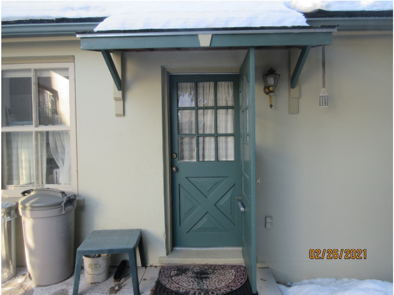
Image 27: Photograph showing the painted wood kitchen door, with nine lites and X-pattern panelling below.
