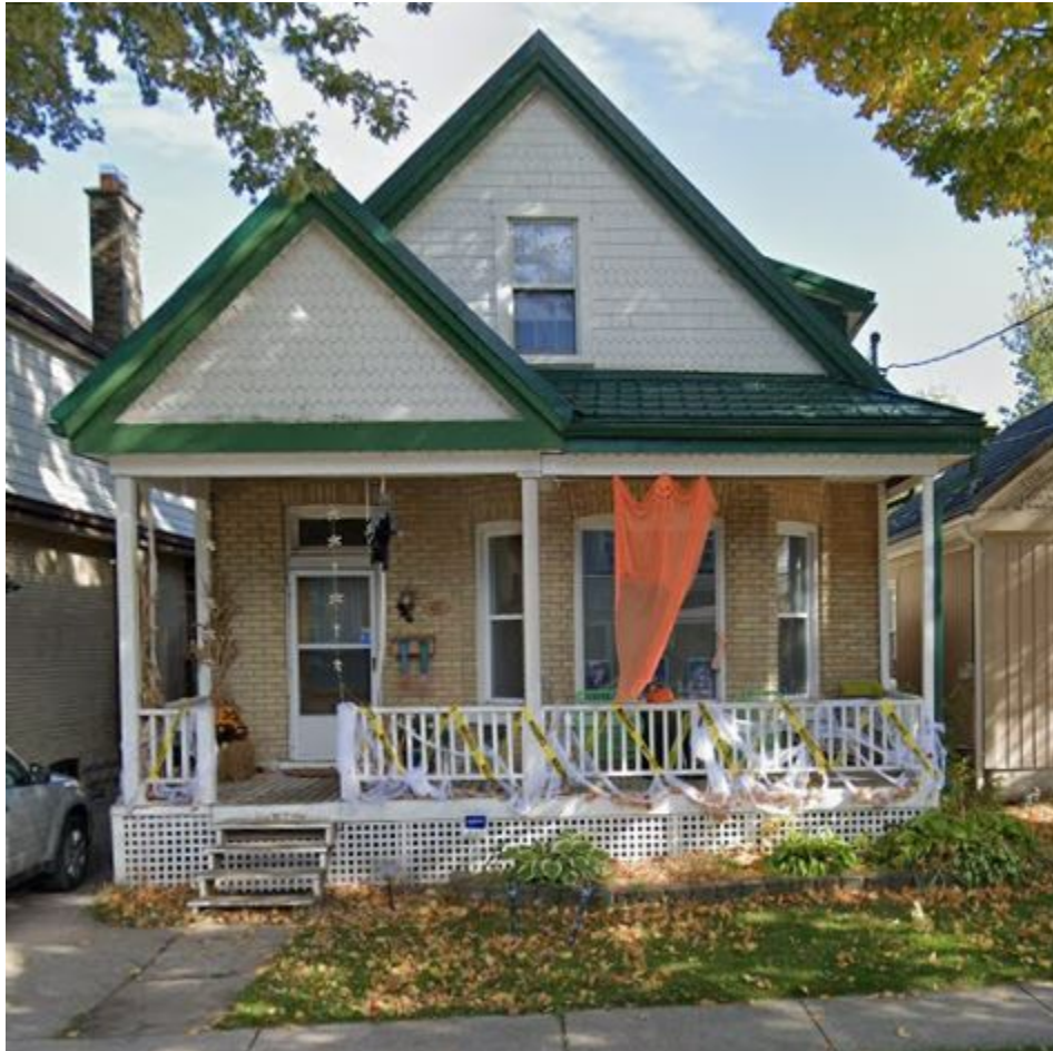
Image 1: Image of the property at 61 Wilson Avenue in October 2018 (courtesy Google).
