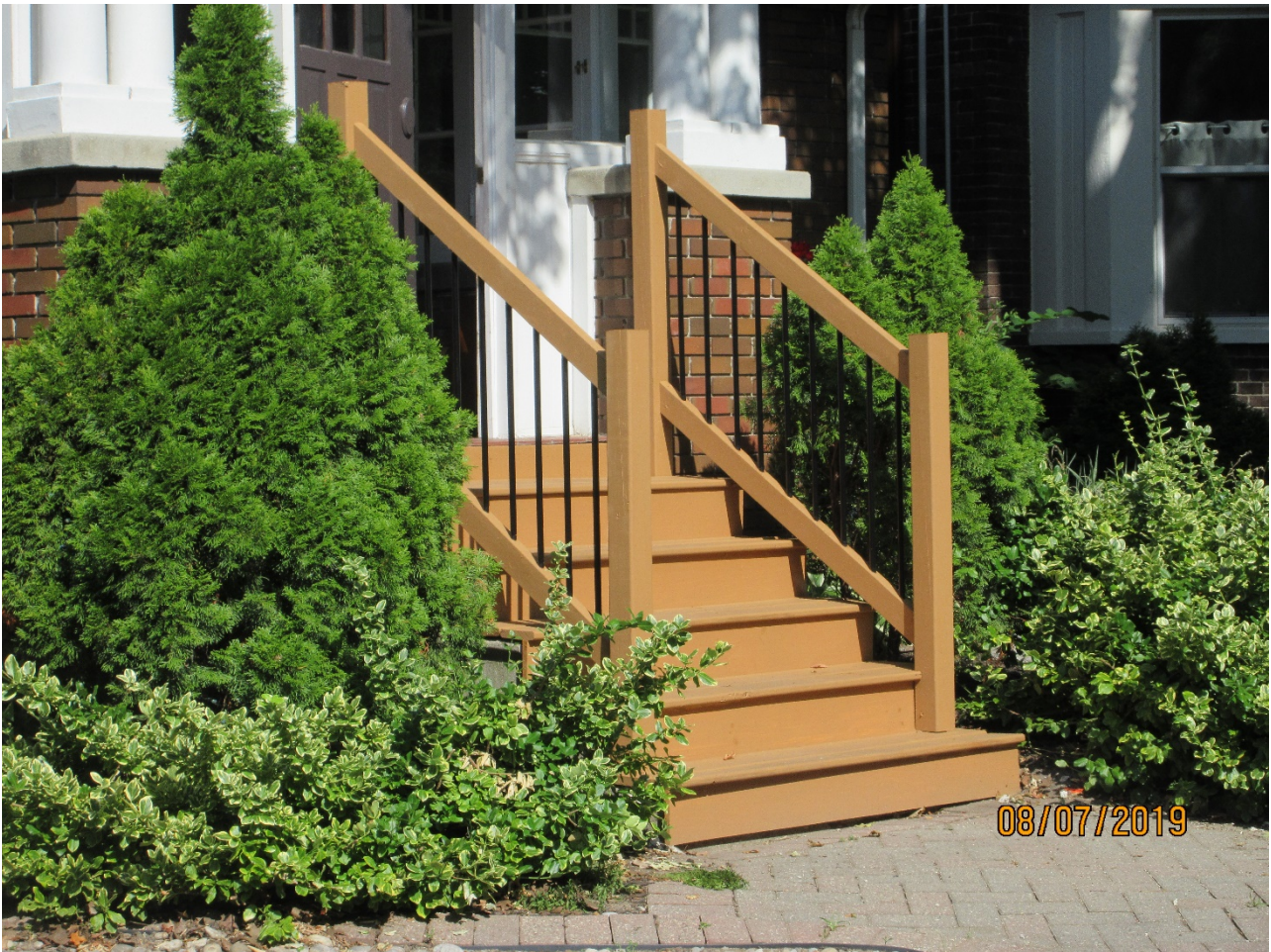
Image 3: Detail photograph of the new front steps of the property at 59 Wortley Road.
