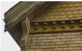
14. The brackets and modillions adhere to a single character throughout the whole structure
