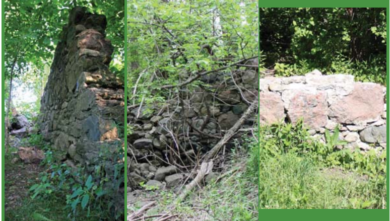
Existing Mill walls from the south, east and west
