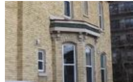
12. There is a bay window to the west side with the style of the windows echoing the characteristic style
