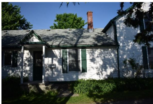
Plate 14: East façade and side entrance, looking west
