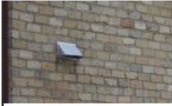
4. Clad in London buff brick masonry
