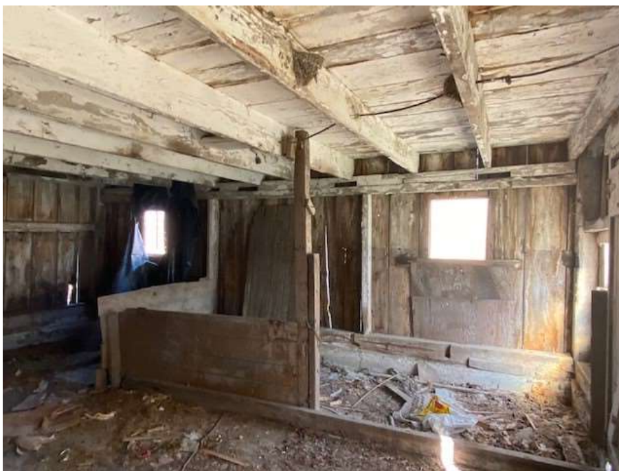
Image 6: Barn, interior view
