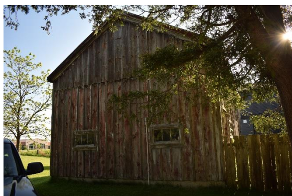
Plate 27: West façade, looking east
