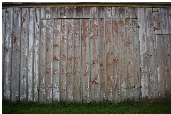
Plate 25: Doors on north façade, looking south
