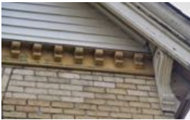
8. The gable is supported by wooden end brackets and a modillion course beneath
