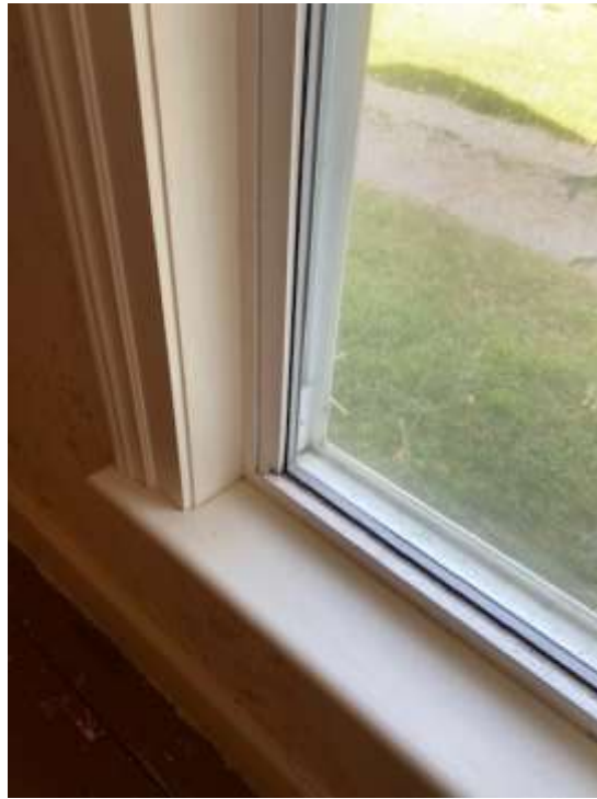
Image 12: Interior view of window replacements, casing and trim
