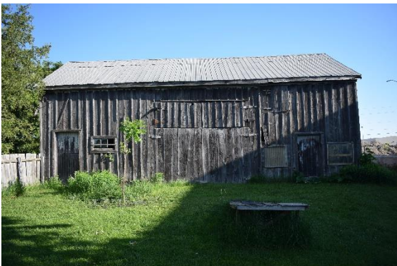
Plate 29: South façade, looking north
