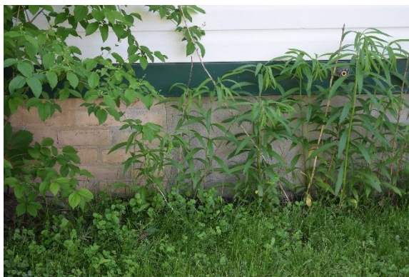
Plate 18: Foundation transition, looking east
