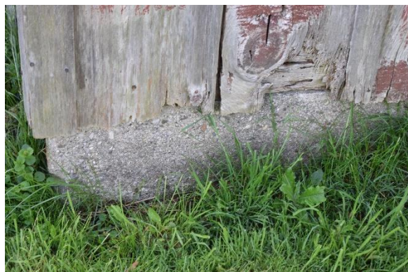
Plate 23: Concrete foundation, looking south
