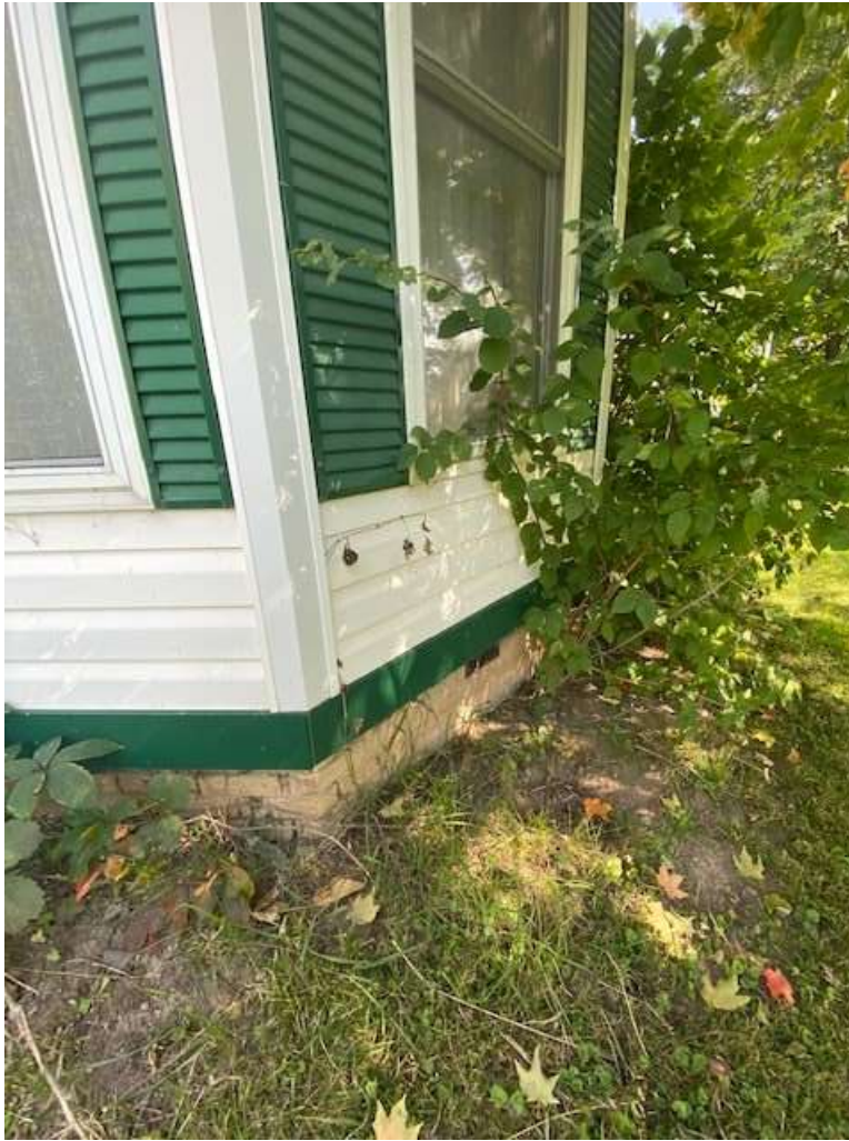
Image 10: Exterior view of bay window showing buff brick foundation
