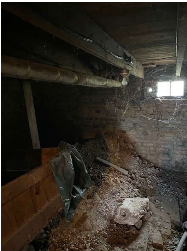
Image 16: Basement of original farmhouse
