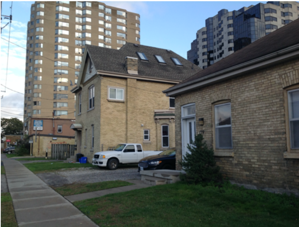
The Kent brewery (far left) and the two residences associated with it, 183 Ann Street (centre) and 179 Ann Street (right). John Hamilton owned all of these properties, and Joseph Hamilton lived in both 183 and 179 Ann Street at different times. The only other identifiable example in Canada of an extant brewery building with the brewer's house still intact next door is Alexander Keith's brewery in Halifax (see Appendix D)
