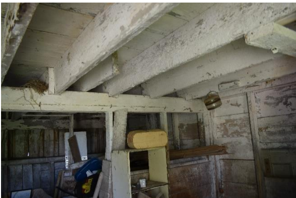
Plate 33: Joists and beams, looking north
