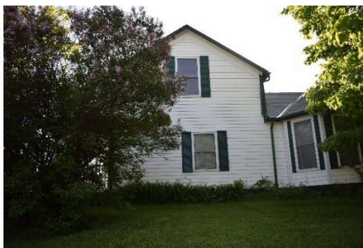
Plate 16: West façade, looking east
