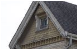
7. The gable ends exhibit wood shingling. The front façade gable is clad with siding but the east gable exhibits the original bargeboard shingling and is outlined with moulded vergeboards
