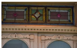
17. The doorway has a dentil-moulded architrave above
