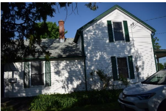
Plate 13: East façade, looking west
