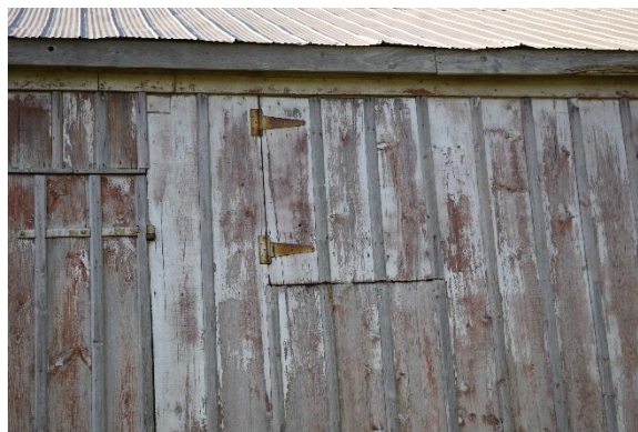
Plate 26: Hay loft door, looking south
