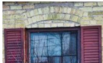
11. The single-storey wash house to the west side also exhibits a segmental-arch window with brick voussoir
