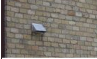
4. Clad in London buff brick masonry
