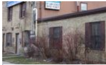
2. And to its function as a vernacular mid-19th century proto-industrial structure
