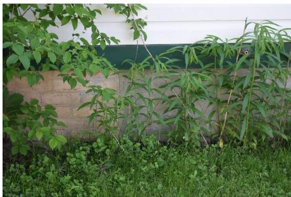
Plate 18: Foundation transition, looking east
