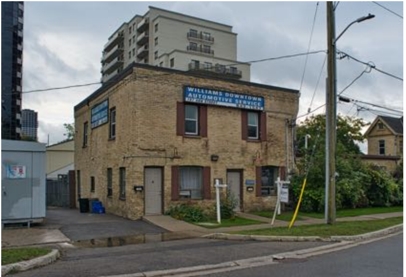
Kent Brewery building, October 2020
