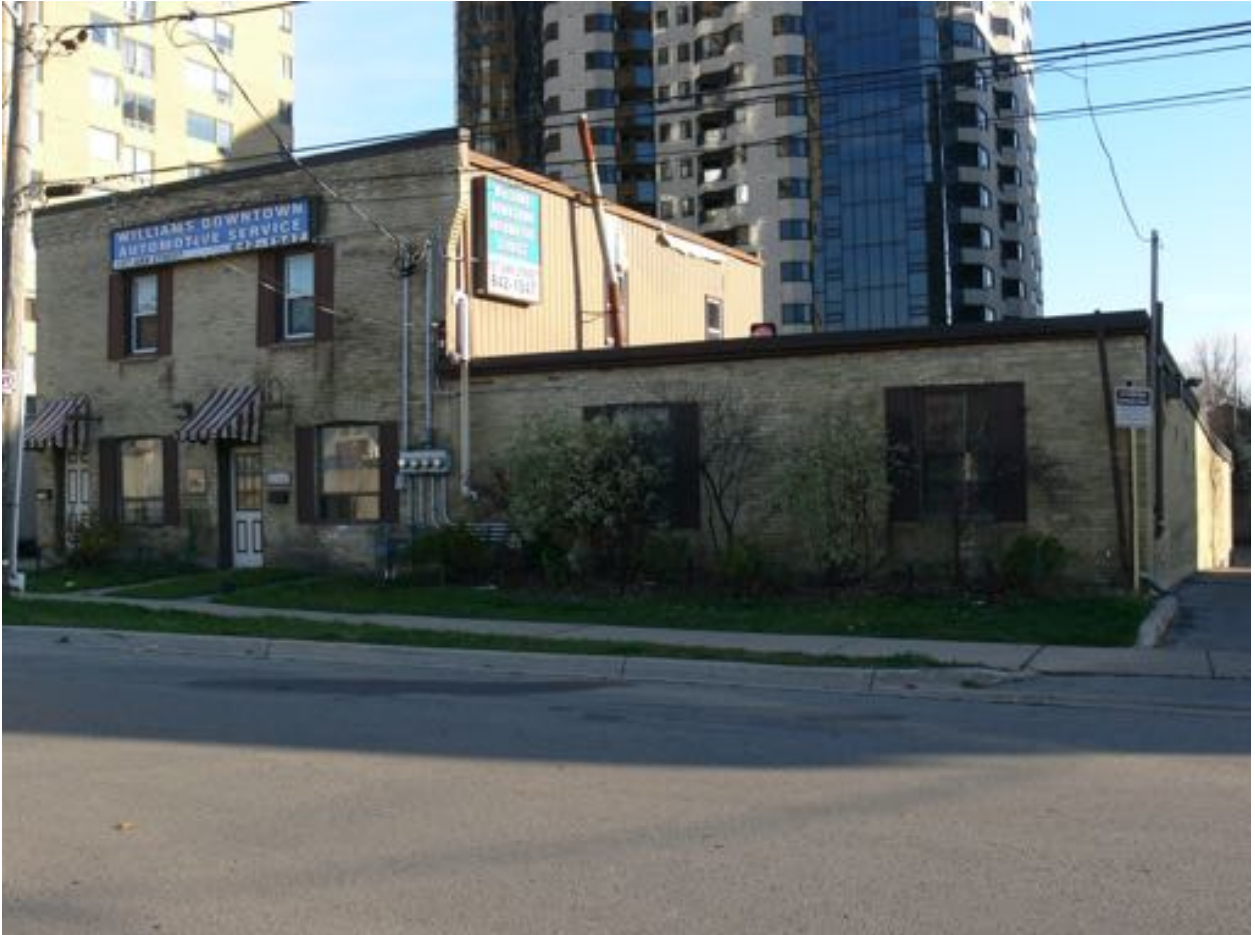
Image 5: Main brewery building (left) and brewery washhouse (right)
