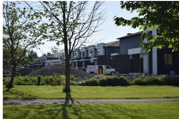
Plate 4: New construction on Gainsborough Road, looking east
