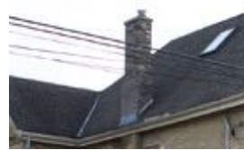
6. There are two buff brick chimneys
