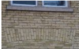
11. On the second storey of the front façade are double windows, which were apparently echoed on the first storey
