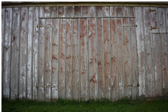
Plate 25: Doors on north façade, looking south
