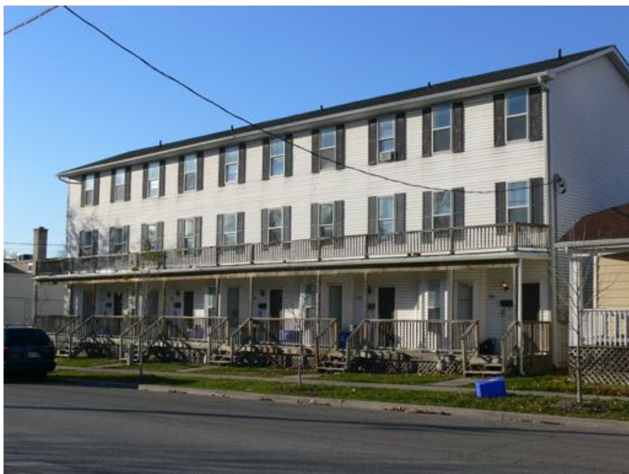
The row-houses at 146-154 Ann Street
