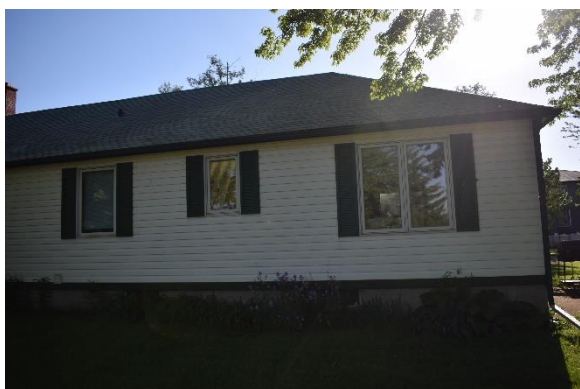
Plate 19: West façade of modern addition, looking east
