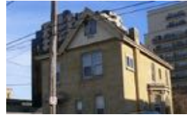
3. The house is built of buff London brick. The house has the typical irregular and stepped outline and profile of this style
