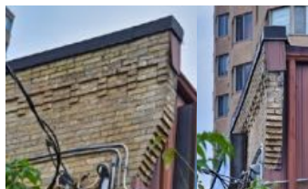
15. The brick courses end in a corbel, and form distinctive corner details
