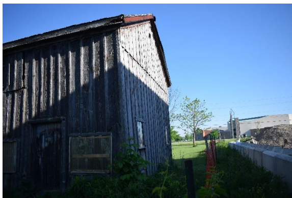
Plate 32: East façade, looking north
