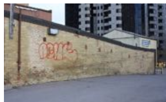
18. The washhouse, brick on a rubble stone foundation, slopes down towards the former creek-bed of Carling's Creek.
