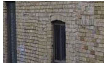
12. Door and window openings on the west and east side have been bricked over as the building's function changed
