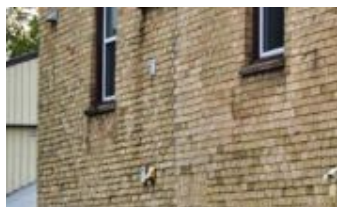
16. A line of demarcation in the brick is apparent in the middle of the east side of the building showing alterations
