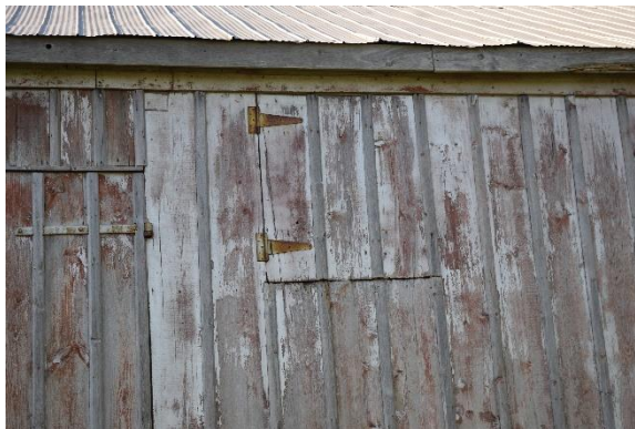
Plate 26: Hay loft door, looking south
