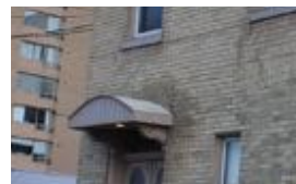
18. The porch roof of the doorway is altered but appears to adhere to the line of a previous porch and is still supported by original brackets
