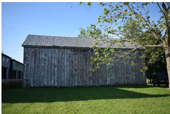
Plate 21: North façade showing side gable roof clad in metal, looking south
