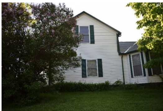
Plate 16: West façade, looking east
