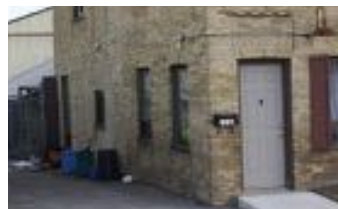
9. The extant front door is to the side of the frontage, breaking the usual symmetry of the Georgian style and pointing up its utilitarian function where floor space is needed inside for production
