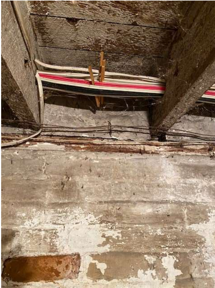
Image 15: Basement of original farmhouse showing floor joist and foundation detail
